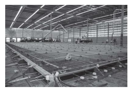
Figure 3.3 Examples of post-tensioned slabs before concrete casting. (Courtesy of VSL Australia Limited, Sydney, New South Wales, Australia.)
