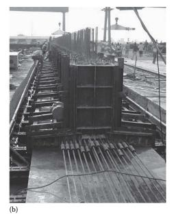
Figure 3.2 Pretensioning beds. (Courtesy of VSL International Limited, Hong Kong, China.) (a) Multi-strand pretensioning. (b) Single-strand pretensioning.
