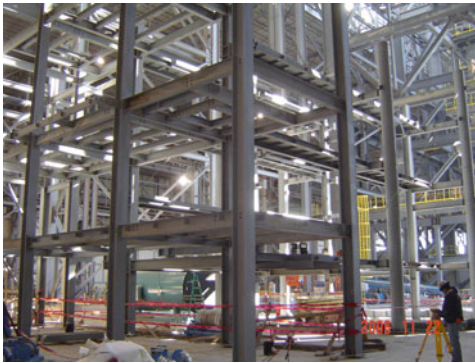
Fig. 17.12 Structural steel as first activity in the furnace area
