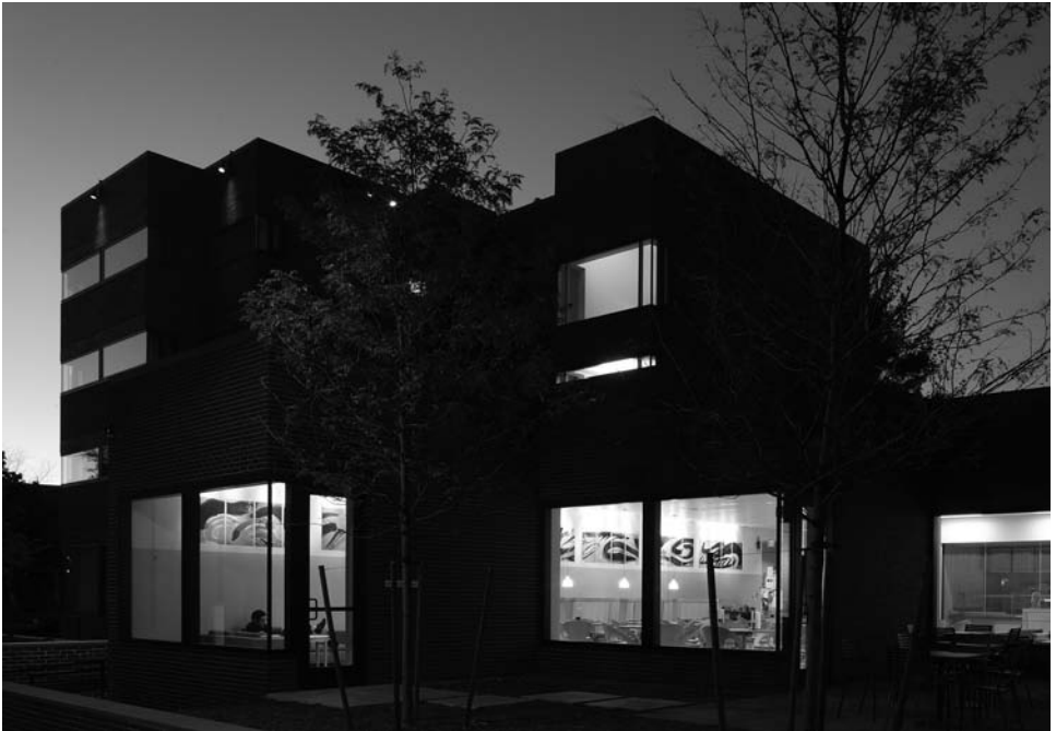
Figure 8.8 Rockefeller Hall—east façade view.
