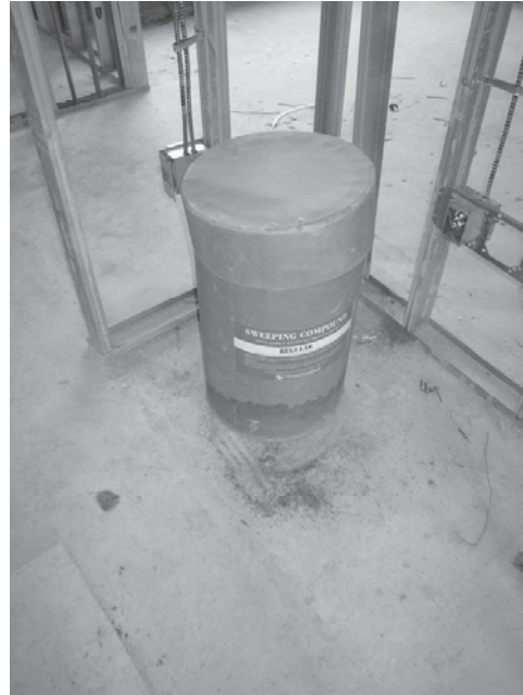
Sweeping compound used to control dust
