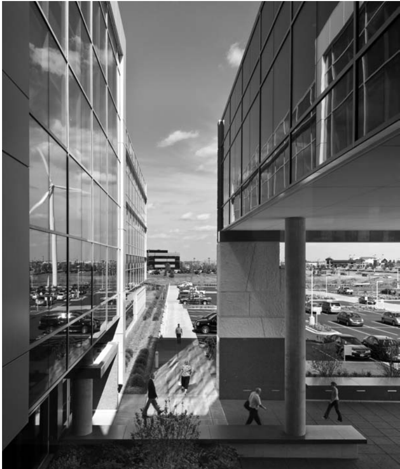
Figure 8.2 GRE headquarters—reflection of the wind turbine in the glazing of the building.
