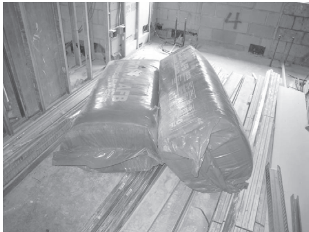
Insulation material kept sealed in plastic prior to installation
