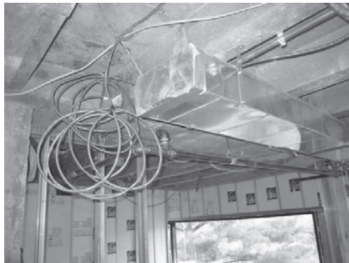
Ssealed Duct – after installation
