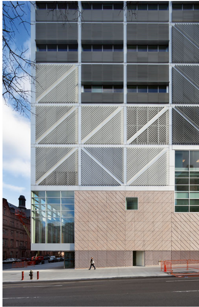
View from the courtyard Copyright Michael Moran
