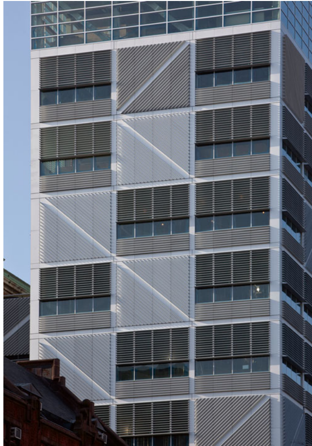
Shading system of the façade Copyright Michael Moran
