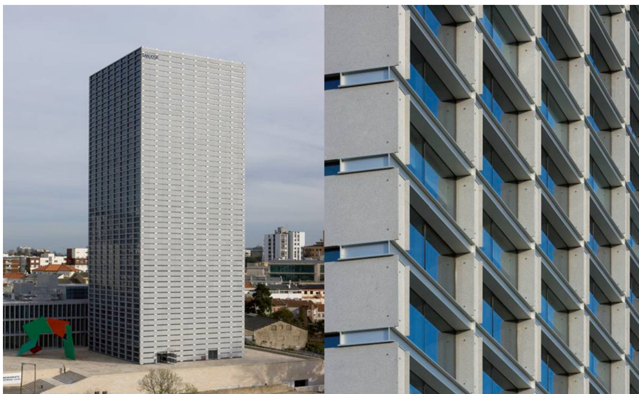
Fig. 1 General view of the building and partial view of the curtain wall
