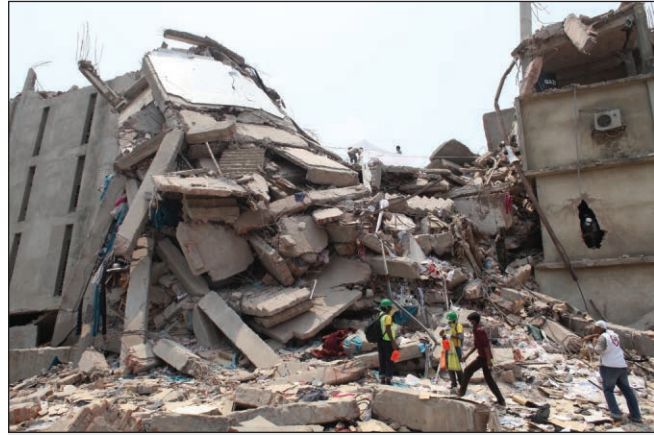
The 2013 building collapse in Rana Plaza in Bangladesh is the largest garment factory accident in history and killed 1,129 people. Although it may have been legal to ask workers to enter a building with structural damages, one could certainly question the ethics of this decision. © Zuma Press, Inc./Alamy
