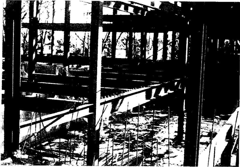
Large girder with stud shear connectors on top flange to be embedded in concrete to provide continuous lateral support (see Fig. 9.2.1b). (Photo by C. G. Salmon)
