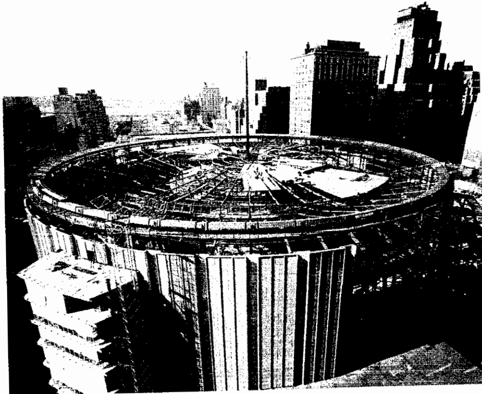
Figure 1.6.6 Cable-suspended roof for Madison Square Garden Sports and Entertainment Center, New York. (Photo courtesy Bethlehem Steel Corporation)
