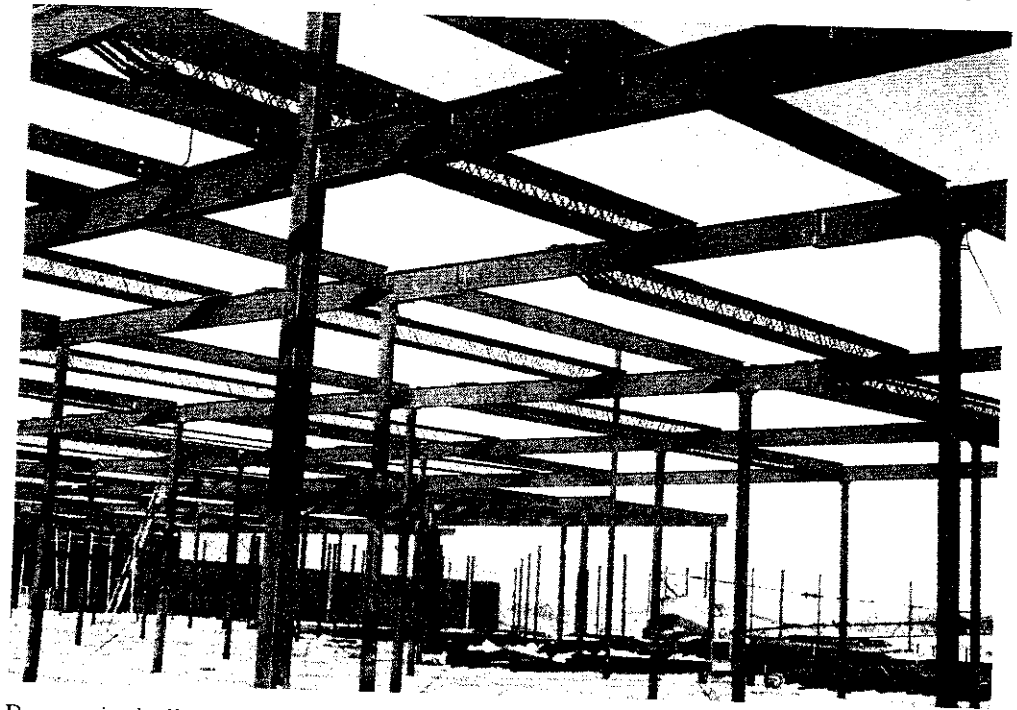
Beams, including open-web joists, channels, and W (wide-flange) shapes, along with tubular columns. (Photo by C. G. Salmon)
