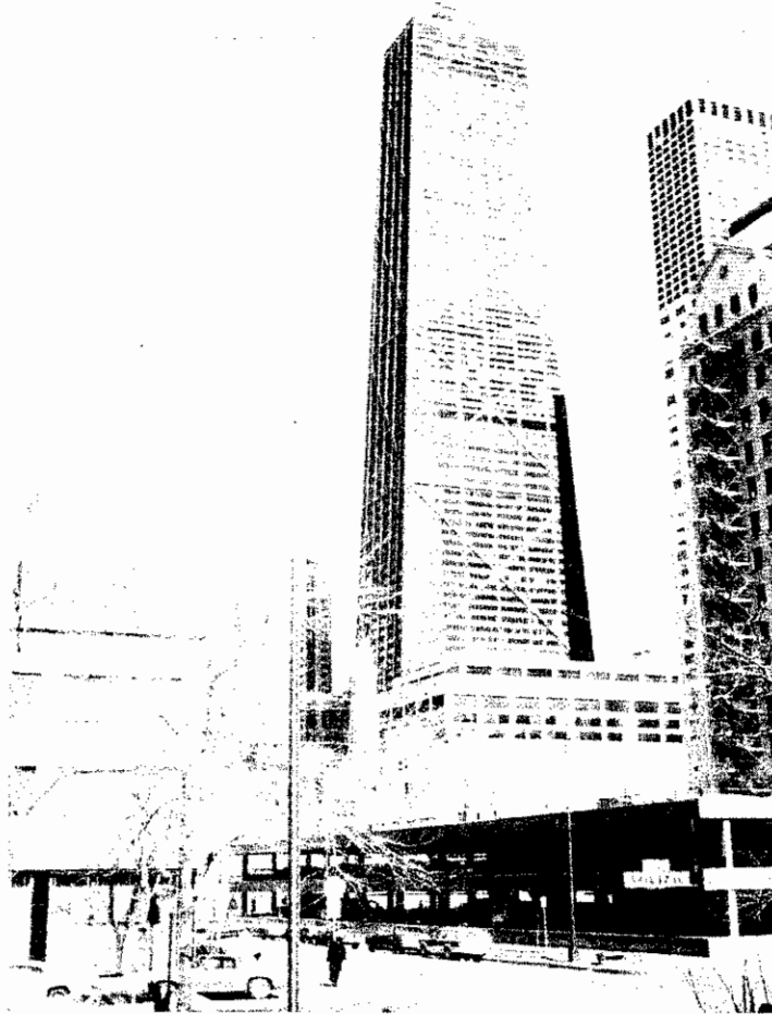
John Hancock Center, Chicago, showing exterior diagonal bracing. (Photo by C. G. Salmon)
