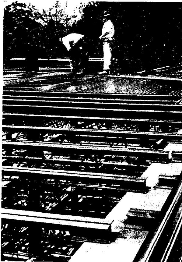
Figure 1.6.1 Floor joists (plane trusses) and steel decking. (Photo by C. G. Salmon)
