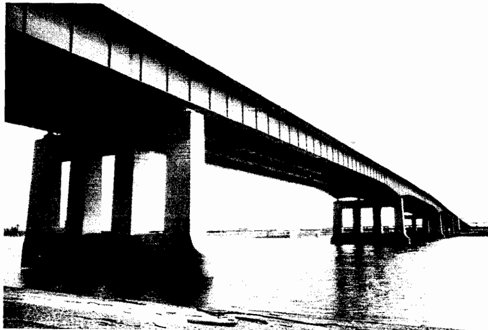
Figure 1.6.4 Continuous orthotropic plate girder across Mississippi River at St. Louis, Missouri. (Photo by C. G. Salmon)
