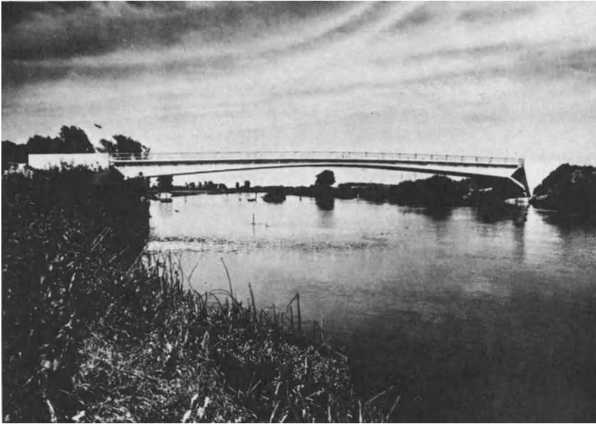
Fig. 14-17. The Esbly bridge across the Marne river in France. (Provided by and reproduced with the permission of the Freyssinet Company, Inc., Charlotte, N.C.)
