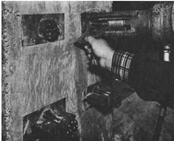
Fig. 16-5. End anchorages of tendons with cold-formed button heads. (Provided by and used with the permission of Prescon, Corp., San Antonio, Texas, a general contractor.)
