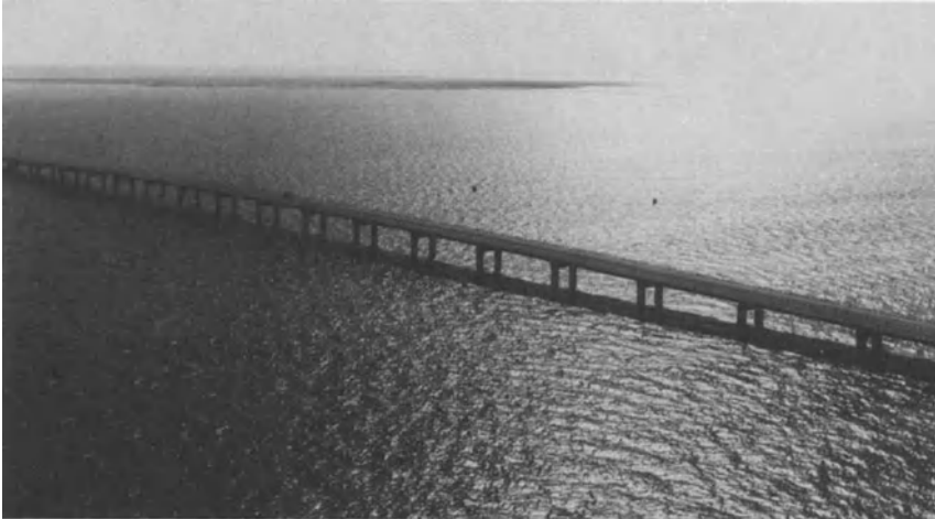
Fig. 14-19. The King Fahed Causeway connecting Saudi Arabia and Bahrain constructed of precast segments erected span-by-span. (Provided by and used with the permission of the King Fahed Causeway Authority, El Khobar, Saudi Arabia.)
