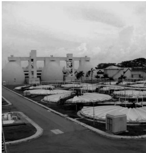
Figure 16.1 (See color insert following page 292.) Anaerobic digesters on municipal wastewater treatment plant.
