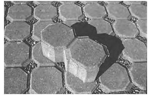
Figure 4. Interlocking pavers can allow water through openings created by the paver shape.
