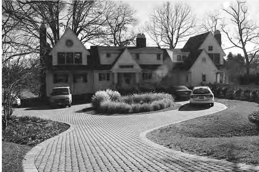
Figure 33. Owners play a key role in keeping permeable interlocking concrete pavements free from sediment, weeds, and spills. This installation filters runoff prior to entering the Chesapeake Bay in Maryland.
