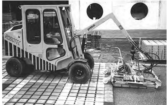
Figure 31. Mechanized placement of pavers with wide joints.
