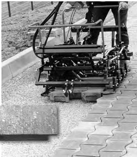
Figure 7. Units with indented sides store additional runoff.
