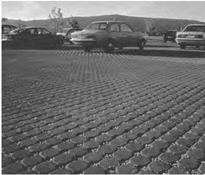
Figure 2. Permeable interlocking concrete pavement combines stormwater infiltration, retention and parking into one place, thereby conserving land.
