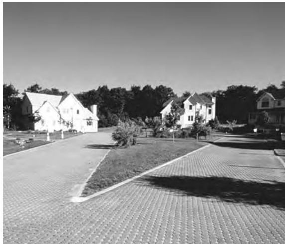
Figure 28. Besides expected decreases in stormwater, runoff monitored from permeable interlocking concrete pavement projects such as Glen Brook Green Subdivision, Waterford, Connecticut in the Jordan Cove Watershed demonstrate substantial reductions of pollutants compared to those from conventional pavements.
