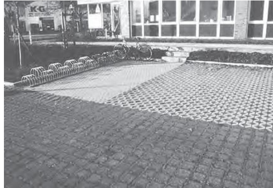
Figure 9. Solid, grid, and permeable interlocking concrete pavers working in harmony to reduce water runoff and pollution, and to provide a more comfortable microclimate.
