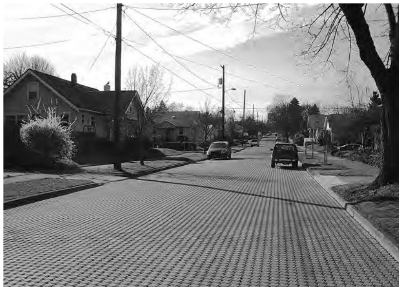
Figure 11. Portland, Oregon renovated streets with about 20,000 sf (2,000 m 2 ) of permeable interlocking concrete pavement after water and sewer line repairs in an older neighborhood. The city incorporated modeling to evaluate this pavement. The pavement decreased combined sewer overflows to the waste treatment plant and discharges into the Willamette River.
