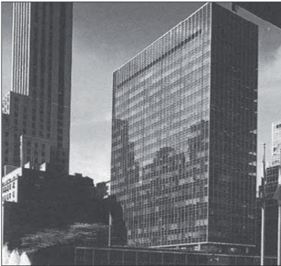
5.9a Early use of green heat-absorbing glass at the Lever House building, New York (1951–52)
