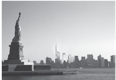
4.5 Proposal for the replacement for the World Trade Center towers, New York (Daniel Libeskind)
