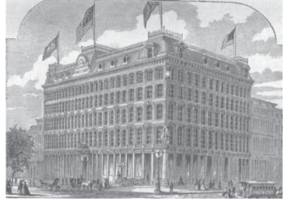
4.7 Public Ledger newspaper building, Philadelphia PA (1867)
