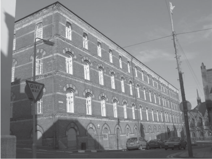
4.10 Welch Margetson factory, Horace Street, Derry (1872)
