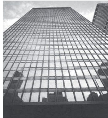
5.9b Early use of pink-grey glass at the Seagram building, New York (1954–58)
