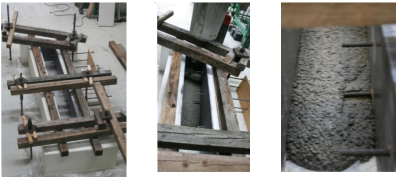
Figure 2. Pictures of the formwork (left), during casting of SCC (middle), and a close up of the SCC flow near the reinforcement (right).
