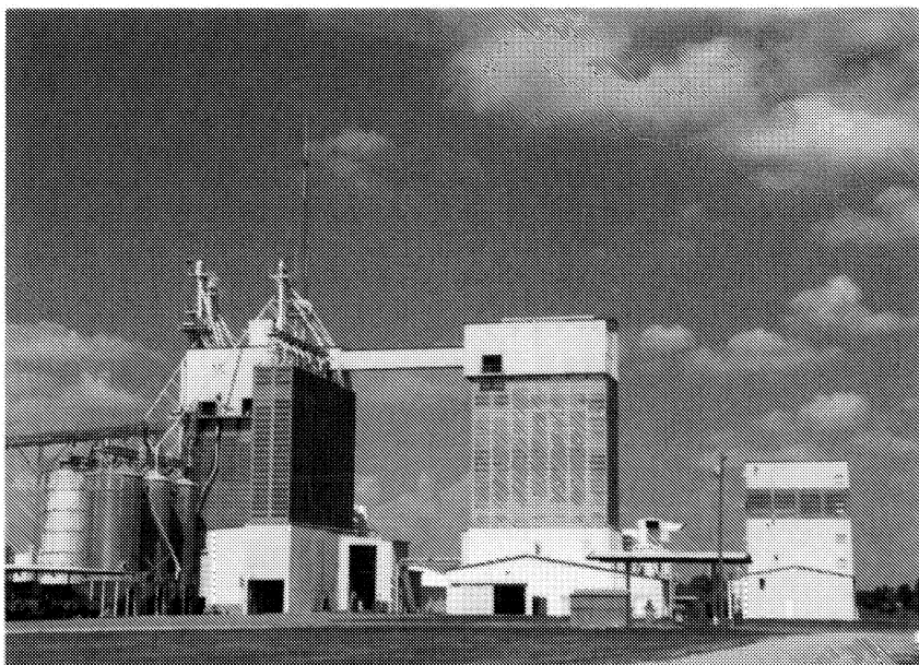
Figure 8.1 Catfish feed mill located in Mississippi Delta. It can produce up to 1500 metric tons of extruded (floating) feed daily. The feed is hauled in bulk directly to catfish farms nearby. Most catfish feed mills are owned by catfish farmers.
