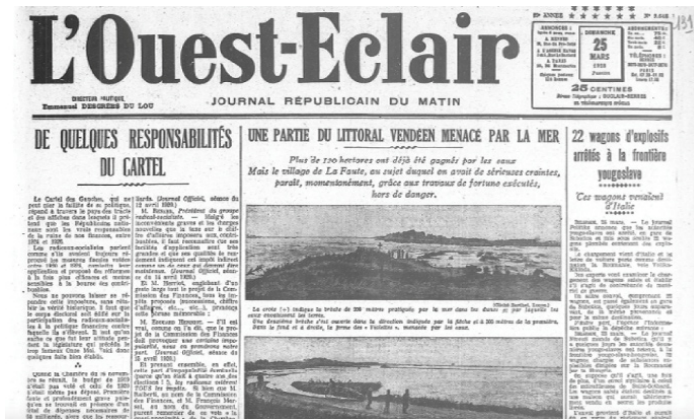
Figure 3.10. Press article of March 25th, 1928 showing the damage caused by an immersion on the current territory of La Faute-sur-Mer. At that time, the sea invades only agricultural lands because of a weak urbanization
