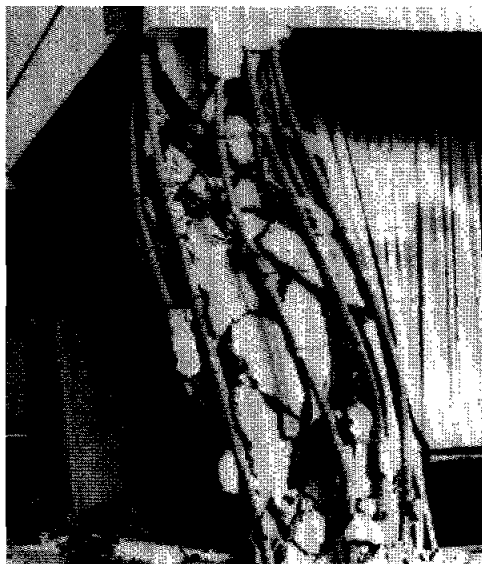
Figure 19.2.7 Brittle failure of a tied corner column of the Olive View Hospital building. (From K. V. Steinbrugge Collection, courtesy of the Earthquake Engineering Research Center, University of California at Berkeley.)
