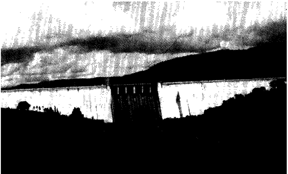
Figure 17.11.3 Koyna Dam, a 338-ft. high and 2,800-ft. long concrete gravity dam near Poona, India. This major dam was damaged by the Koyna earthquake of December 11, 1967, a Magnitude 6.5 event centered 3 miles from the dam. [From A. K. Chopra, "Earthquake Response Analysis of Concrete Dams," in Advanced Dam Engineering for Design, Construction and Rehabilitation (ed. R. B. Jansen), Van Nostrand Reinhold, New York, 1988.]
