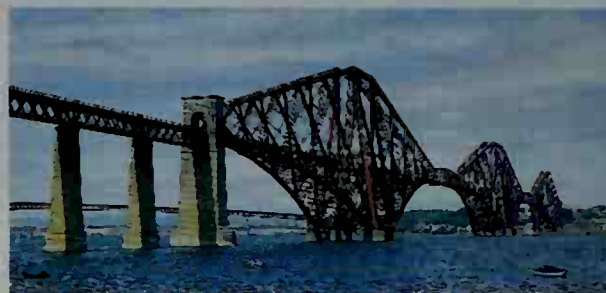
Figure 6.17 The Forth Bridge (Scotland, 1890) is an example of a large truss bridge. Each main span is 520 m long.
