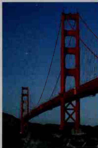
Figure 6.19 The Golden Gate Bridge (California) has a central suspended span 1280 m (4200 ft) in length.
