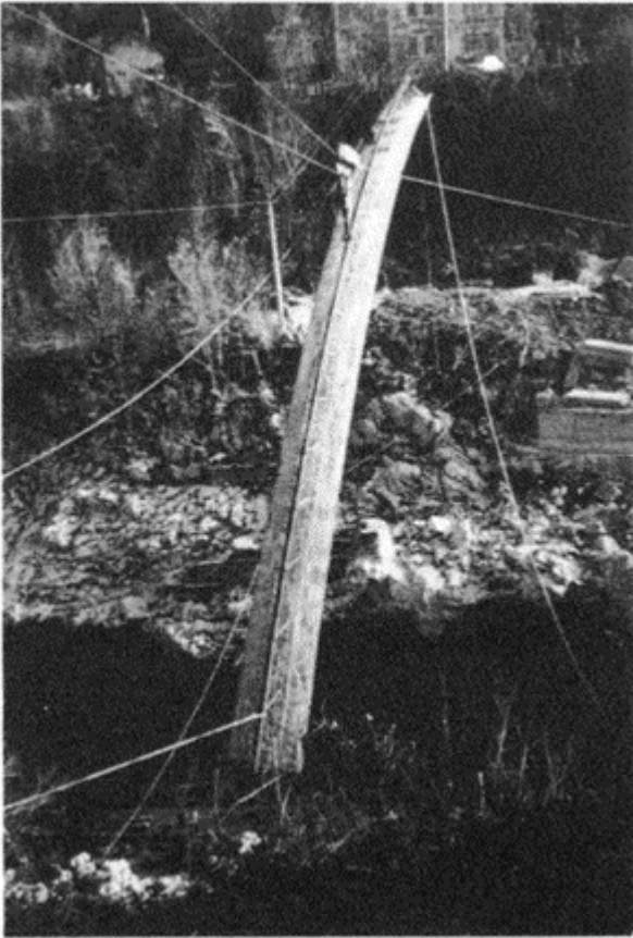
Figure 5 Placement of the first element on site
