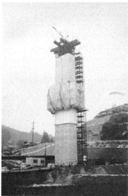
Photo 5 Installation of Slipform zv568
