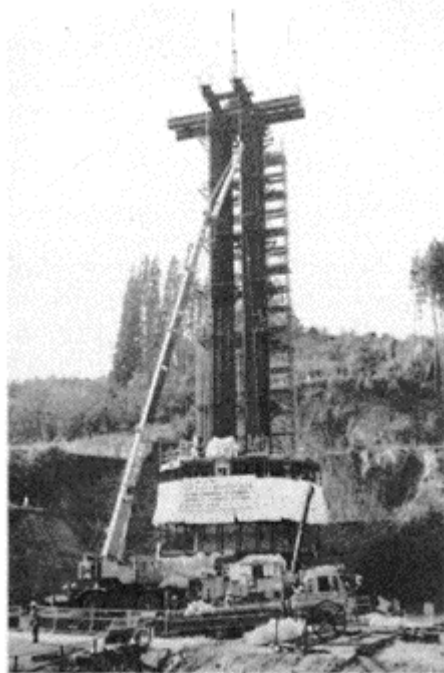
Photo 4 PC Strand Automated Feeder
