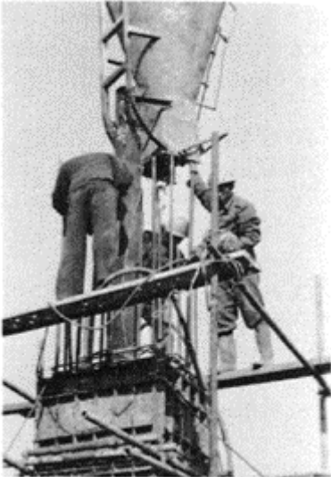
Figure 6 Pouring C80 concrete column with steel pipe core
