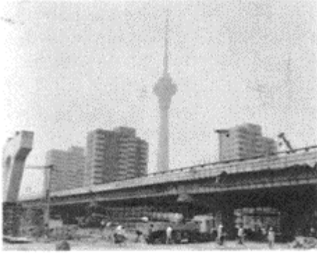
Figure 8 Concrete beams for the bridges
