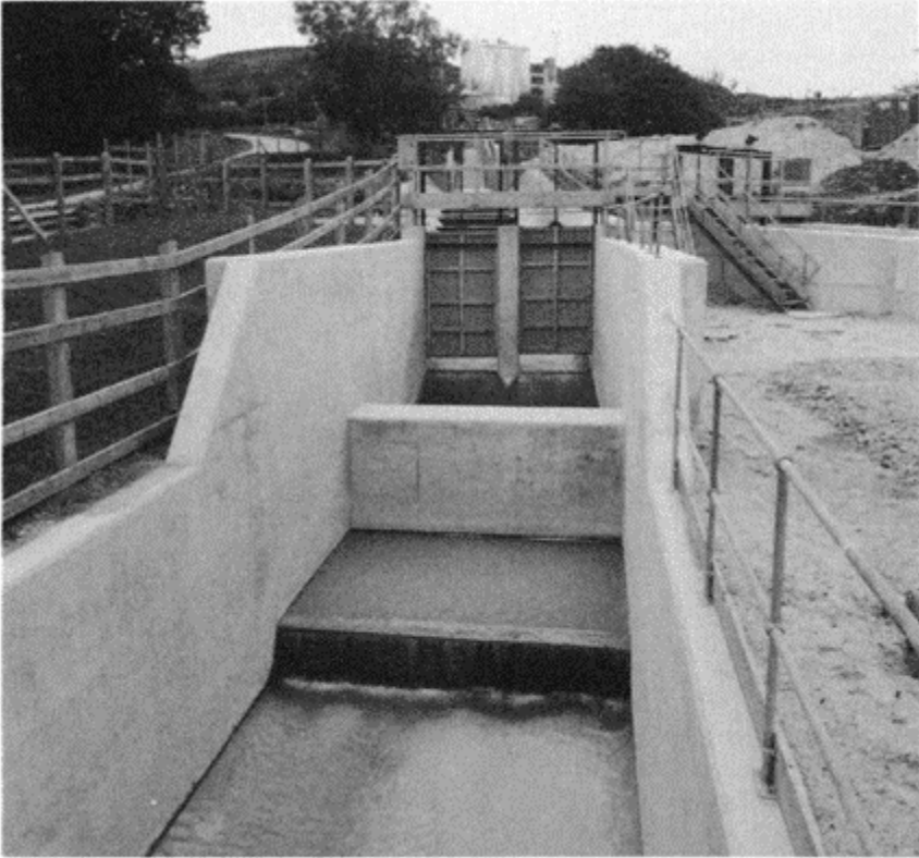
Figure 2 Culvert constructed in project 3
