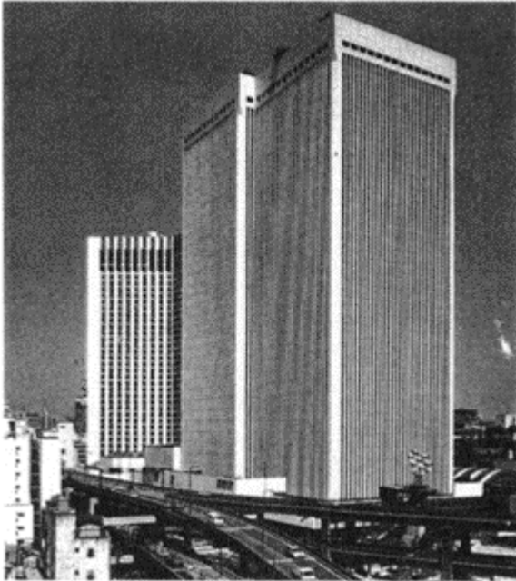
Figure 14 Applications of FRC: Fiber reinforced wall panels [Ark Mori Building, photograph courtesy of Kajima Corporation, Tokyo, Japan]
