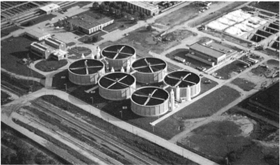
Figure 1—Trickling Filter Towers at end of construction.
