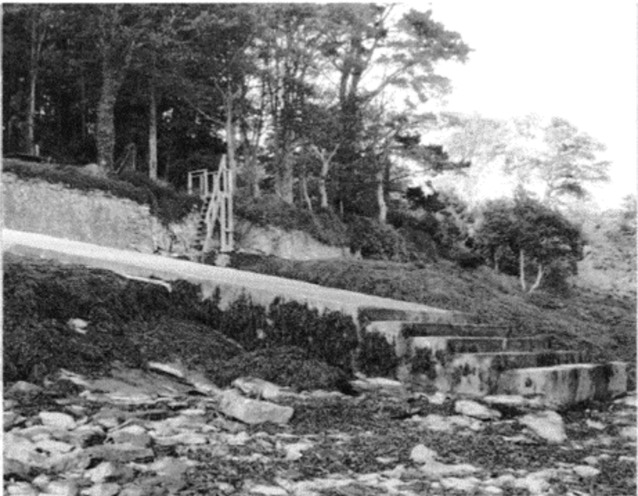
Figure 1 Marine slipway constructed in project 2
