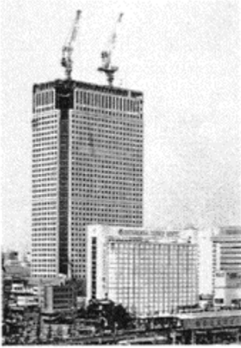
Figure 24 New Shinagawa Prince Hotel (39-story, CFT-structure) [34]
