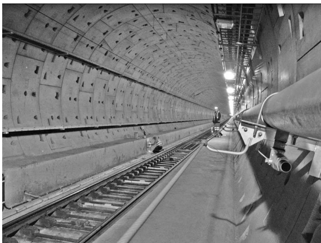
Figure E.2. Installing monitoring in CTRL tunnel during maintenance period
