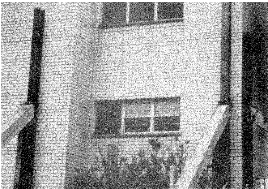
FIGURE 8.67 Shoring to abate settlement (see Figure 8.66).
