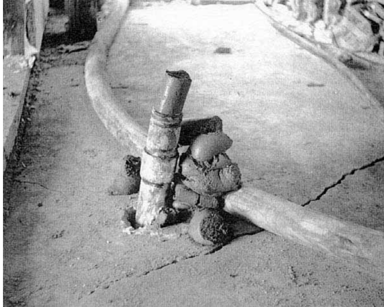
FIGURE 6B.58 Very stiff, mortar-like consistency grout.
