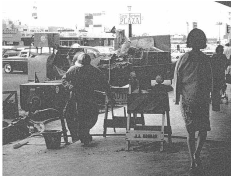
FIGURE 6B.70 Grouting faulty backfill in shopping center.
