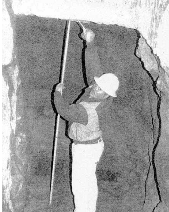
FIGURE 6B.103 Nine foot vertical cut under foundation in cohesionless beach sand.
