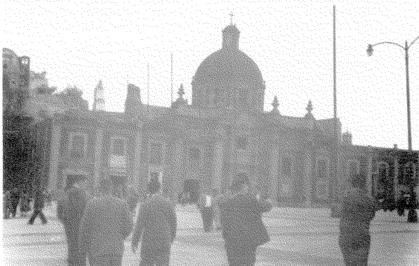
FIGURE 8.34 Foundation failure of Guadalupe shrine.
