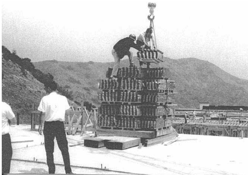
FIGURE 6B.61 Load test in progress.
