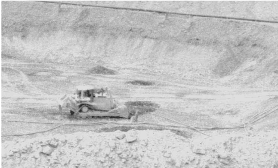
FIGURE 6A.152 Leveling backfilled crater.
