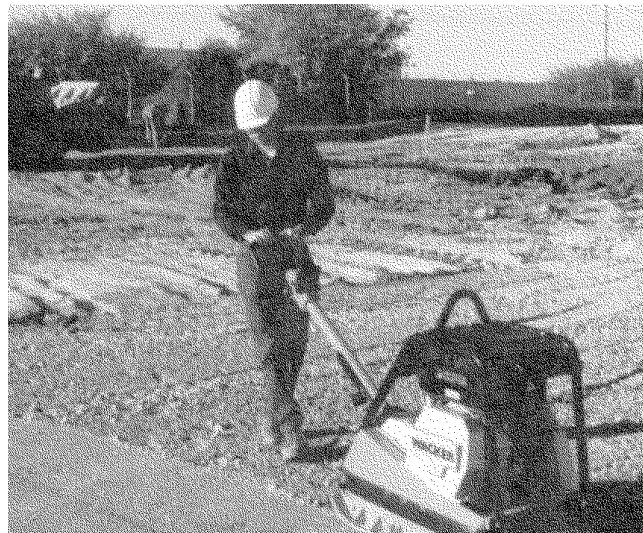
FIGURE 6A.30 Vibratory plate compactor (courtesy of Wacker Corporation, Menomonee Falls, WI).
