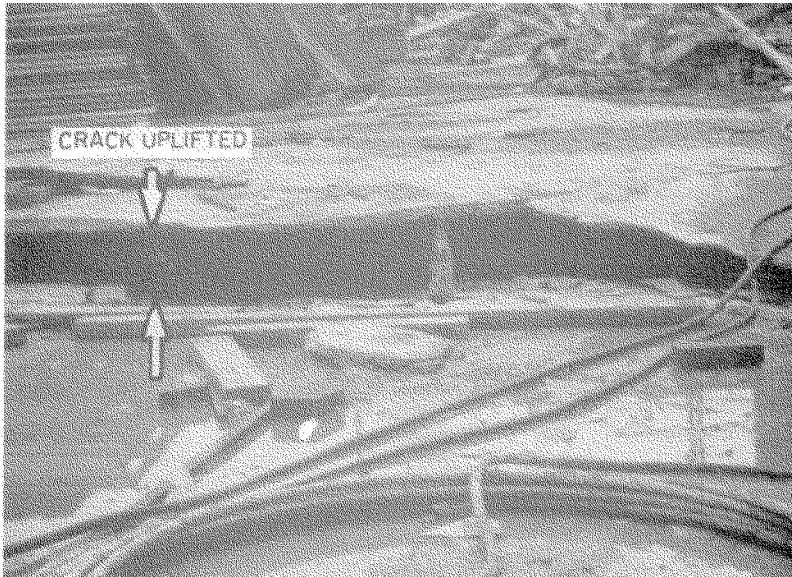
FIGURE 8.50 Prestress loads cause slab uplift.
