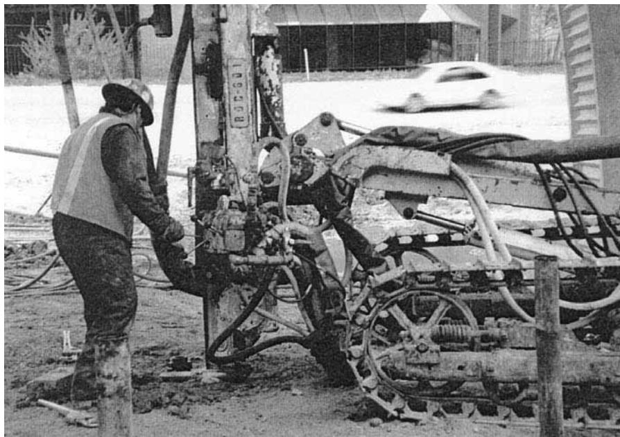
FIGURE 6B.75 Small track-mounted rig used for drilling grout holes.
