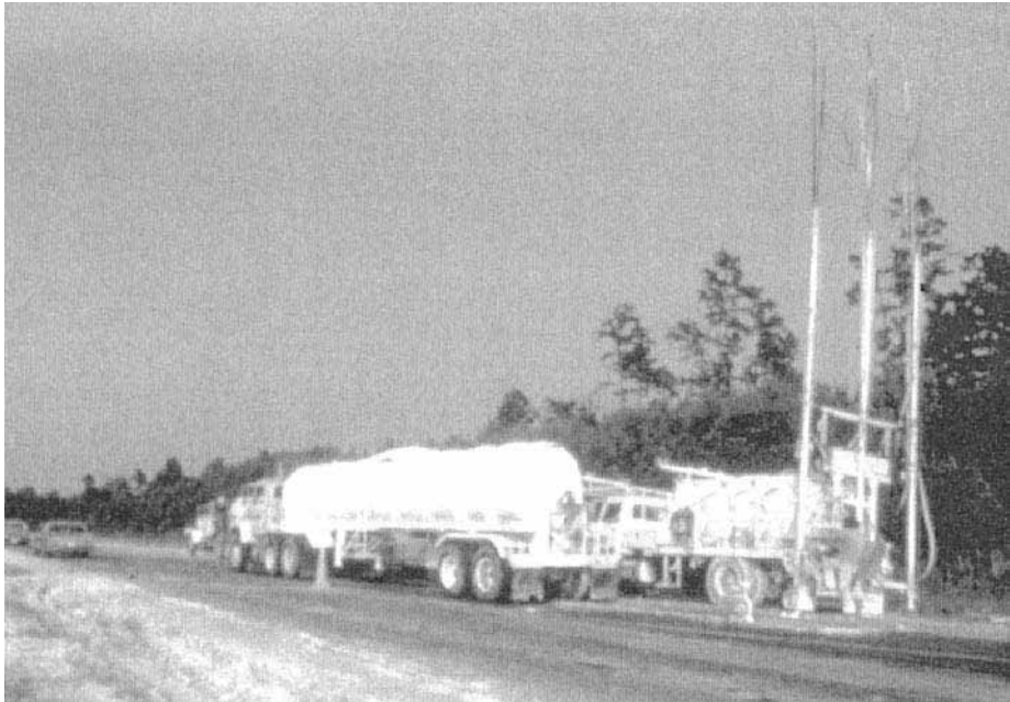
FIGURE 6B.34 Large-scale lime injection.
