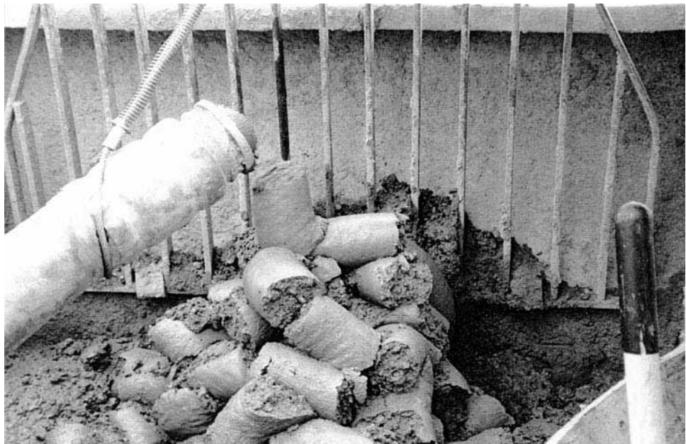
FIGURE 6B.7 Stiff mortar-like grout extruding from grout hose.
