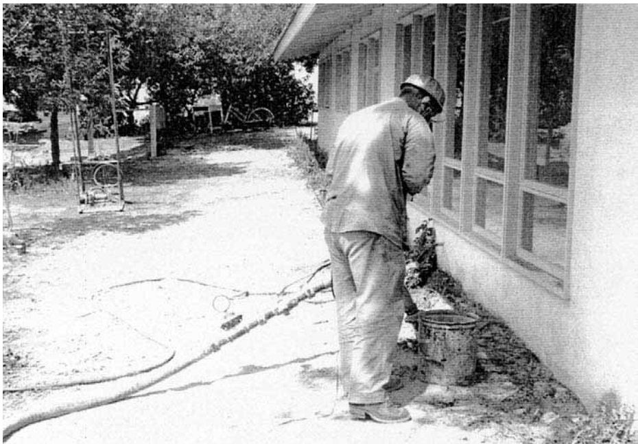
FIGURE 6B.2 Compaction grouting under a structure to correct settlement damage.
