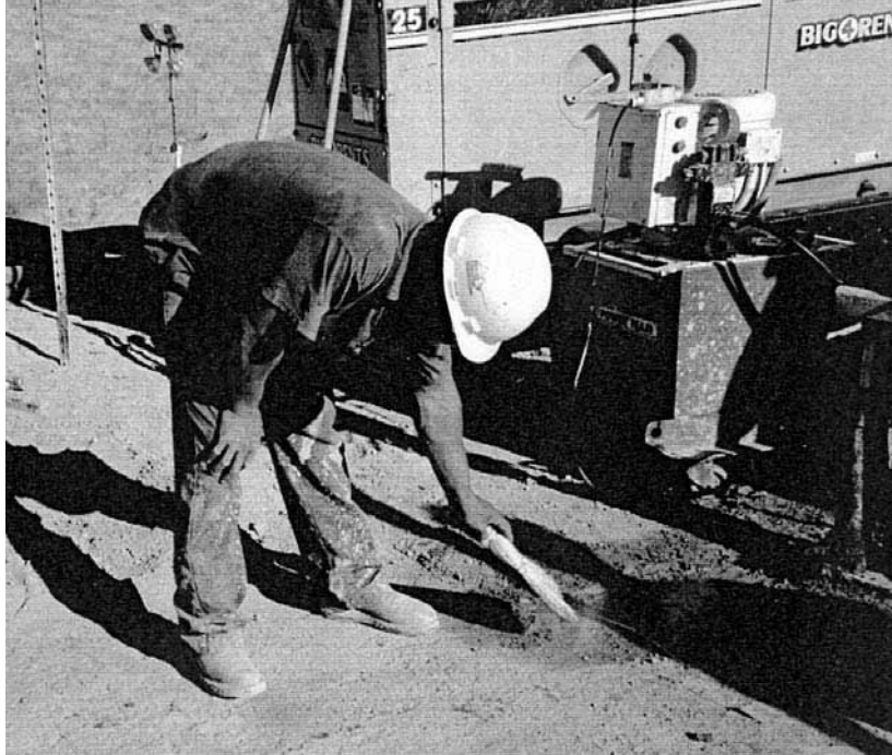
FIGURE 6B.163 Sweeping loose material off of earth surface to enable closer visual inspection of surface.
