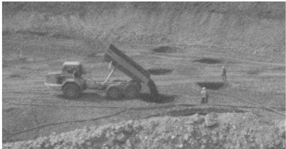
FIGURE 6A.151 Dumping backfill into crater.
