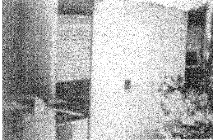
FIGURE 7B.7.4. ( continued ). Apartment building repair. (c) Steel beams are replaced with smaller plates once the wall has been plumbed. The excess bar is cut off flush with the nut and the assembly is stuccoed over and painted
