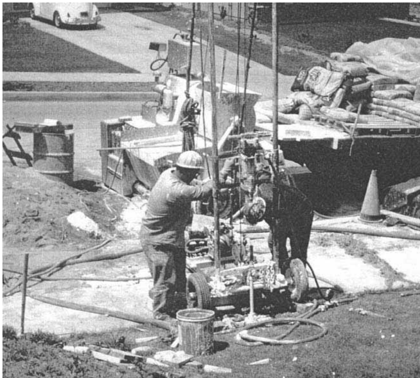
FIGURE 6B.33 Small-scale lime injection
