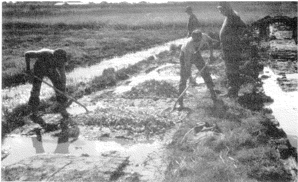
FIGURE 6A.208 Modification of highly plastic clay with lime in Vietnam in 1967, illustrating the reduction in plasticity and agglomeration of particles into clods (courtesy of Dr. Nathaniel S. Fox, Geopier Foundation Company, Scottsdale, Arizona).
