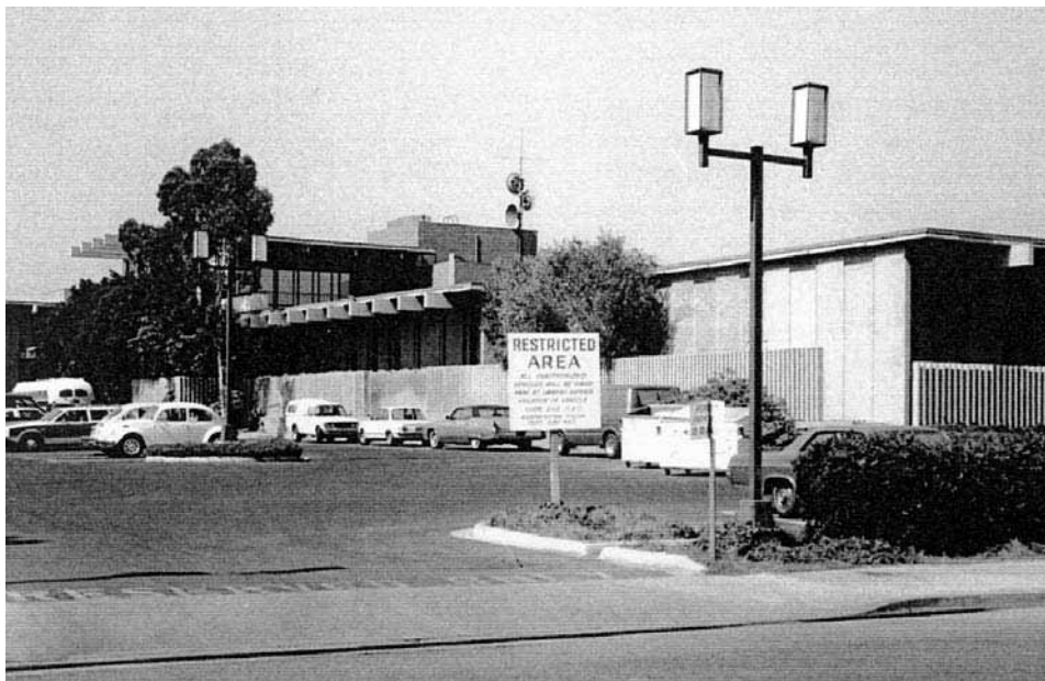
FIGURE 6B.62 West Orange County Municipal Courts building underlain by faulty soil.
