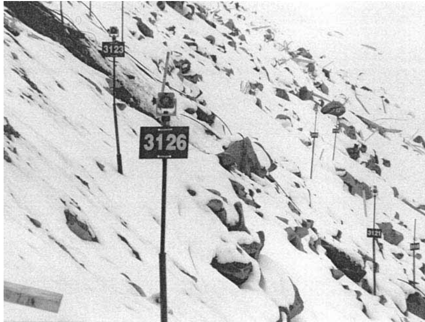
FIGURE 6B.159 Part of a large array of survey prisms covering the face of a dam during grouting.
