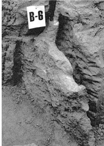
FIGURE 6B.42 Two wing grout mass resulting in hydraulic fracturing of the soil.
