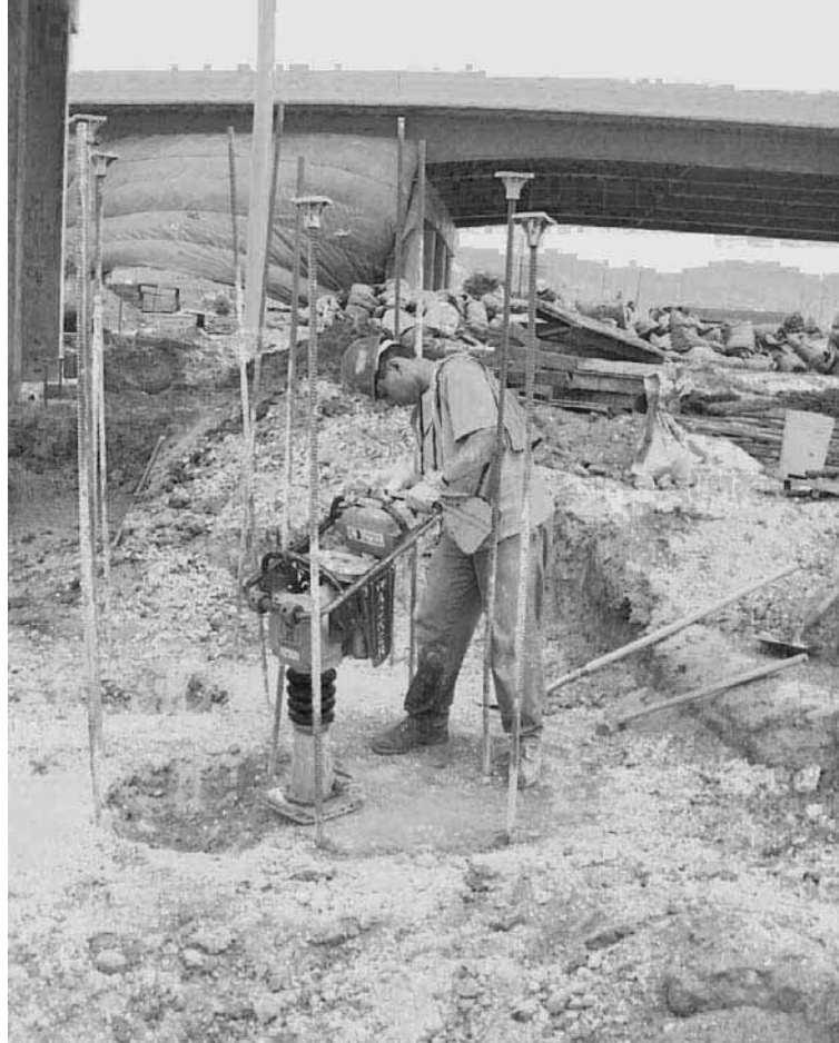
FIGURE 6A.32 High-frequency rammer.
