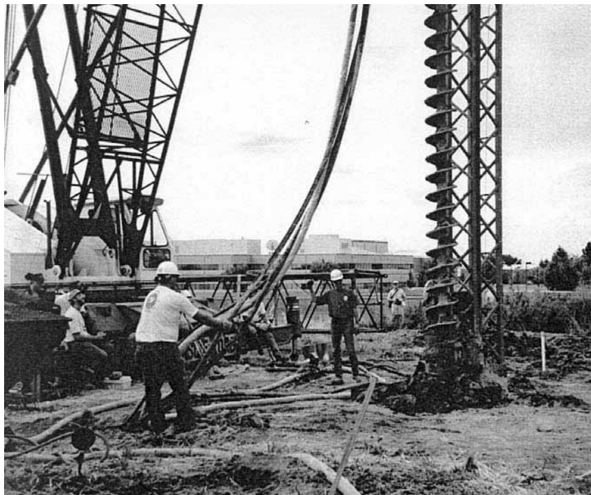
FIGURE 6B.132 Casting of an auger-cast pile.
