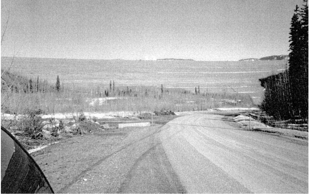
FIGURE 6B.79 Bennett dam in British Columbia, Canada, one of the worlds largest earth embankment dams.
