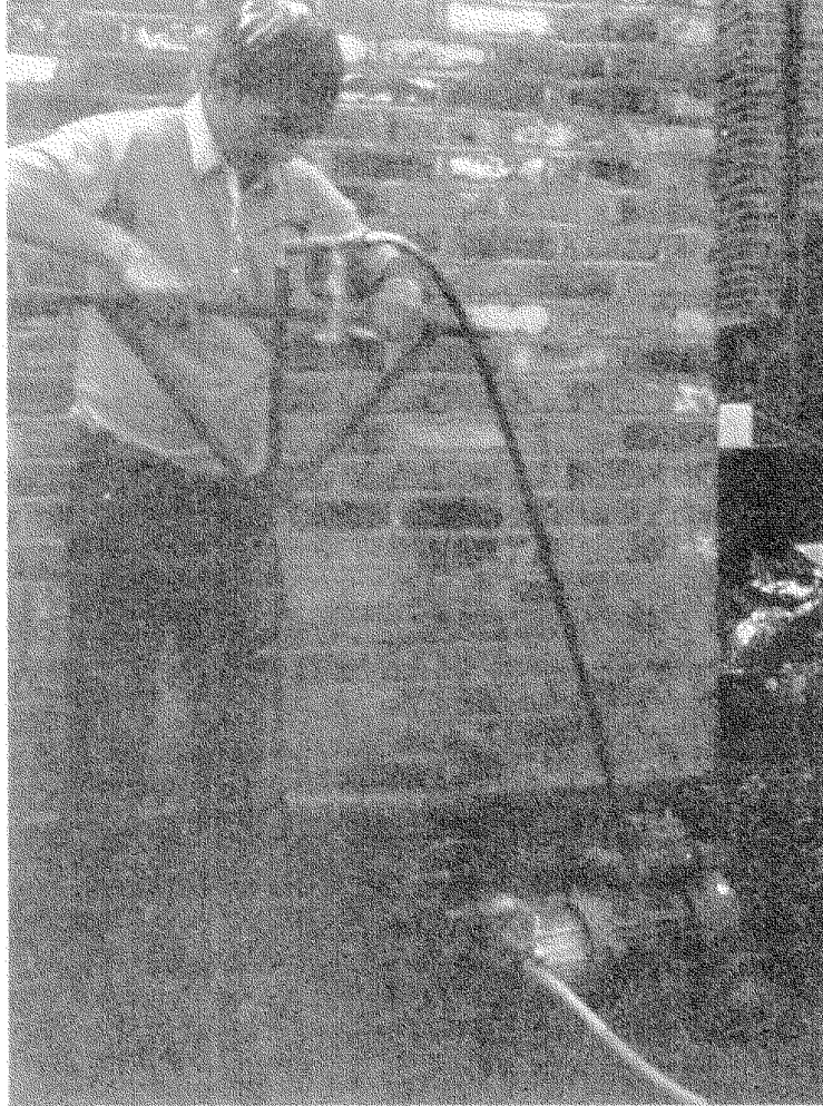
FIGURE 7B.6.5. Chemical injection through a specially designed stem.
