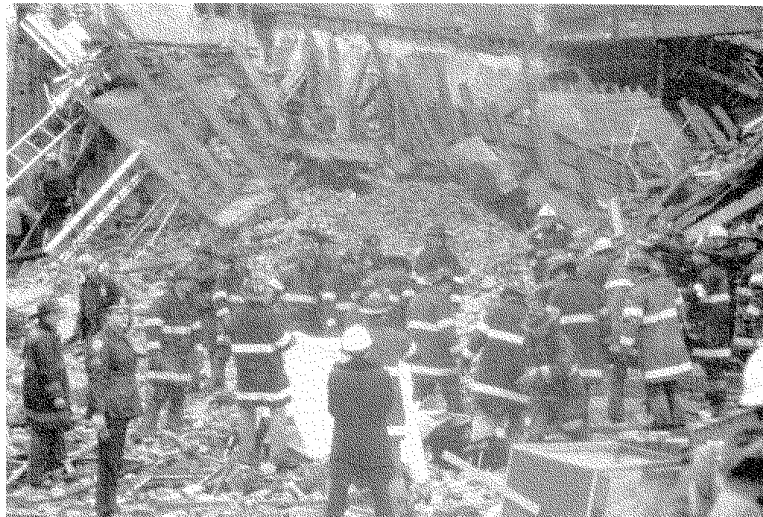
FIGURE 8.55 Collapse of structure.
