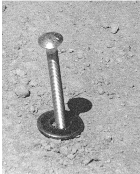
FIGURE 6B.171 Long bolt used to mark location of grout hole.
