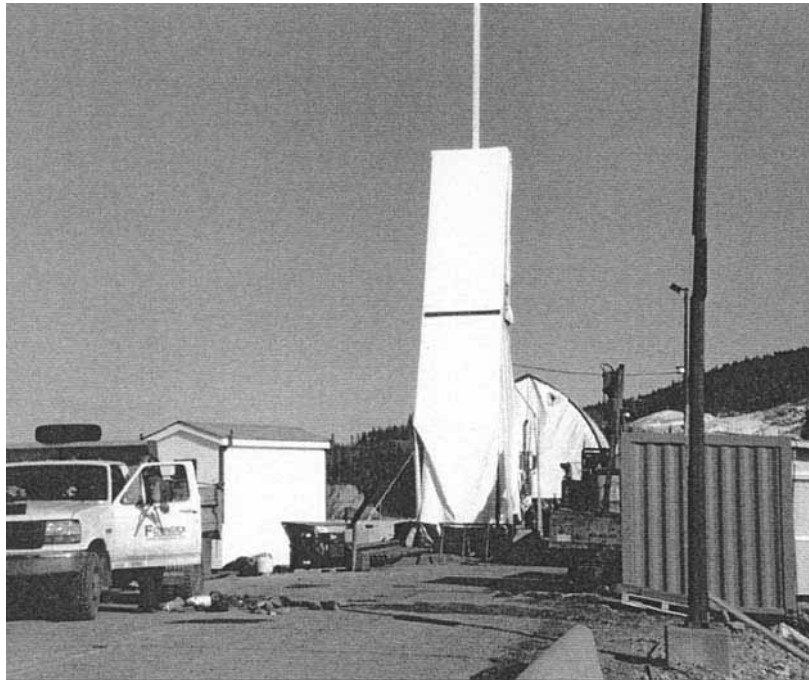
FIGURE 6B.81 Cold weather enclosures.
