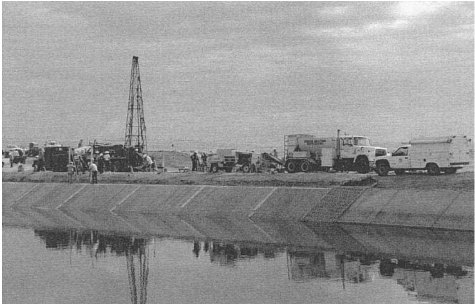
FIGURE 6B.84 Mile 55 of the California Aqueduct during the emergency grouting repairs.
