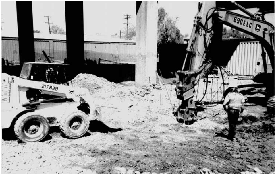
FIGURE 6A.171 Installation of a geopier with an excavator supplying the energy.
