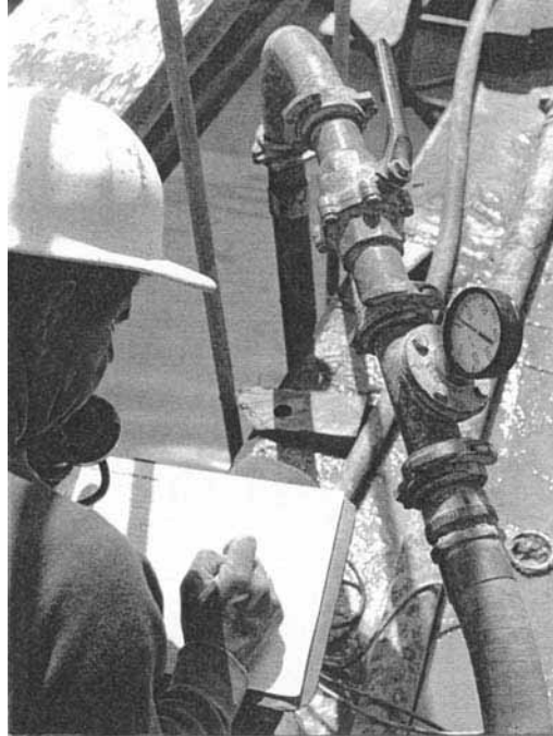
FIGURE 6B.69 Grout injection header.
