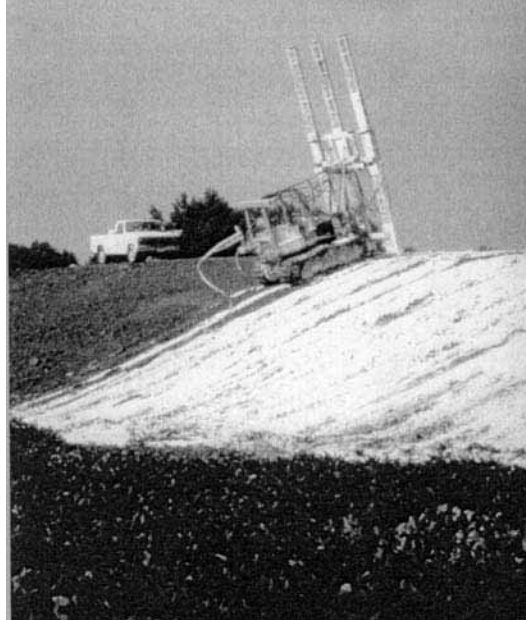
FIGURE 6B.5 Injection of lime slurry into a clay soil.
