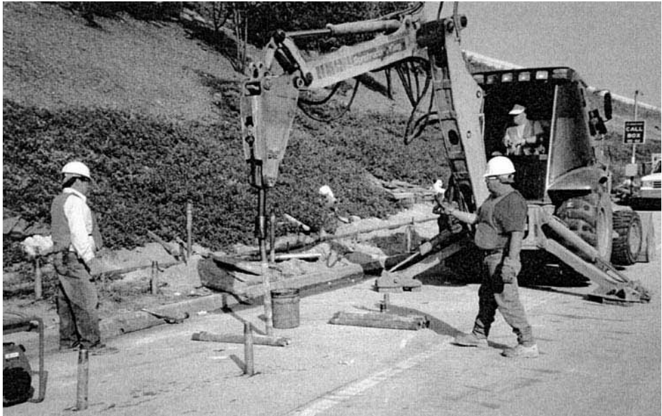
FIGURE 6B.74 Driving grout injection casing.
