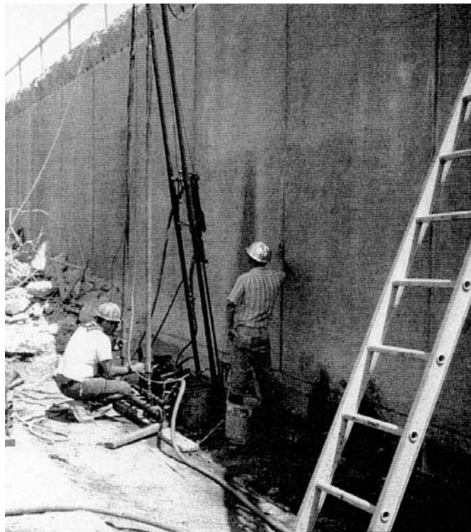
FIGURE 6B.96 Grout injection from the top down with special drive needles.
