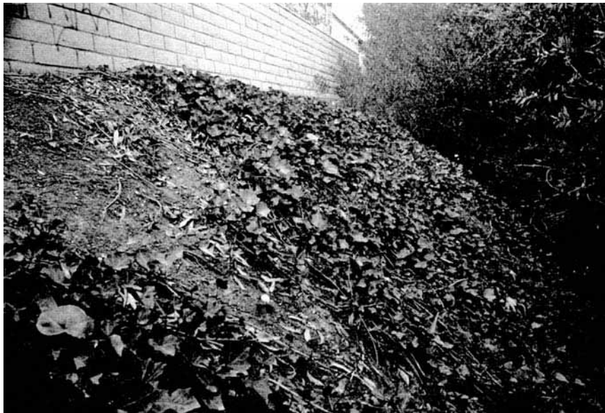
FIGURE 6B.50 Displaced slope caused by excessive pumping rate and clay in the grout.
