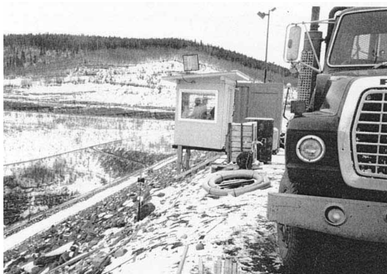
FIGURE 6B.160 Prisms were constantly scanned from a survey total station inside protective shelter.
