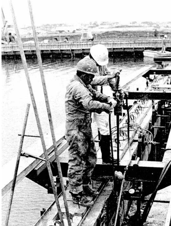
FIGURE 6B.68 Drilling of underwater grout holes.
