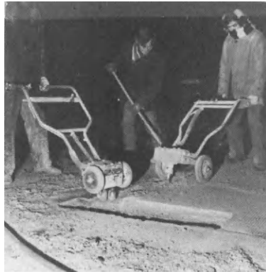
(e) Scabblers and Crack Cutter
