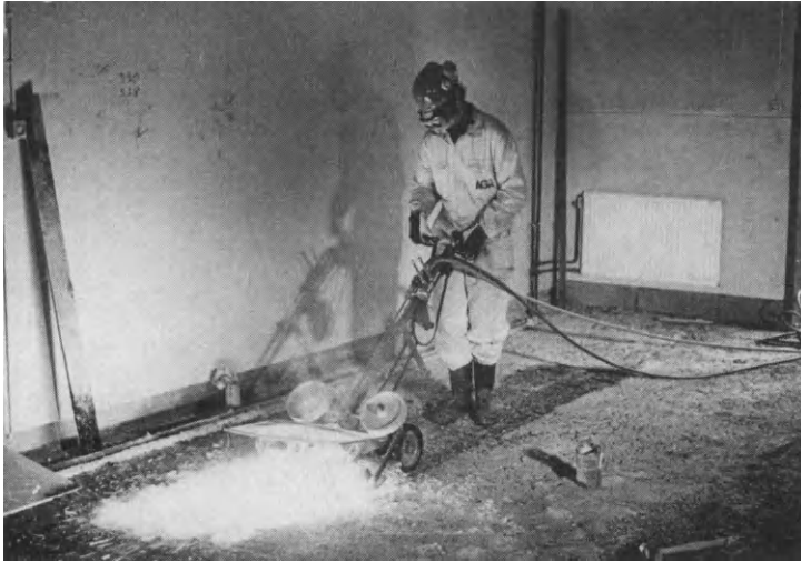
Figure 1 Flame Cleaning a Concrete Floor
