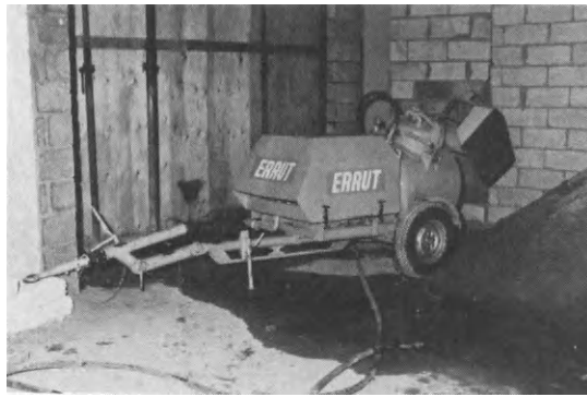
Figure 4 Sand/Cement Screed Pump
