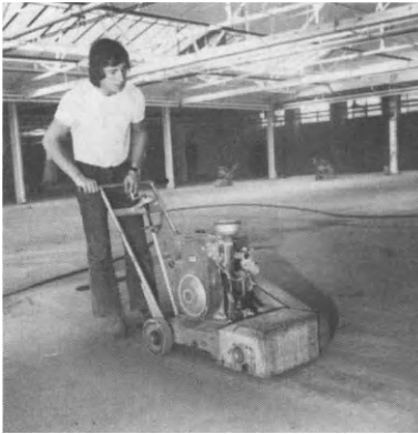
(c) Concrete Grinder
