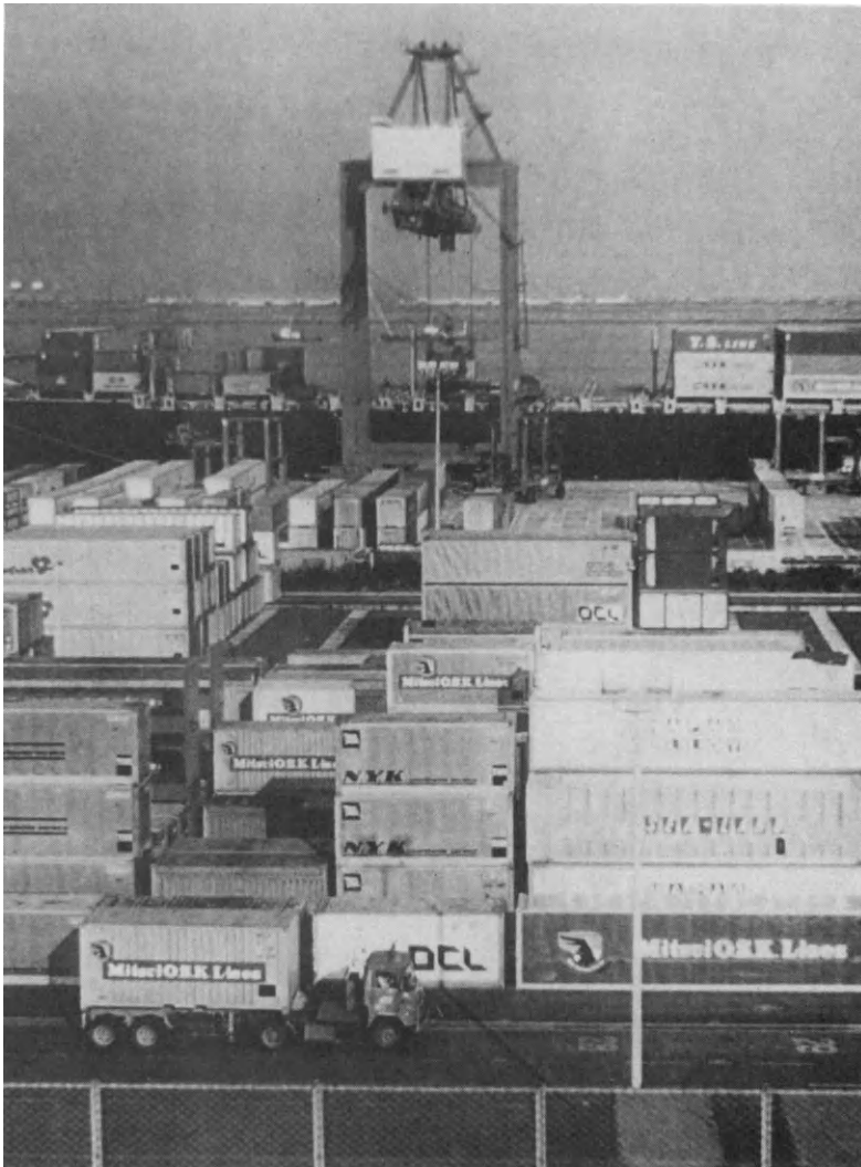
Figure 1 Heavy Loading on a Container Park Pavement from Lorries and Containers
