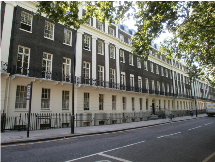
Fig. 7.1 Housing south of Paddington Station. Source Image by the author
