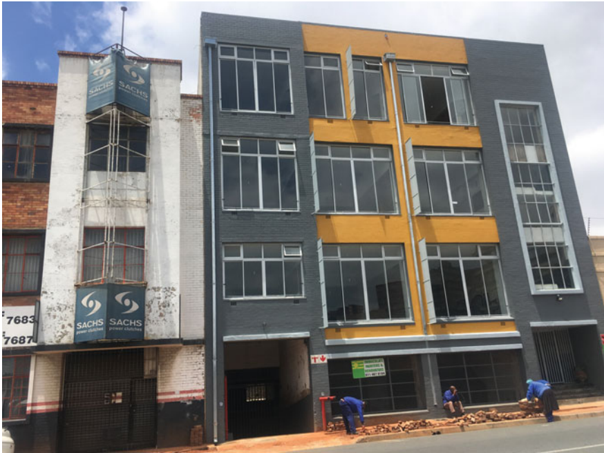
Fig. 5.5 The Main Frame building. Image by the author
