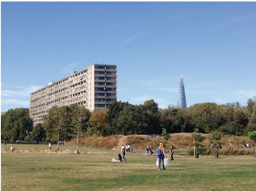
Fig. 4.1 Aylesbury Estate block from Burgess Park. September 2016. Image by the author
