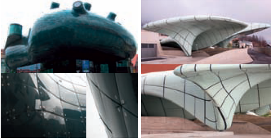
Figure 2: Projects involving double-curved panels where a separate mold has been built for each panel. These examples illustrate the importance of the curve network and the existing difficulties in producing architectural freeform structures. (Left: Peter Cook and Colin Fournier, Kunsthhaus, Graz . Right: Zaha Hadid Architects, Hungerburgbahn, Innsbruck .) Figure taken from [Eigensatz et al. 2010].
