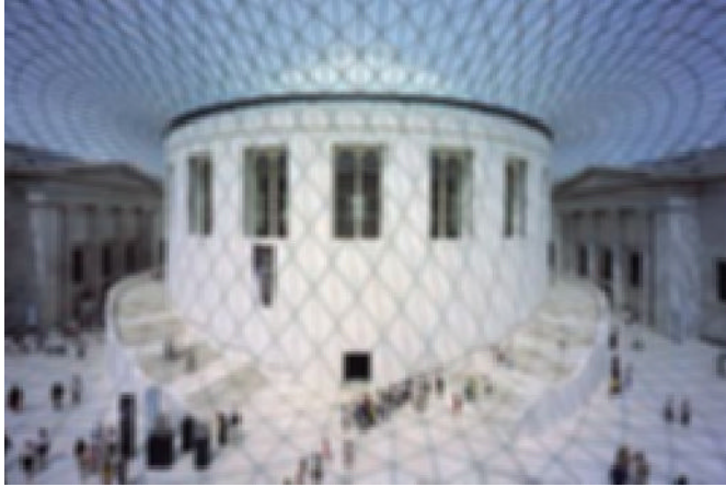
Figure 1: Roof over the Great Courtyard of the British Museum, London, in classical realization by triangular steel/glass panels (Source: http://carpelondinium.wordpress.com ). We present a rationalization by a planar quadrilateral mesh with optimized statics.
