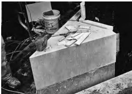
Because the corner is exposed to the gorillas and keepers at grade level, the durable corner was fabricated as a solid unit and beveled to resist chipping. Regenstein Center for African Apes, 2004, Chicago.
