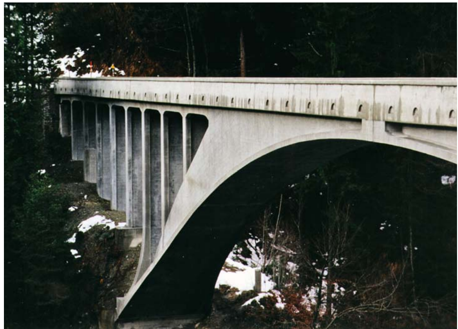
Robert Maillart used static graphics to design the innovative reinforced concrete bridges at Salgina, Switzerland, 1929.
