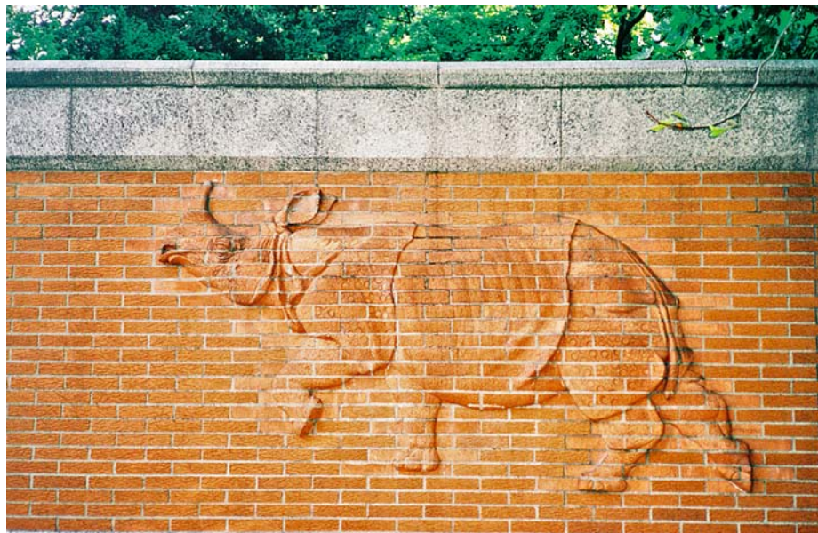
Sculptured brick free of defects, exterior wall of Zoo Berlin.
