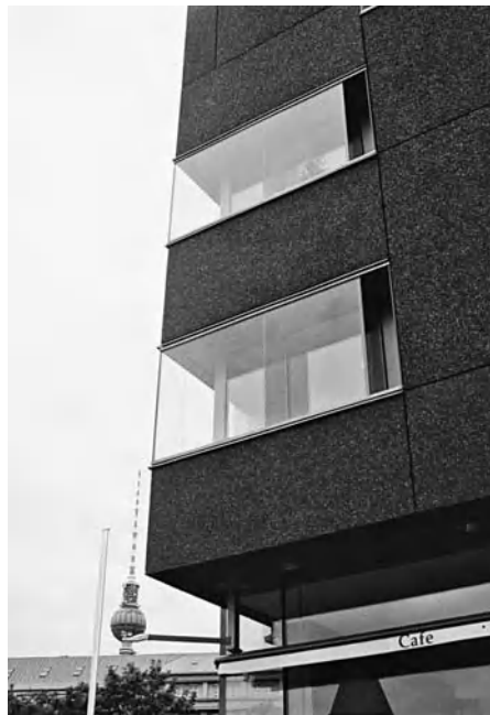
above and right Exposed aggregate in precast concrete panels, Headquarters of Sozialverband Deutschland, Léon Wohlhage Wernik Architekten, Berlin, 2003.
