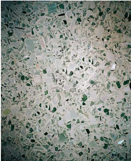
Precast concrete panels using recycled glass as an aggregate can show alkali silica reaction.
