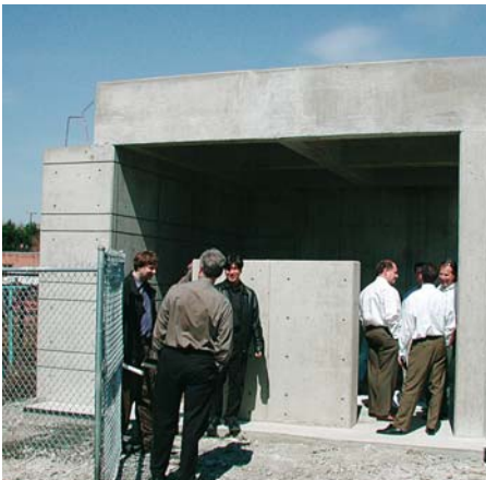
Concrete mock-up for Lincoln Park Zoo, Regenstein Center for African Apes, Chicago, 2004.
