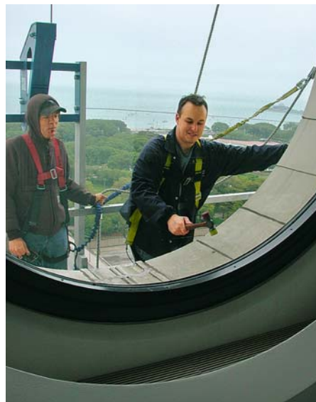
above right Terra-cotta panels are susceptible to corrosion failures.
