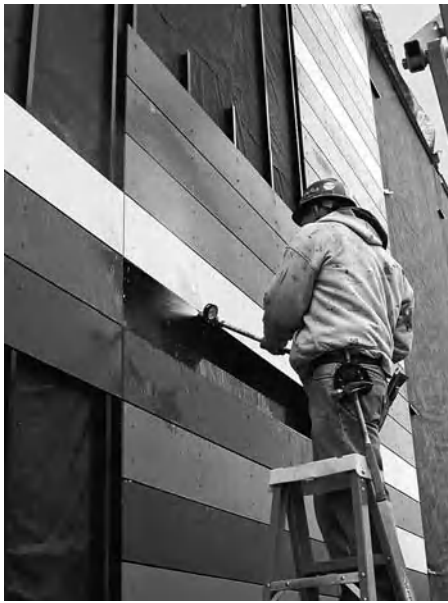
Field water test of cement fiber panel and window system transition. Gary Corner Youth Center, Chicago, 2006.
