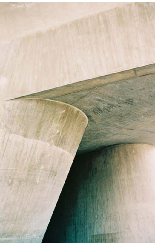
Phaeno Science Center. Self-compacting concrete support elements.
