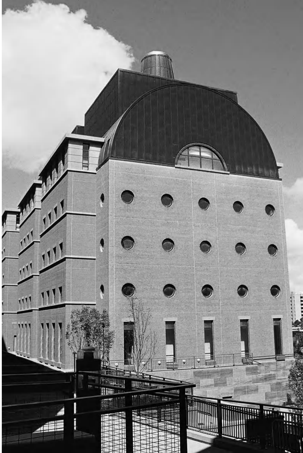
right and below Masonry expansion joints can be an integral part of the façade design. Engineering Research Center (ERC) at the University of Cincinnati, Ohio, 1995.
