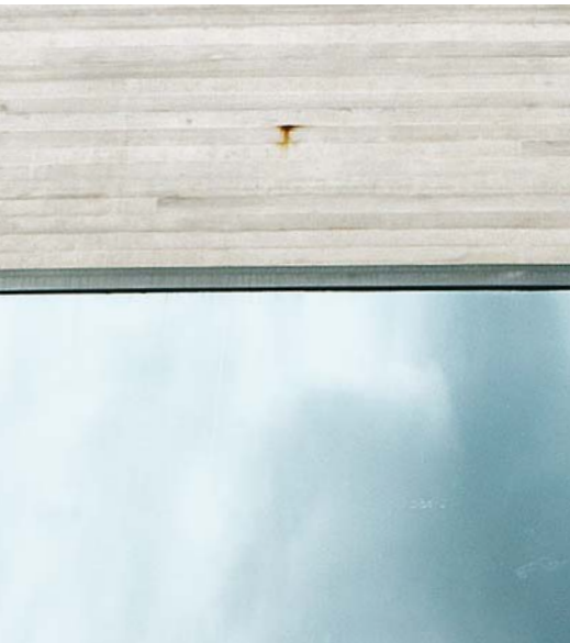
above and right Extension of the Deutsches Historisches Museum, Berlin, 2004. Signs of carbon steel corrosion are visible above the window.
