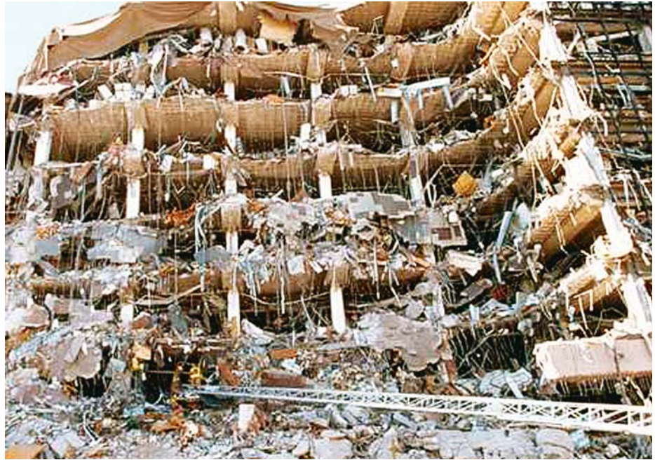
right and below Murrah Building, Oklahoma City. Façade destruction due to impact.
