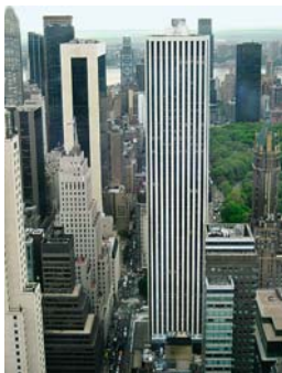
General Motors Building, New York City, 1968. Clad with white marble, with no signs of thermal hysteresis.
