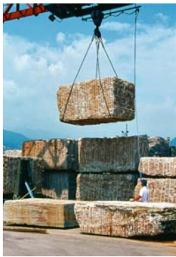
The granite blocks from the quarry were tested during the fabrication process. If results were below minimum specifications, the blocks were rejected.
