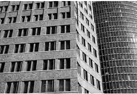
above and right Masonry tower at Potsdamer Platz, Berlin, 2000.
