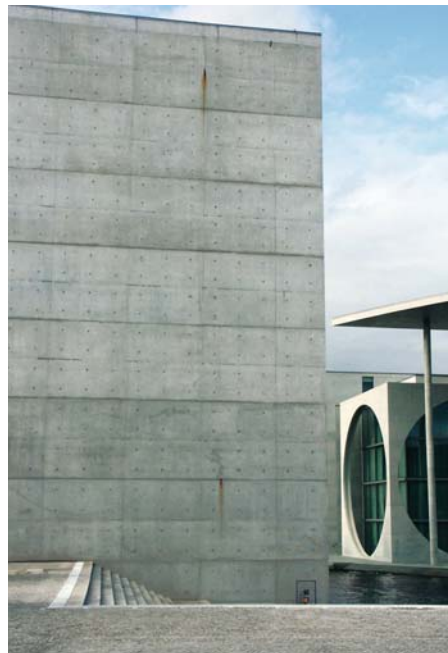
right Paul-Löbe-Haus, Berlin, 2001. Unwanted stains from carbon steel appeared on concrete walls shortly after the project was completed.
