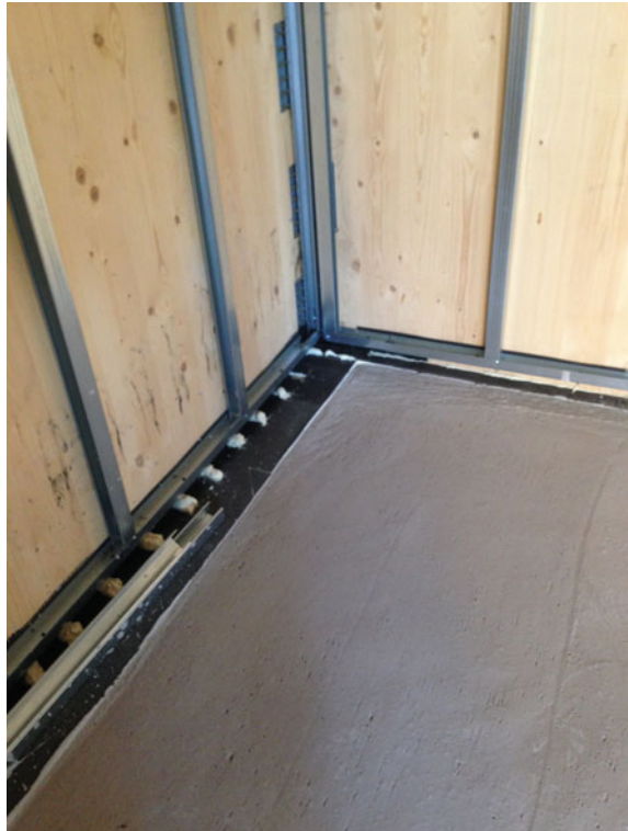
Fig. 7.8 Lightened screed reaches the height of the polyurethane insulation
