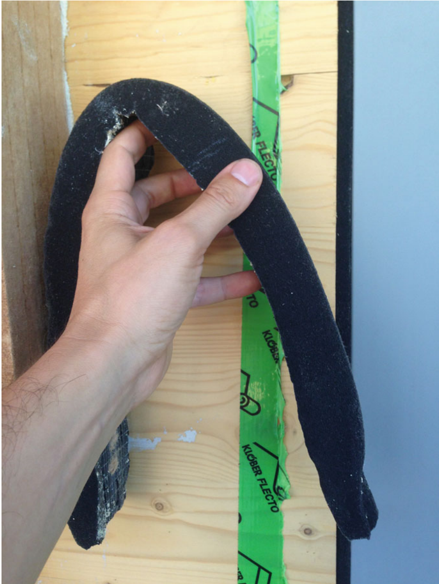
Fig. 8.10 Installation of the frame with expanded butyl tape
