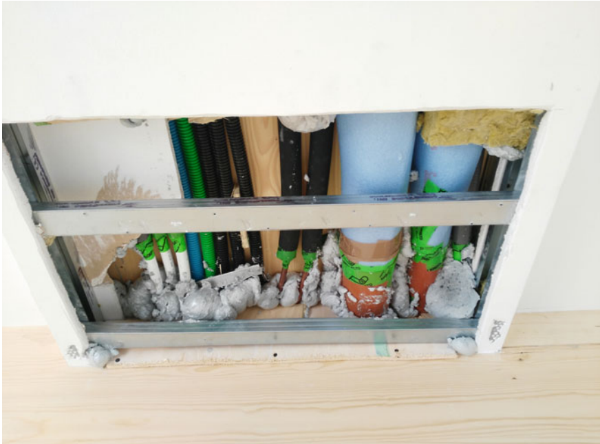
Fig. 8.15 Sealing tapes and polyurethane foams applied on the different types of plants (internal side)
