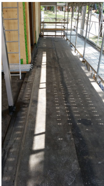
Fig. 4.34 Application of waterproofing sheath on the terraces
