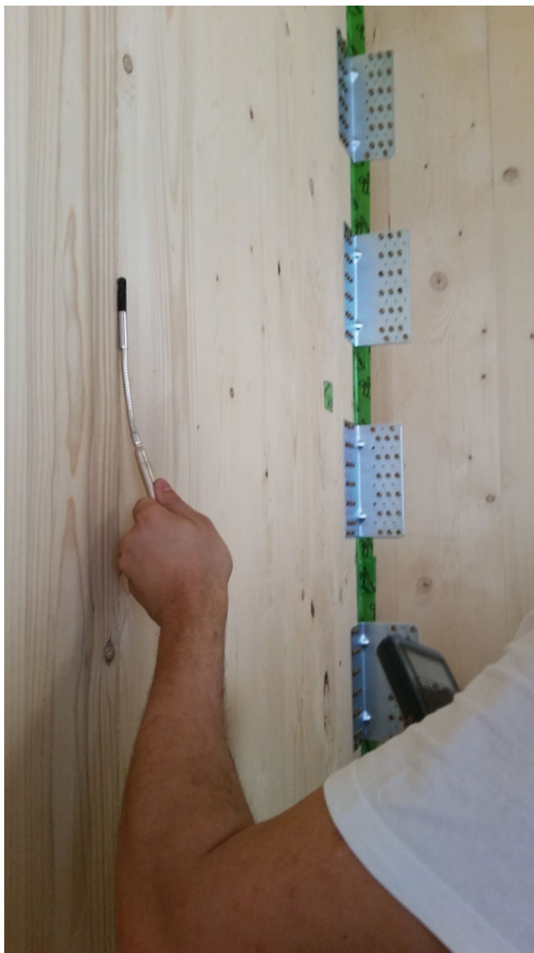
Fig. 8.19 Search for air infiltrations with the anemometer
