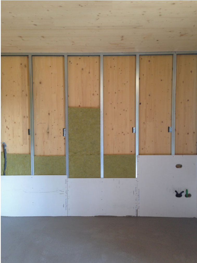
Fig. 5.2 Internal wall covering
