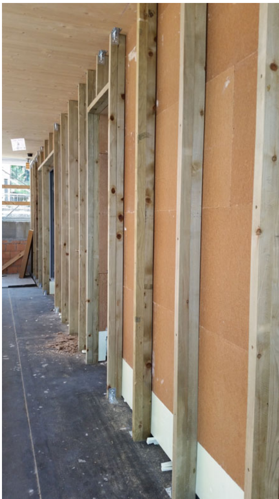
Fig. 5.6 XPS panel at the base of the wood fibre panels
