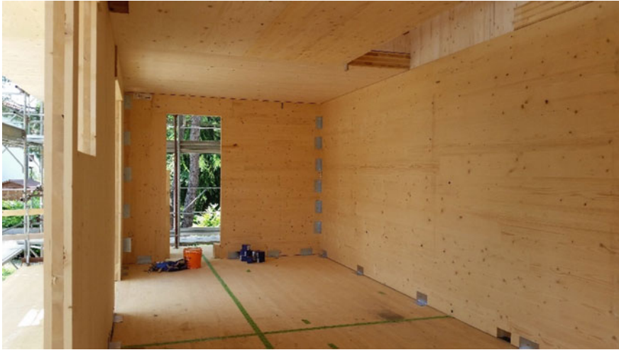
Fig. 4.17 Internal view of the structure in CLT
