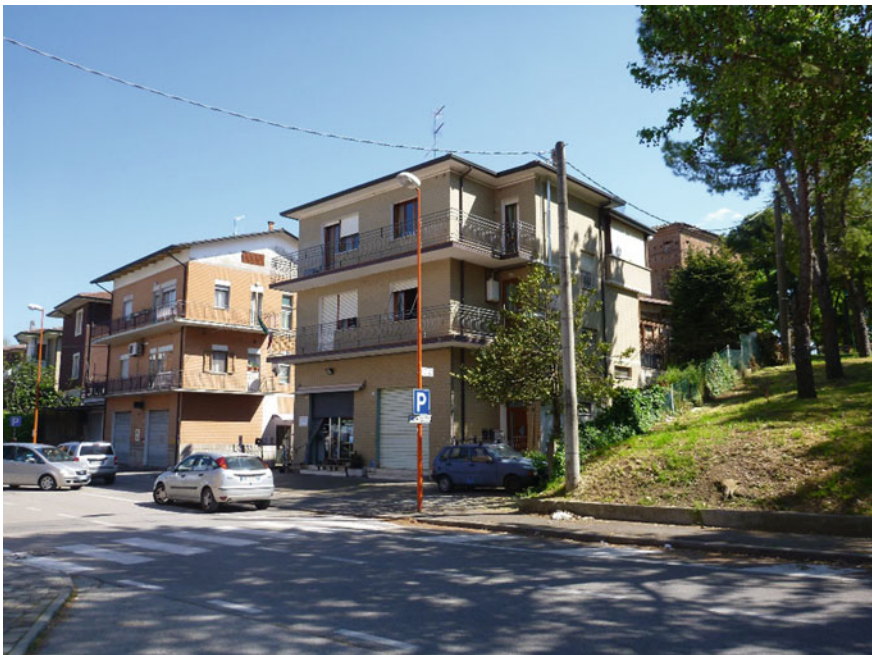
Fig. 1.1 Building owned by the Zoffoli family, subject of the intervention
