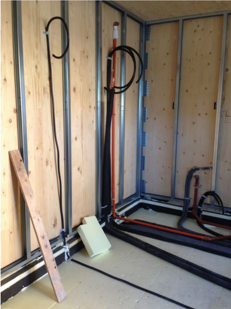
Fig. 9.19 Technical systems on the ground slab. The insulation is continuous and there is no interference with the technical systems
