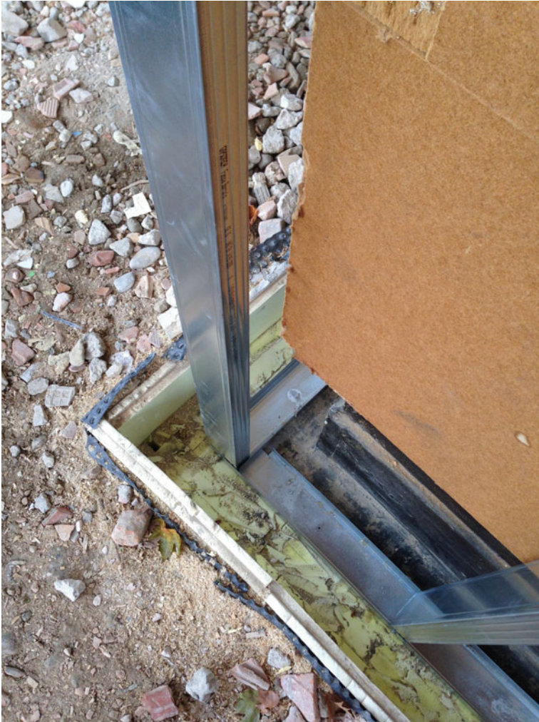
Fig. 5.14 Application of the studs on the foundation's kerb
