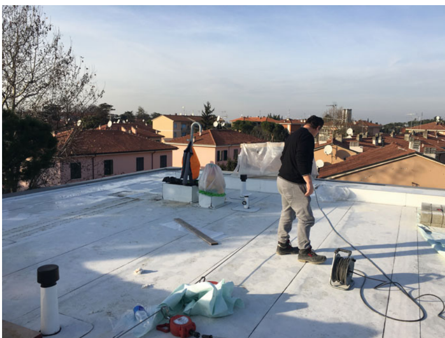
Fig. 5.23 Laying of the bitumen-based sheath with reflective white surface
