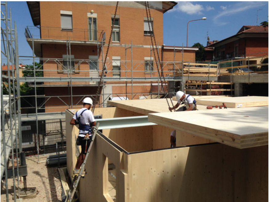
Fig. 4.30 Laying of the panel in CLT which constitutes the first-floor slab
