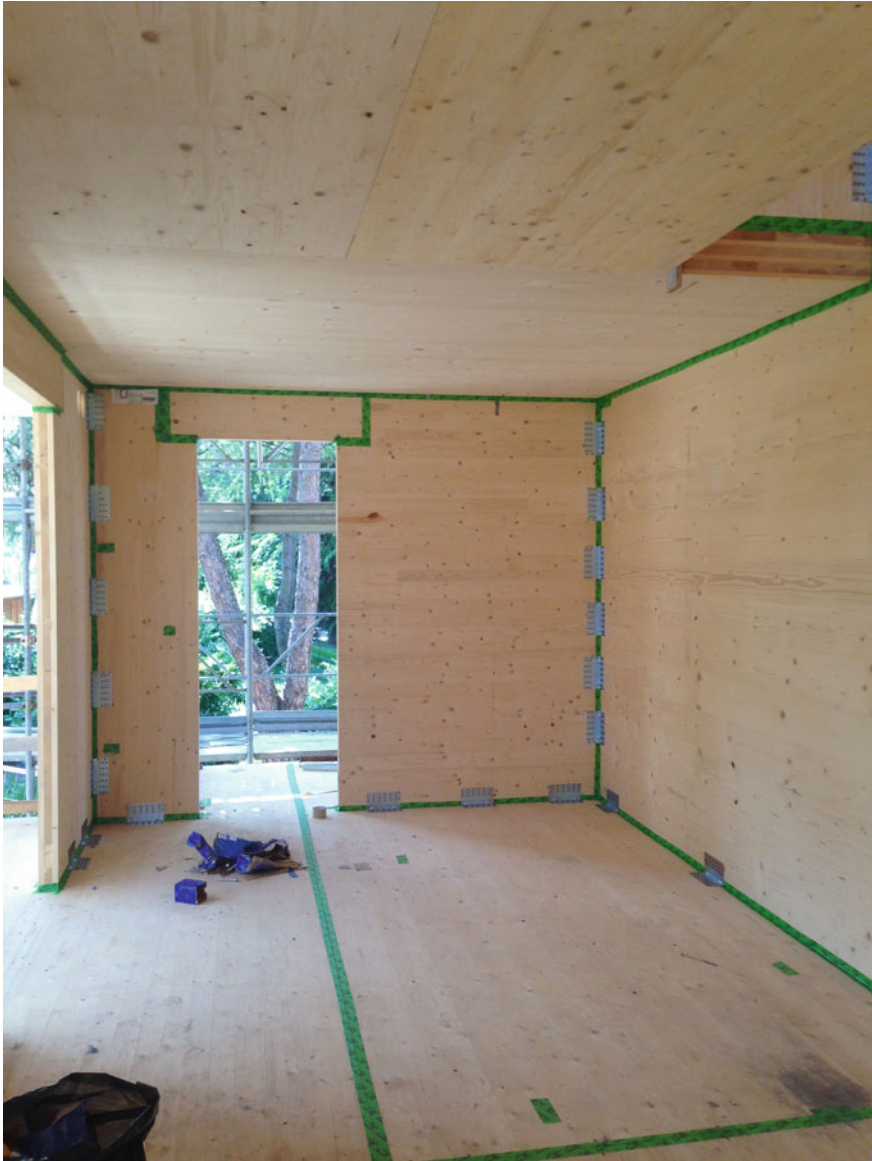
Fig. 8.3 Sealing of the joints on the internal side with sealing tape
