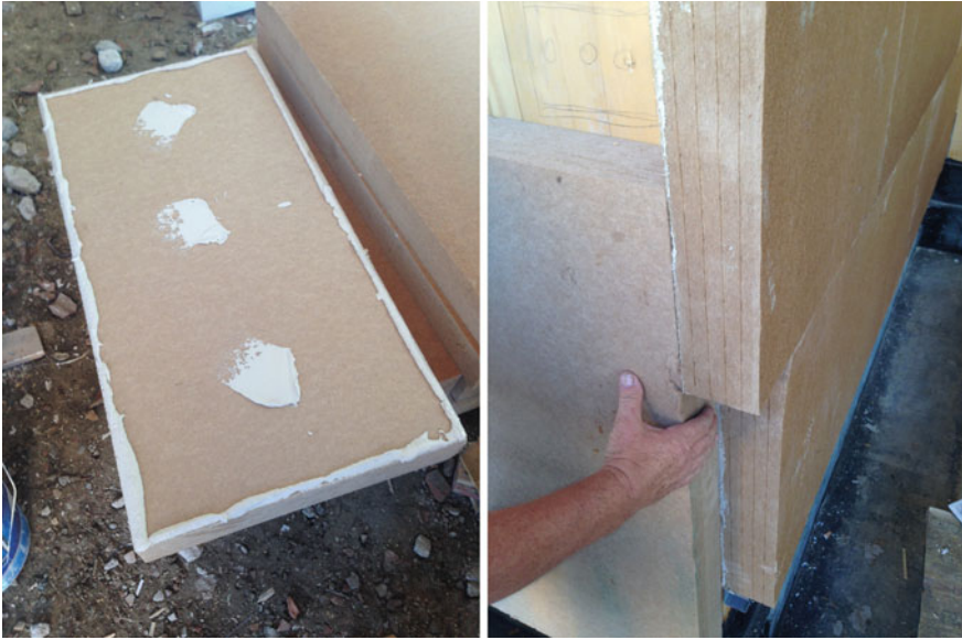
Fig. 5.3 Bonding phases of the wood fibre
