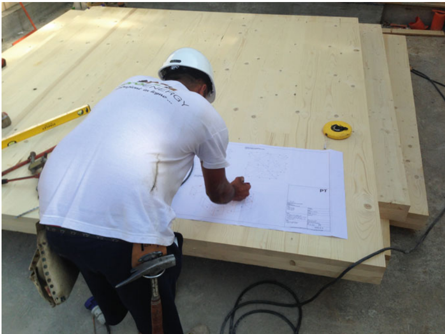
Fig. 4.25 Worker studying the laying diagram of the panels in CLT
