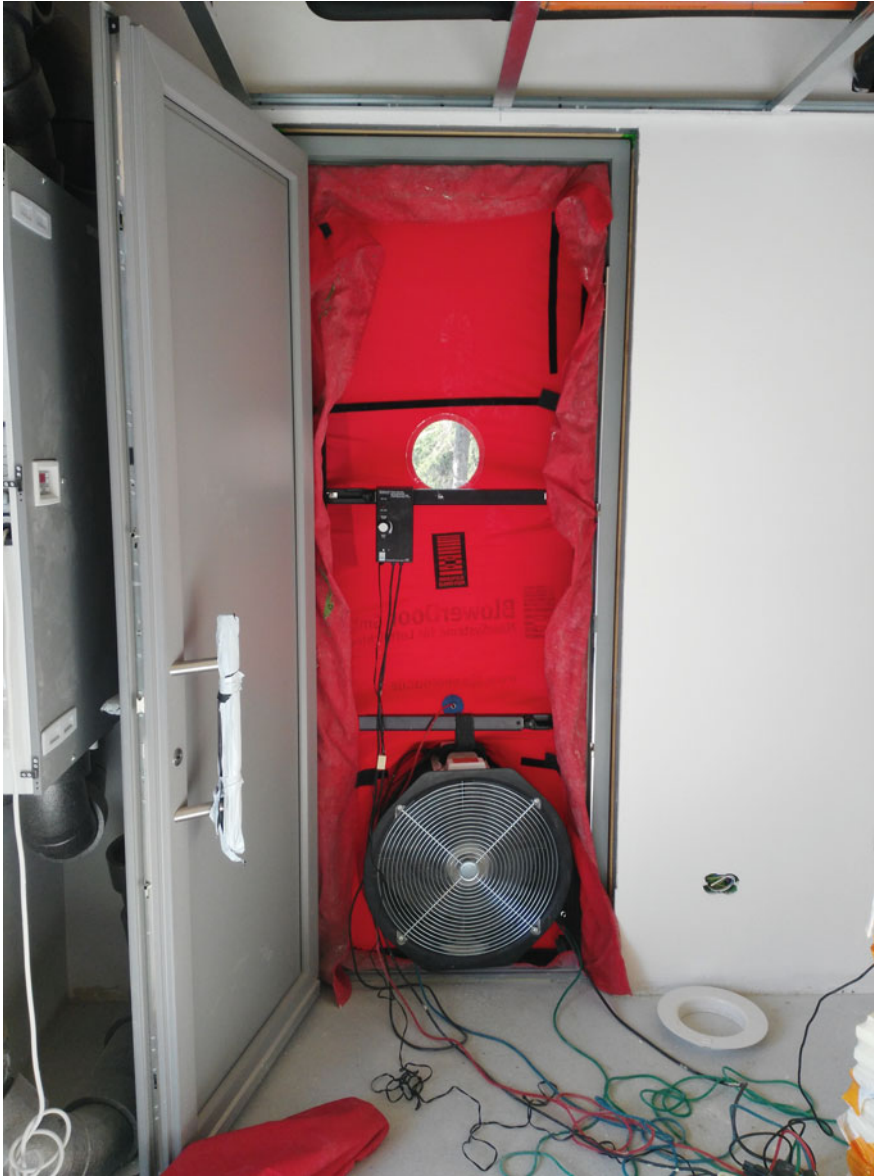
Fig. 8.20 Installation of the fan for the blower door test (internal view)
