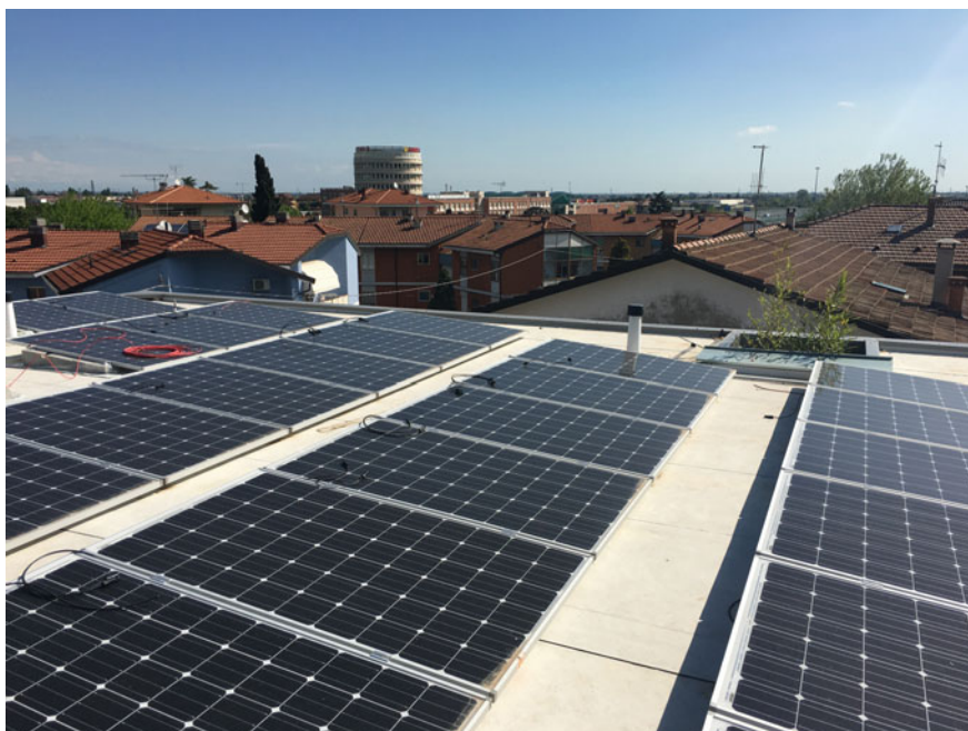
Fig. 9.20 Installation of photovoltaic panels in the roof
