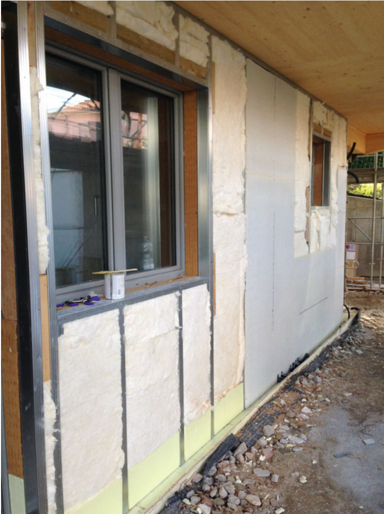
Fig. 5.16 Application of the fiberglass panels and cladding with panels in fibre cement
