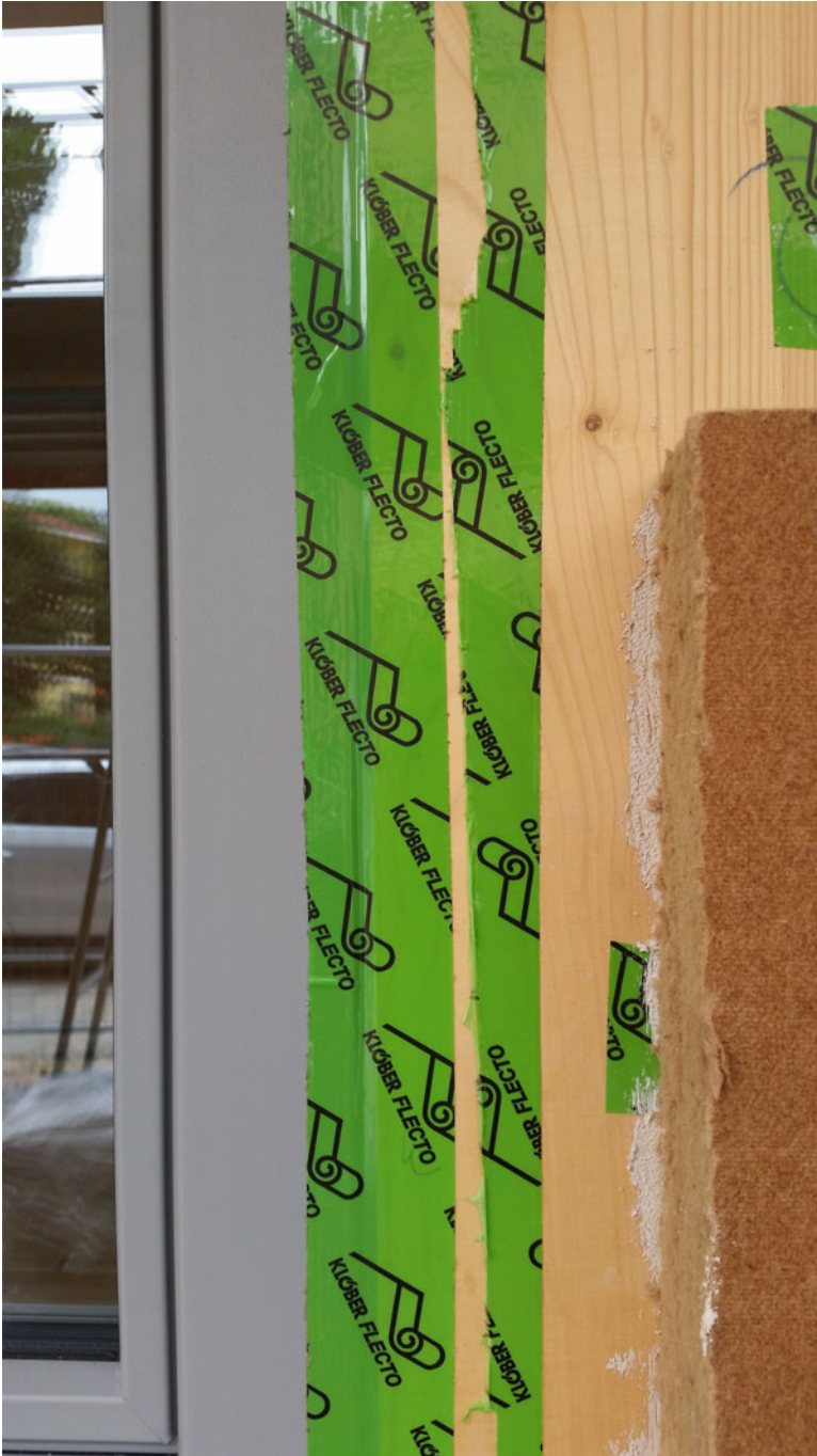
Fig. 8.11 Application of the sealing tape
