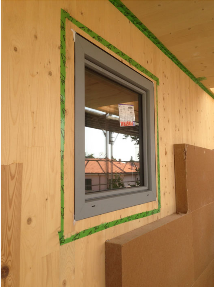
Fig. 5.32 Window inserted in the panel of CLT without using the subframe
