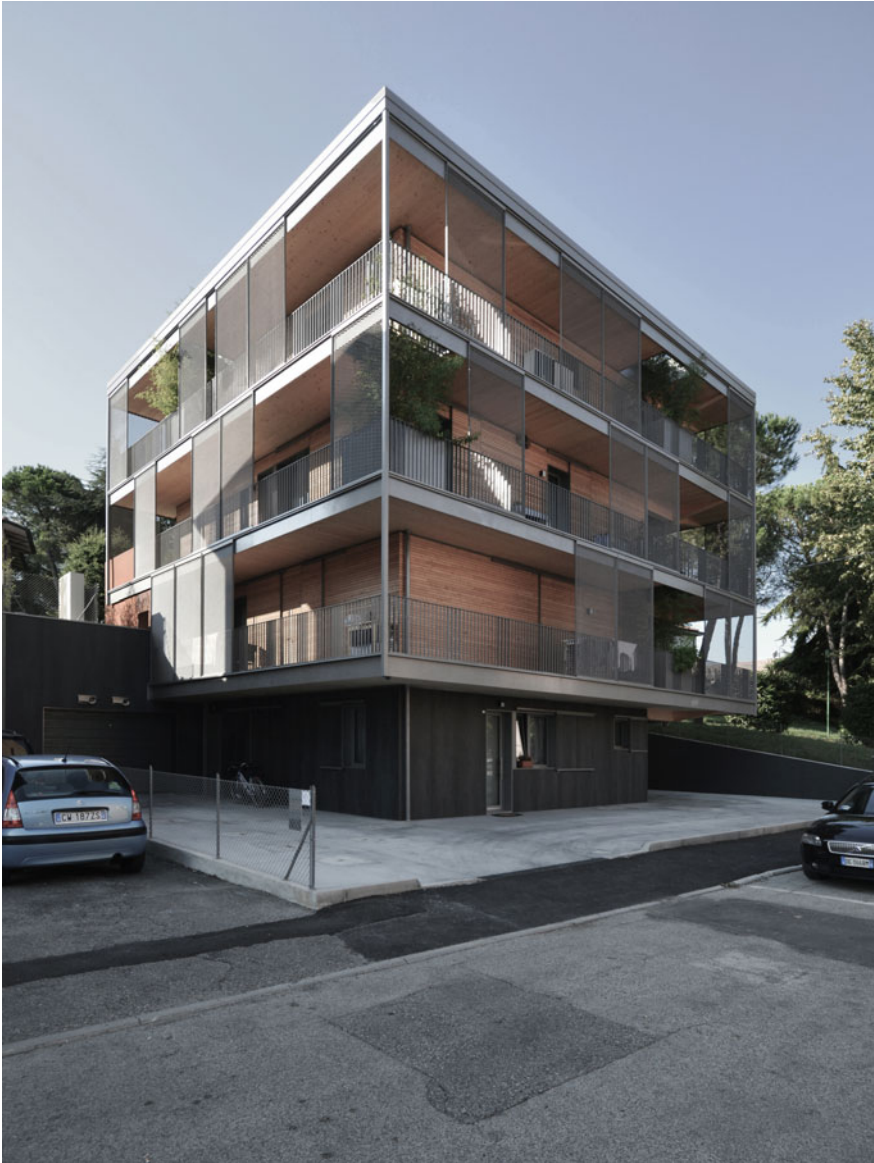
Fig. 11.13 View from Via Ariosto, east and north faces
