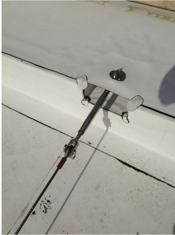
Fig. 7.45 Steel pin for the fixing of the line life at completion
