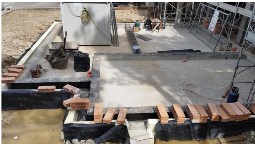
Fig. 4.22 Insulation of the external kerbs
