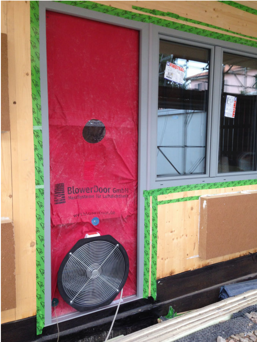
Fig. 8.17 Installation of the fan for the blower door test (external view)
