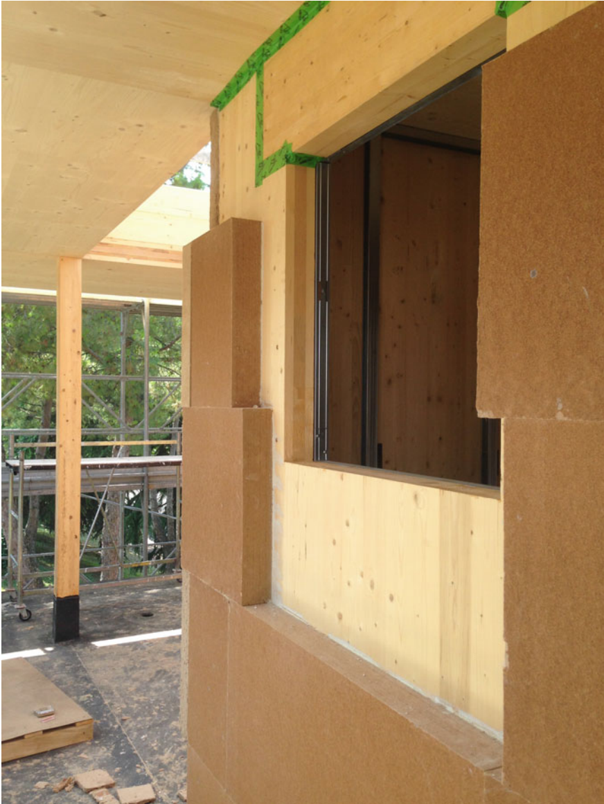
Fig. 8.7 Taping in the presence of the architrave of the windows
