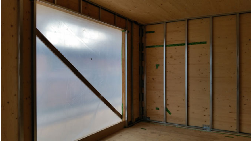
Fig. 8.21 Closing of the holes of the windows with taped PVC sheets
