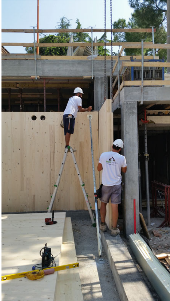
Fig. 4.20 Dry structure and wet structure
