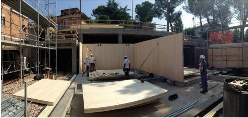
Fig. 4.19 Panels in CLT resting on the kerbs of the foundation
