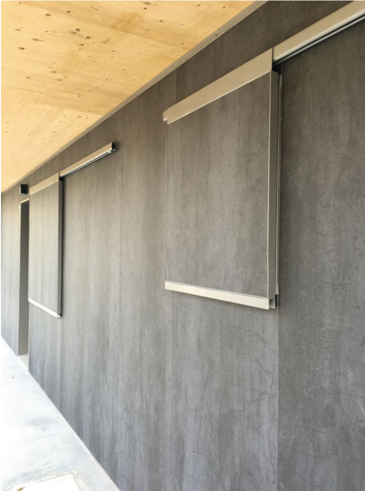
Fig. 5.17 Cladding in ceramic slab
