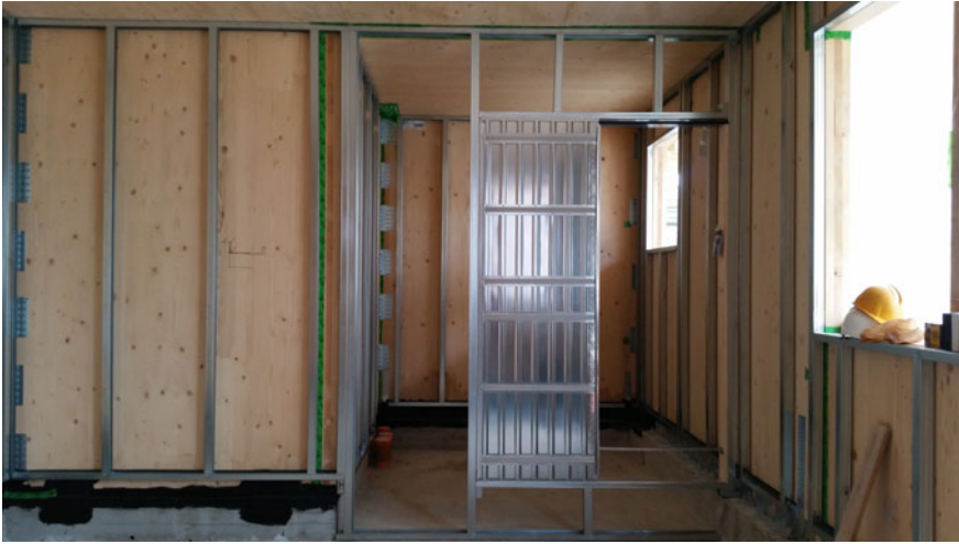
Fig. 5.28 Ground slab prior to the installation of the insulating panels
