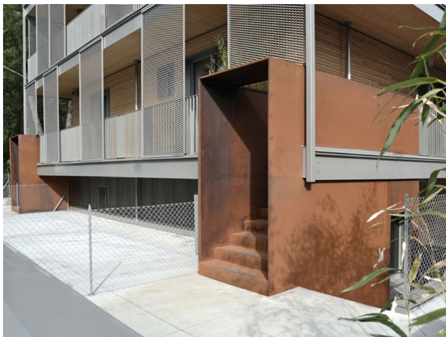
Fig. 11.21 Detail of the accesses on Via Liguria made in Corten steel sheet
