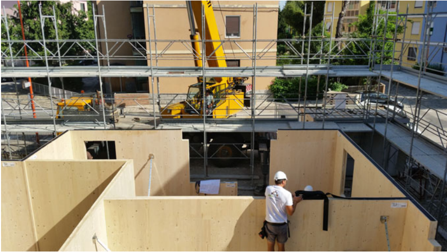
Fig. 4.29 Application of the sound insulating joint
