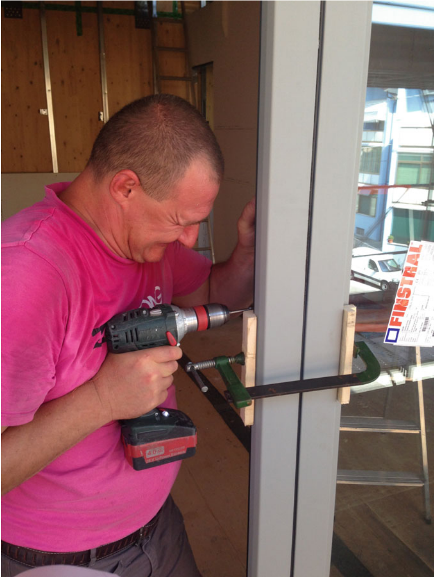
Fig. 8.22 Tightening of the screws to compress the expanded butyl tape
