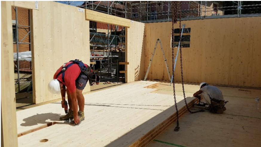
Fig. 4.16 Preparing for the lifting of a panel in CLT
