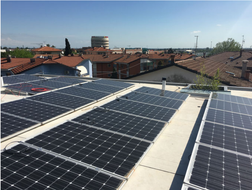
Fig. 5.24 Installation of photovoltaic panels on the roof covering
