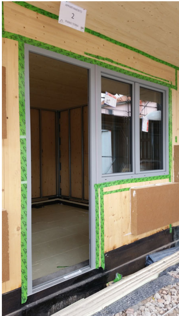
Fig. 5.30 Window integrated into the entrance door
