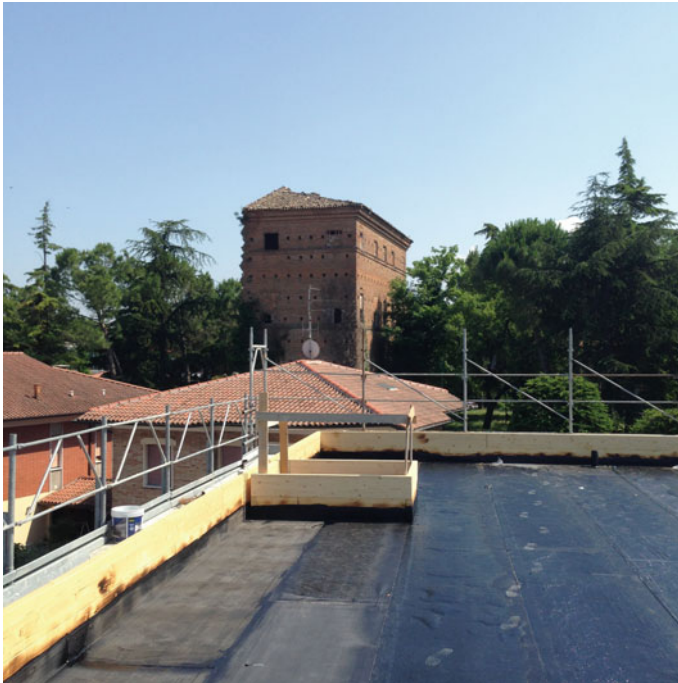
Fig. 4.31 Waterproofing of the roof slab panel in CLT
