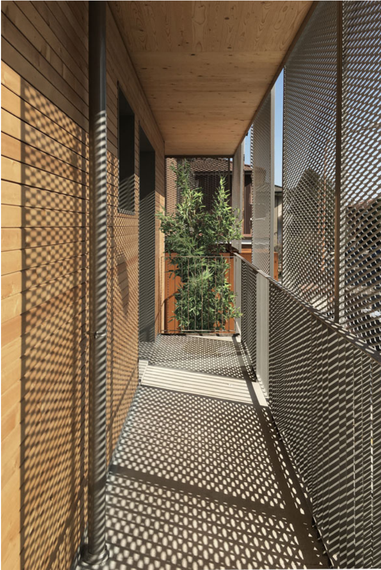
Fig. 11.27 View inside the terraces
