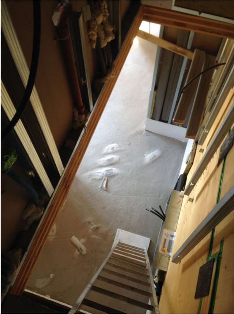
Fig. 9.17 Technical systems are covered by the 12-cm-thick lightened screed
