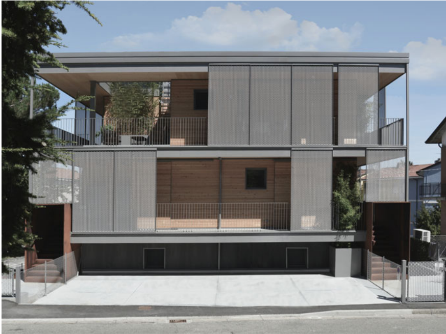
Fig. 11.14 View of the south face from Via Liguria. The photograph was taken in the summer: the awnings systems, overhangs and sliding panels shield the solar radiation
