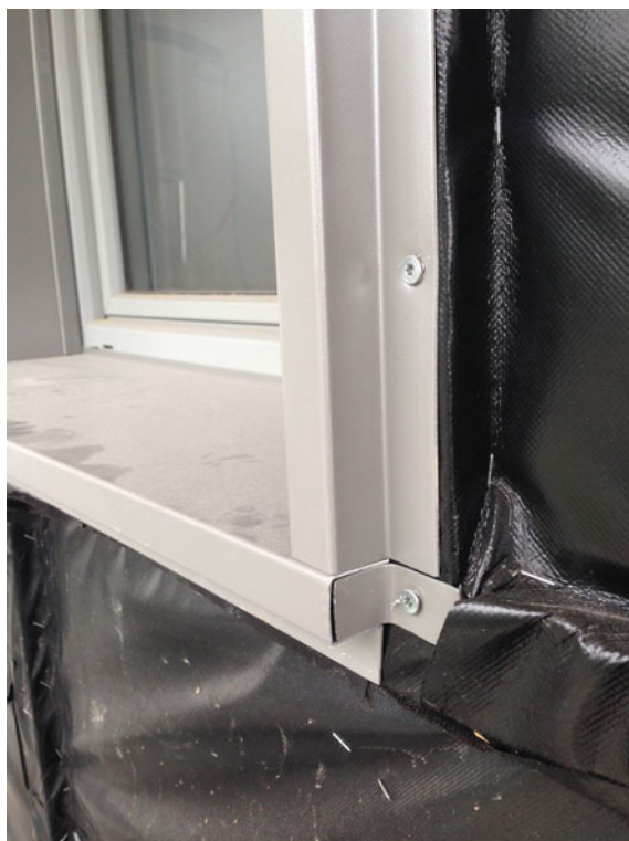
Fig. 7.36 Installation of the window sills in painted aluminium sheet
