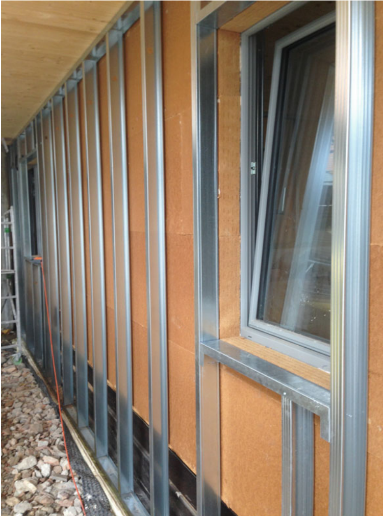
Fig. 5.13 Application of the sheet metal studs
