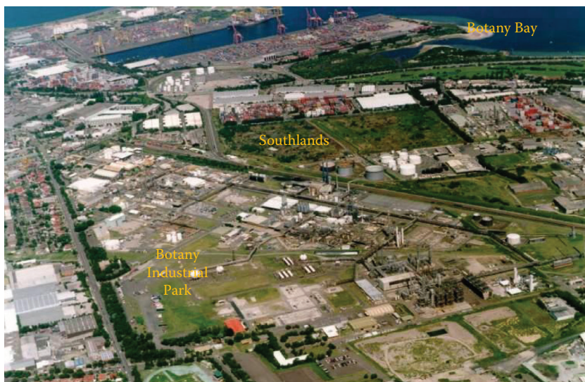
FIGURE 12.2 BIP and surrounds. (From Orica Ltd.)
