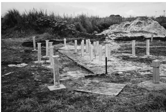
FIGURE 12.9 The completed pilot-scale reactive iron barrier with a protective concrete cap. (From Orica Ltd.)
