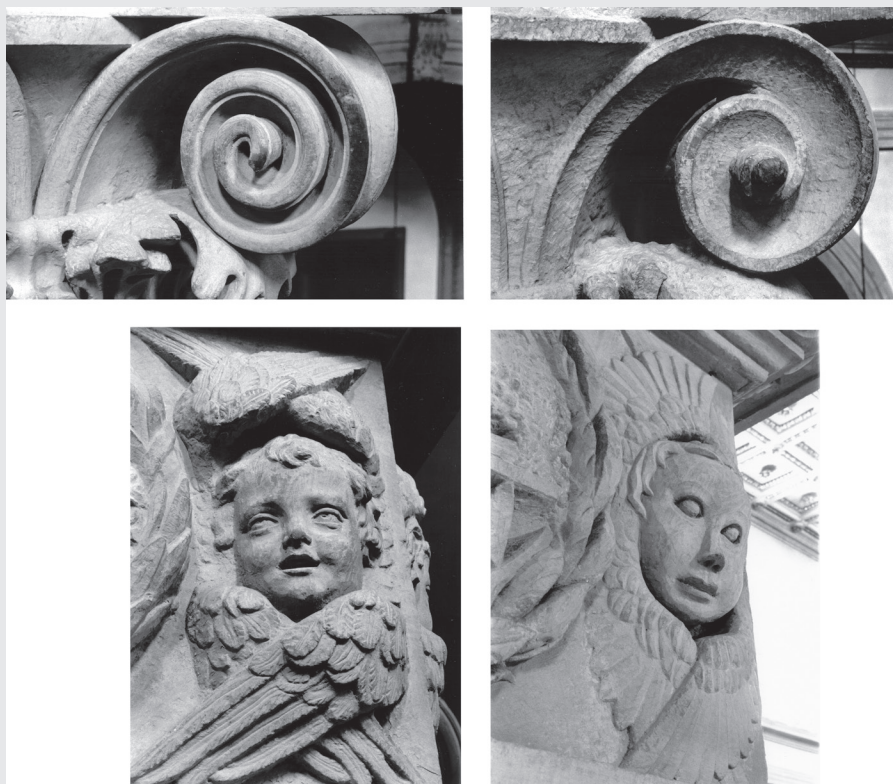
Figure 6.10 Images on the left are of detailing on the western bays of San Lorenzo, while the images on the right are from the eastern bays. From this striking difference in quality, Cohen infers a significant gap in time during construction. By permission of Matthew A. Cohen.
