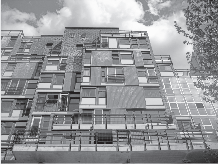
Figure 4.3 La Maison Medicalé (La Mémé) in Woluwé-Saint-Lambert, Brussels: Lucien Kroll designed the exterior as a framework such that students could create and change their own façade by choosing among its various finishes, sizes, and removable panels. Image (and text) courtesy of Kush Patel, PhD student, University of Michigan Taubman College of Architecture and Urban Planning.
