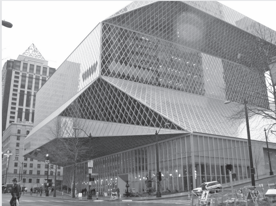
Figure 12.8 Exterior of Seattle Public Library by Rem Koolhaas. Photograph courtesy of David Wang.
