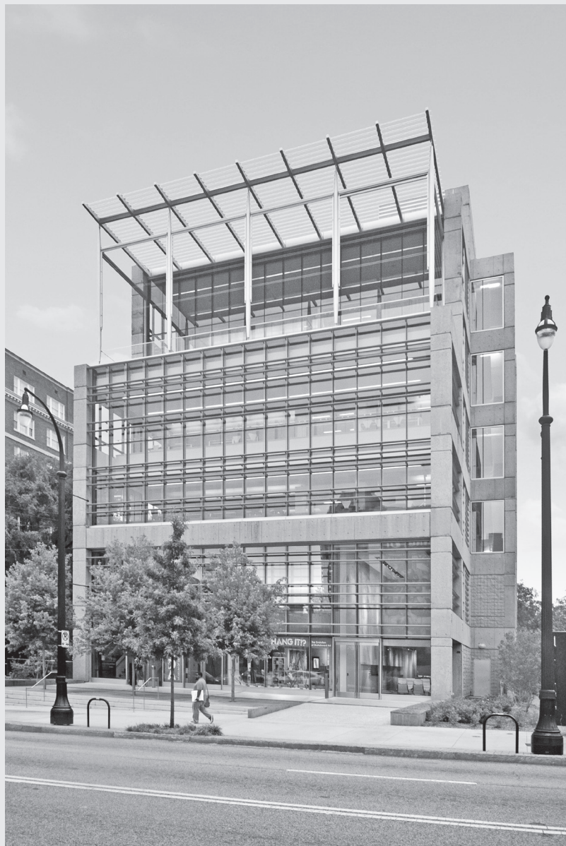
Figure 7.22 New 1315 Peachtree St. office building. Image courtesy of Perkins + Will. © Eduard Hueber/archphoto.
