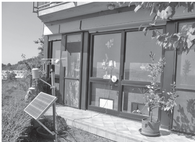
Figure 9.20 Exterior view of the Trombe wall. Courtesy of Elsevier.
