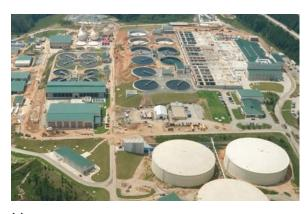
✓ Figure 26.9 Traditional sewage treatment. (a) A municipal wastewater treatment facility. (b) The traditional sewage treatment process. Microbial digestion during secondary treatment removes most of the biochemical oxygen demand (BOD) before the water is chemically treated and released; dried sludge is recycled as landfill.
