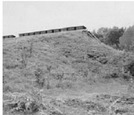
Figure 2.58 The Hockerton development near Newark, Nottinghamshire, makes use of thermal mass and earth banking to provide a stable internal environment
