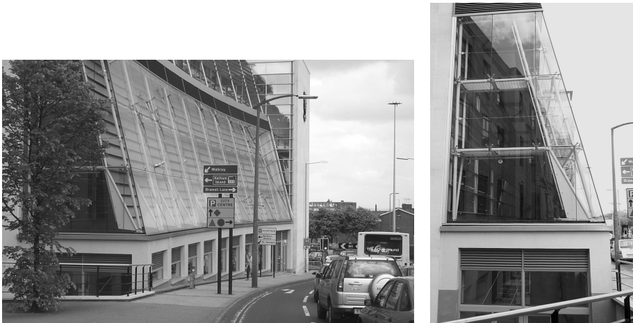
Figure 2.23 An example of internal solar shading – effective at preventing direct sunlight hitting people or surfaces within the space but not as effective in reducing solar heat gains as it would be if positioned on the outside
