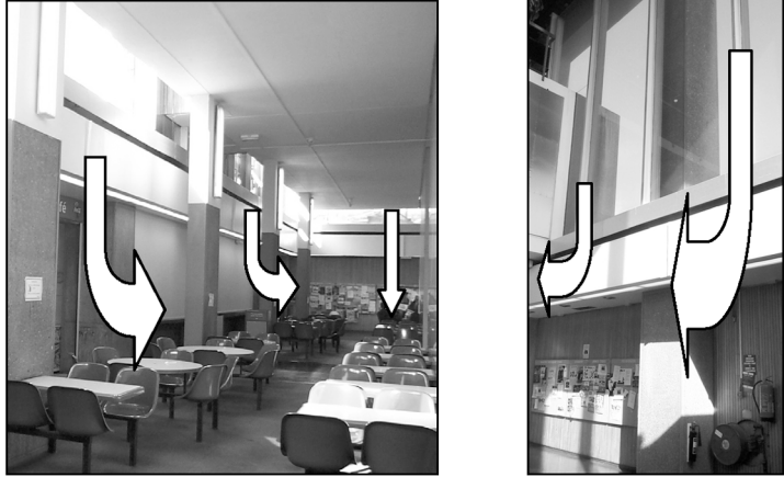
Figure 2.8 Illustration of downdraught possibilities where there are large glazing areas at high level
