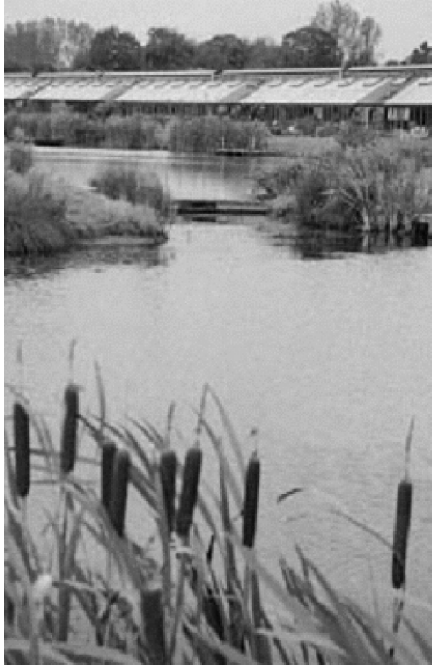
Figure 2.58 The Hockerton development near Newark, Nottinghamshire, makes use of thermal mass and earth banking to provide a stable internal environment
