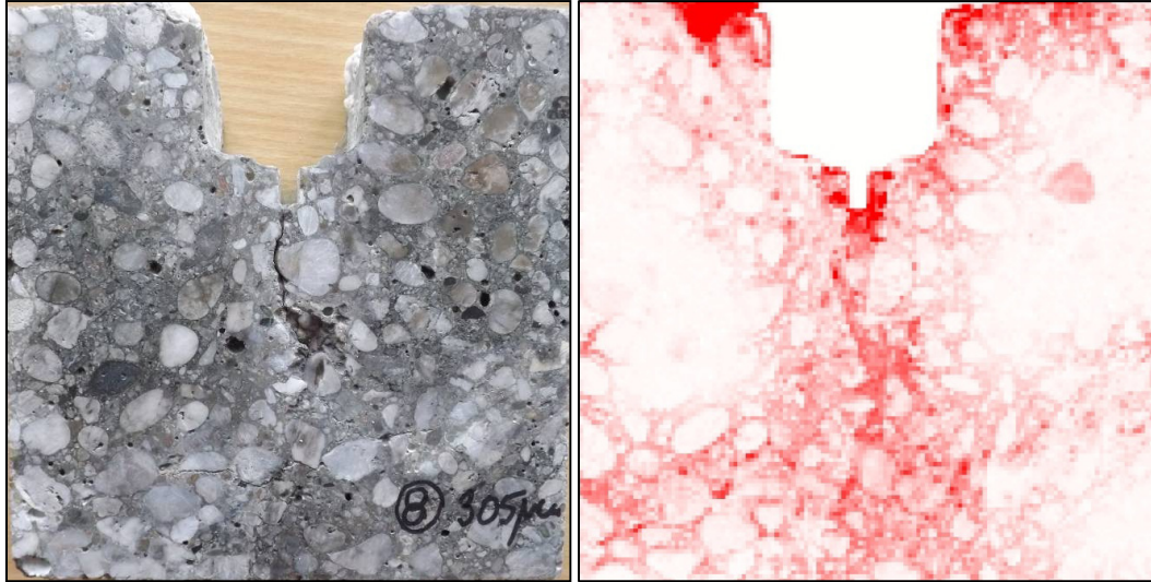
Figure 5. Left: Photo of the cross section of a cracked concrete specimen; sample-size 140 mm × 140 mm; crack width 305 µm. Ingress of NaCl-solution from the top. Right: Color coded chlorine intensity on same specimen; dark red represents high chlorine content.
