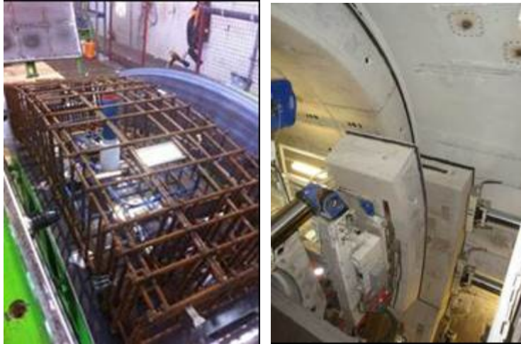
FIGURE 4. Precast of an instrumented segment and assembly of a ring
