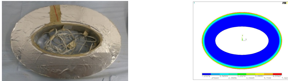
(a) crack position (b) circumferential stress contour at 7 th day
