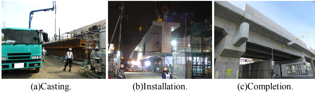
Figure 1. Measured PC girder.
