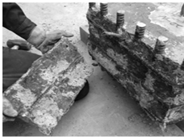
(a) Removed cover concrete
