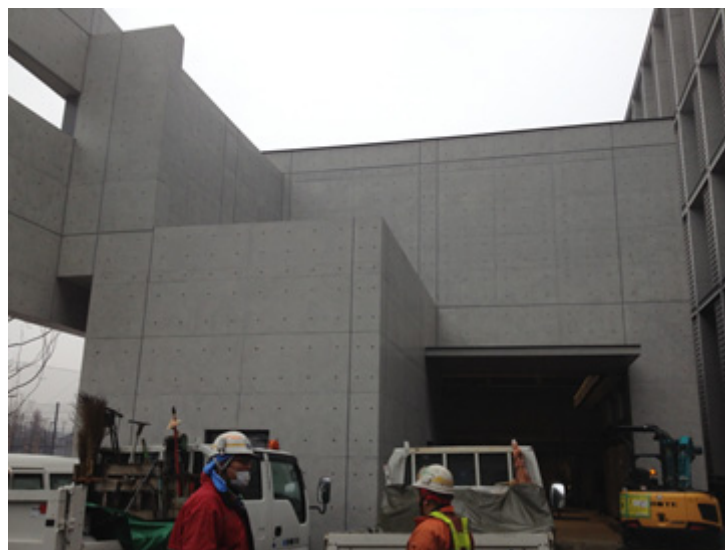
Picture-1 Appearance of the structure
