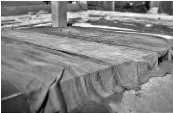
FIGURE 6.16 Curing by using cloth.
