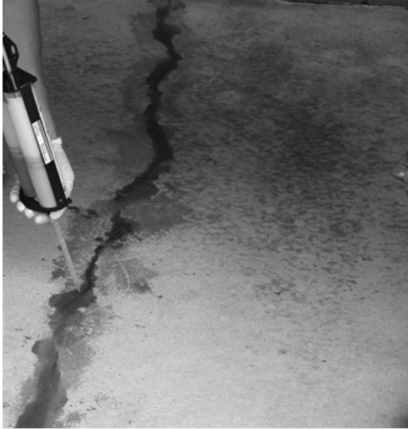
FIGURE 8.28 Repair of wall with epoxy.
