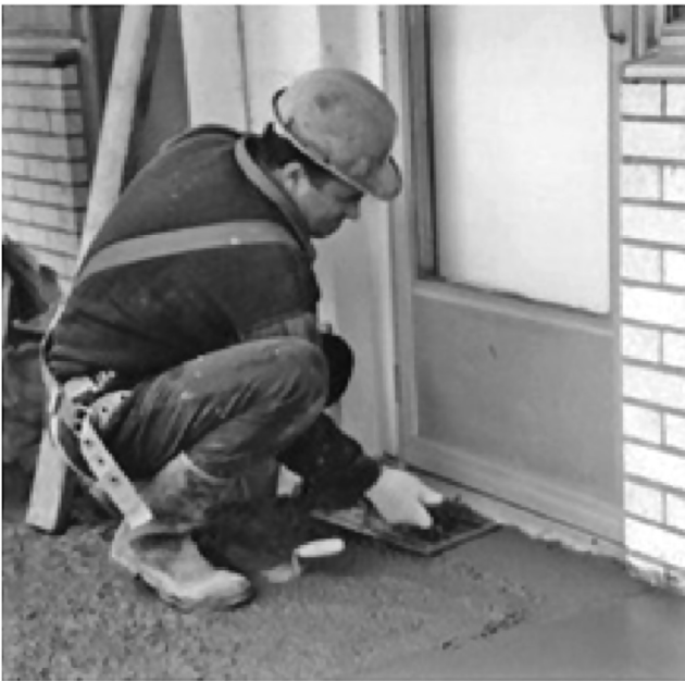
FIGURE 8.13 Manual method for repair.
