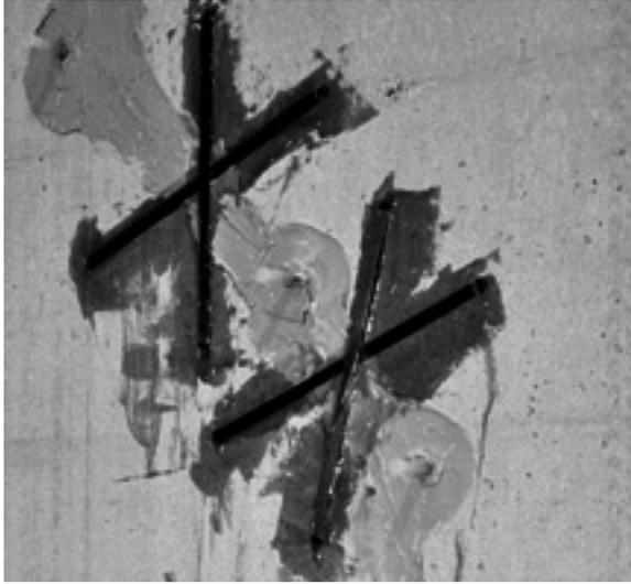
FIGURE 8.30 Repair of wall cracks by CFRP method 1.
