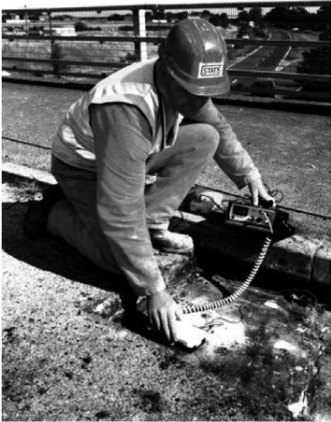
FIGURE 4.22 Concrete cover measurement to a bridge deck.
