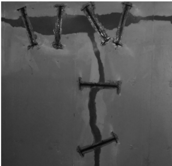
FIGURE 8.31 Repair of wall cracks by CFRP method 2.
