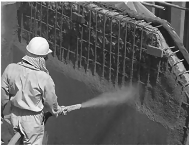
FIGURE 8.16 Using shotcrete.
