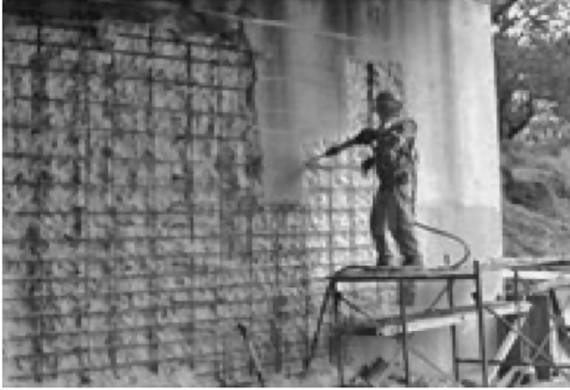
FIGURE 8.3 Using a pneumatic hammer to remove wall concrete cover.
