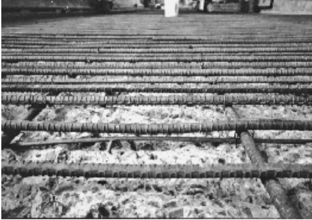
FIGURE 8.5 Concrete surface after using a water jet.
