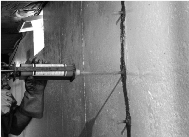
FIGURE 8.29 Repair of floor with epoxy.
