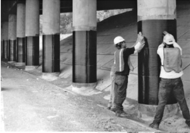
FIGURE 8.27 Column repair.
