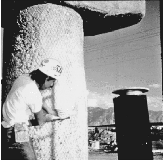
FIGURE 7.11 Fixing titanium on a concrete column.
