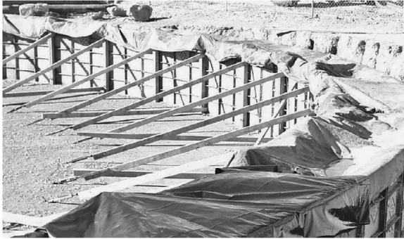
FIGURE 6.18 Plastic sheet to protect from evaporation.
