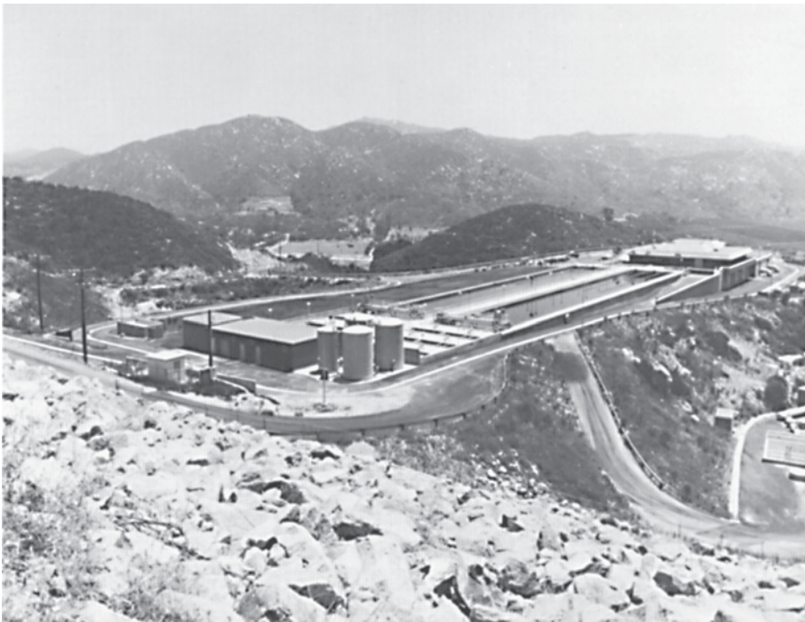
FIGURE 21.10. 75MGD (ult.) Water Treatment Plant for the City of Escondido, Vista Irrigation District, California, “Substantially Completed.”
