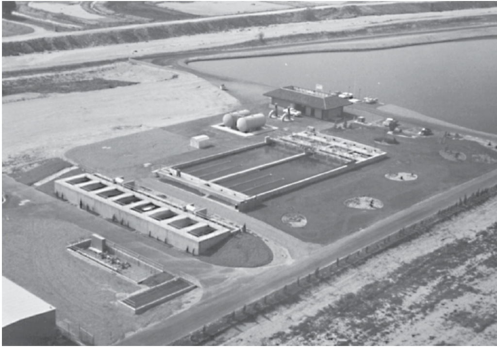
FIGURE 16.1. Typical EPA Clean Water Grant Project Requiring a Separate Value Engineering Contract.
