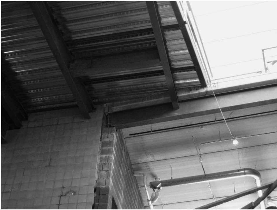
FIGURE 5.22. Photo of a Complex Connection on a Job Site.
