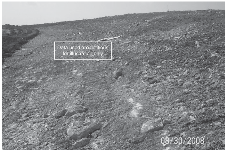
Rough slope trimming at SW side
