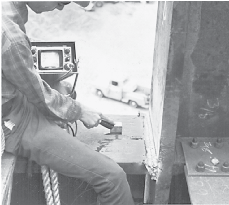
FIGURE 18.7. Ultrasonic Testing of Structural Field Welds.
