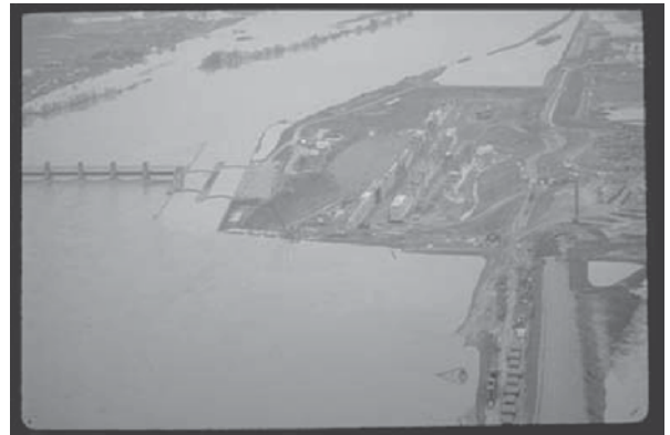
FIGURE 20.7. Suspension of Work Necessary Because High Water Threatened to Flood the Lock Construction Site.
