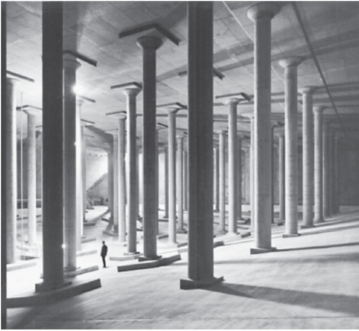
FIGURE 4.14. Typical Public Relations Photograph of Construction. Greystone Reservoir, City of Beverly Hills, California. Engineers: Montgomery-Watson Consulting Engineers, Pasadena, California.
