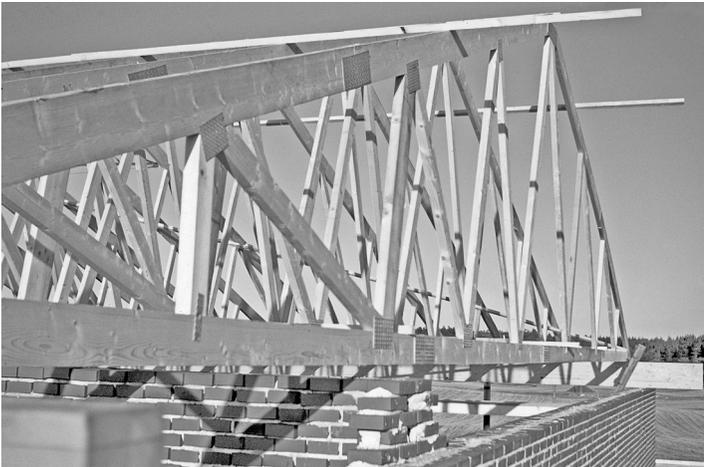
Fig. 3.2 Trusses with punched metal plate connectors spanning from façade to façade. The members carrying the roof covering are not shown
