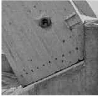
Fig. 2.33 Dowelled joint between glulam arch and cast-in steel plate
