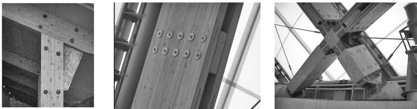
Fig. 2.31 Bolted structures
