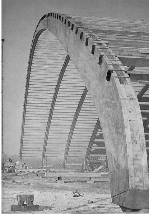
Fig. 3.3 Glulam arches spanning 80 m at 8 m centres carry glulam joists
