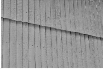
Ensure that the wood can move freely; use overlap joints rather than butt joints
