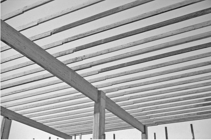
Fig. 3.1 Structural timber joists supported by glulam beams
