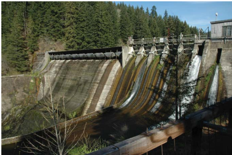
Figure 17.2 Condit Dam on the White Salmon River, Washington State, USA. This dam measured 38 m high and 144 m wide, and provided 80,000 MWh of power generation per year. The dam also resulted in the loss of 53 km of salmonid habitat. Breach of the dam occurred on October 26, 2011, and it was subsequently removed. (Photo by A. Yeakley). (See colour plate section for colour figure).
