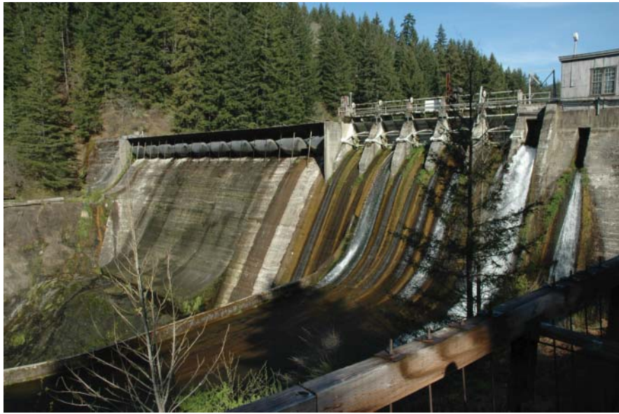
Figure 17.2 Condit Dam on the White Salmon River, Washington State, USA. This dam measured 38 m high and 144 m wide, and provided 80,000 MWh of power generation per year. The dam also resulted in the loss of 53 km of salmonid habitat. Breach of the dam occurred on October 26, 2011, and it was subsequently removed. (Photo by A. Yeakley.)
