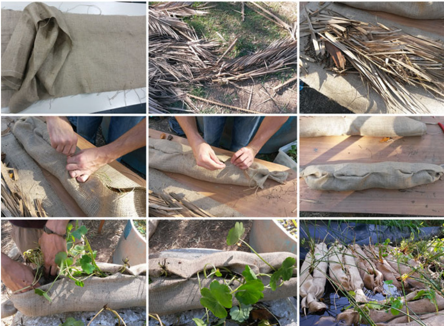
Fig. 2 Vegetated roll assembly sequence. Roll design: Sebastián Miguel
