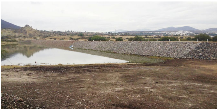
Fig. 9.19 La Lagartija Dam rehabilitated, January 2016 (Conagua SISP 2016)
