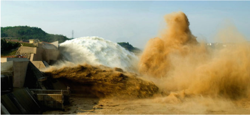
Fig. 6.3 Sediment flushing (by density currents) in Xiaolangdi dam, Yellow River ( source YRCC)
