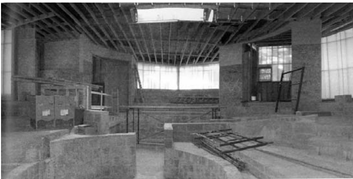
Figure 6. Bioscleave central room still under construction
