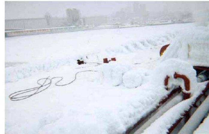
Figures 5.3F– Deck, piping and valves inaccessible
