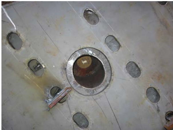
Figure 12: Access to the bow void docking plug
