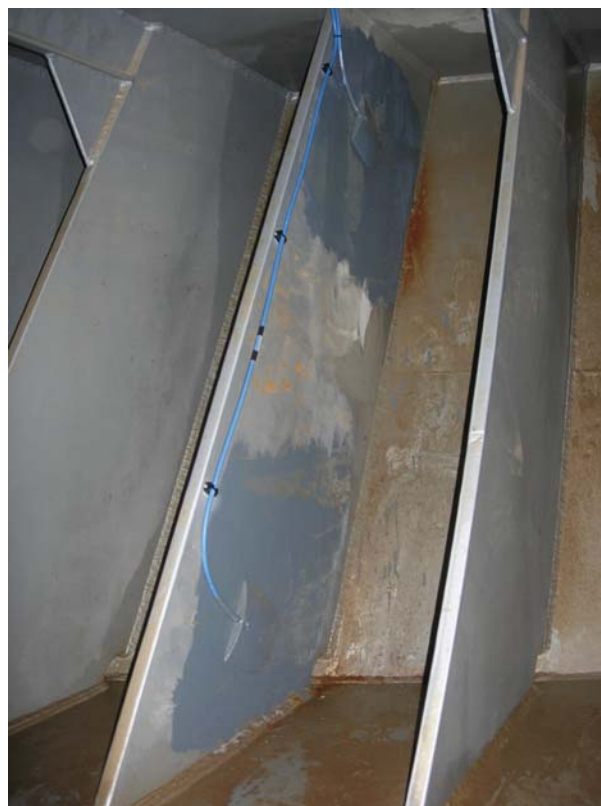
Figure 9: Mounting of fibre optical sensors
