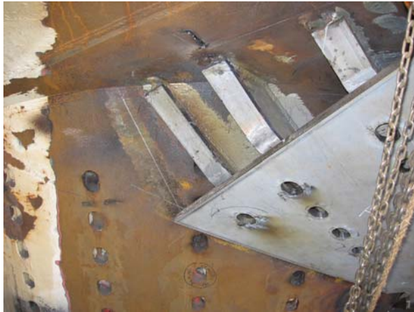
Figure 11: Snipe at the after intersection
