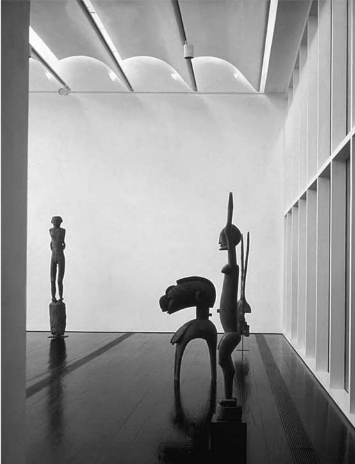
3.30 Museum for the Menil Collection. Composite structure of ferrocement and ductile iron.
