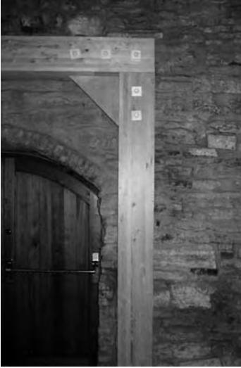
2.34 Rigid connection in a laminated wooden frame. Architect Sverre Fehn: Storhamarlåven (1976), Storhamar, Norway.
