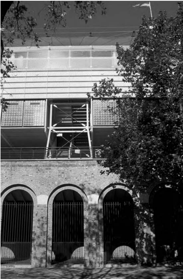
2.20 Architects Michael Hopkins and Partners: Mound Stand (1987), Lord's Cricket Ground, London.
