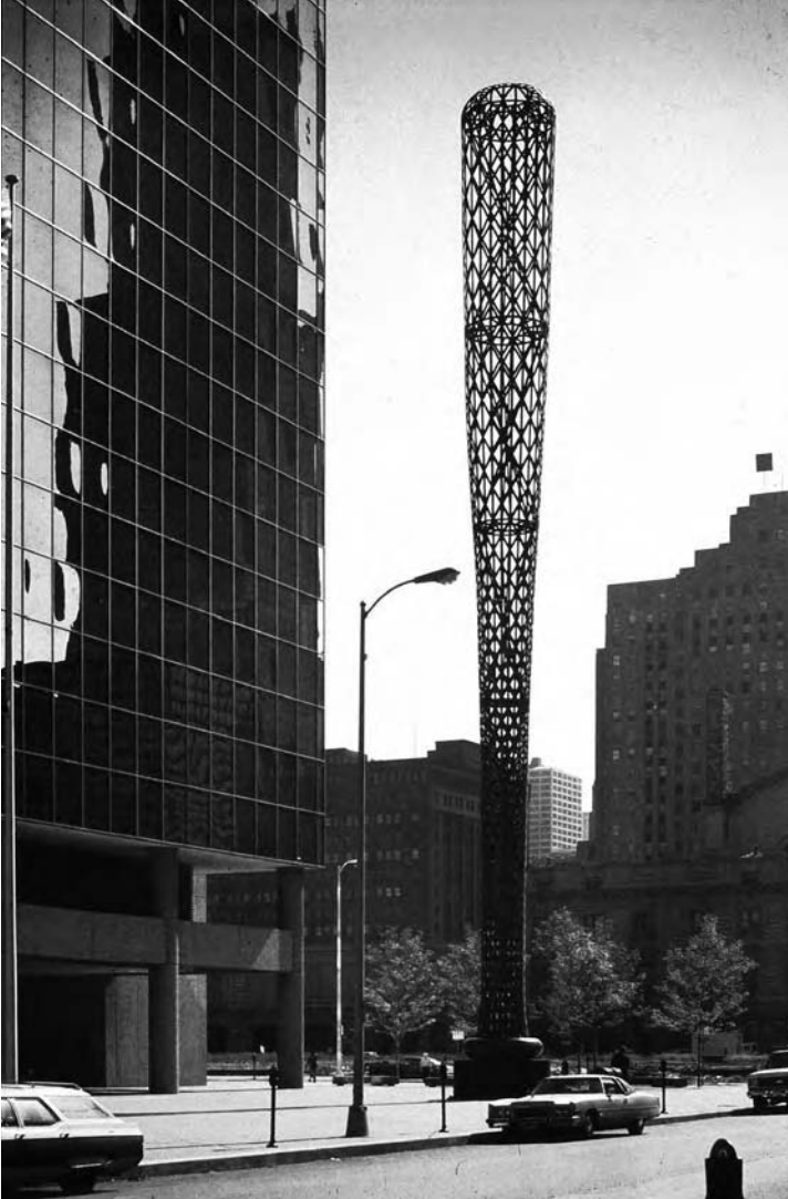
2.69 A dramatic increase in scale forces structural openness to replace solidity. The Bat Column (1977), Chicago. Height 29.5 m, diameter 3 m. Sculptors Claes Oldenburg and Coosje van Bruggen.
