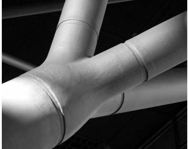
3.51 Stuttgart airport, Terminal 1. Detail of cast steel joint.
