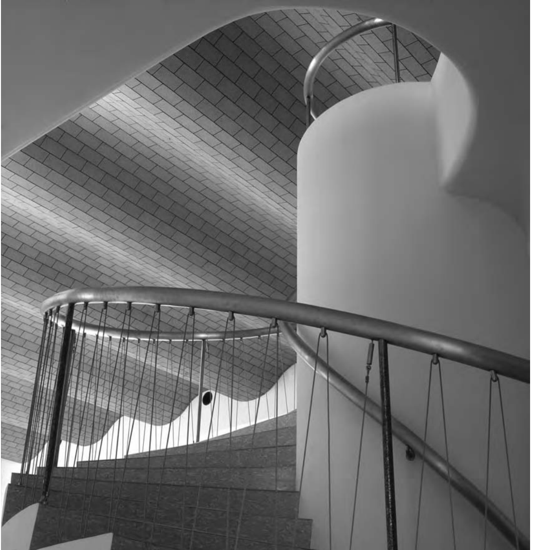
2.39 Stiffness through structural geometry. Architect Vilhelm Lauritzen: the roof structure of Copenhagen Airport Terminal Building (1939).
