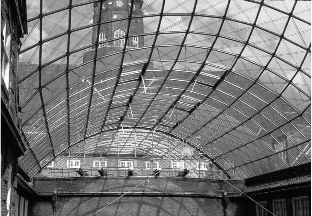
2.77 Museum of History (1989), Hamburg. Architects von Gerkan, Marg and Partners, engineers Schlaich, Bergemann and Partner.
