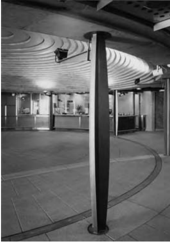
2.50 A tapered column. Architect Arne P. Eggen: National Theatre Underground Station (1998), Oslo.
