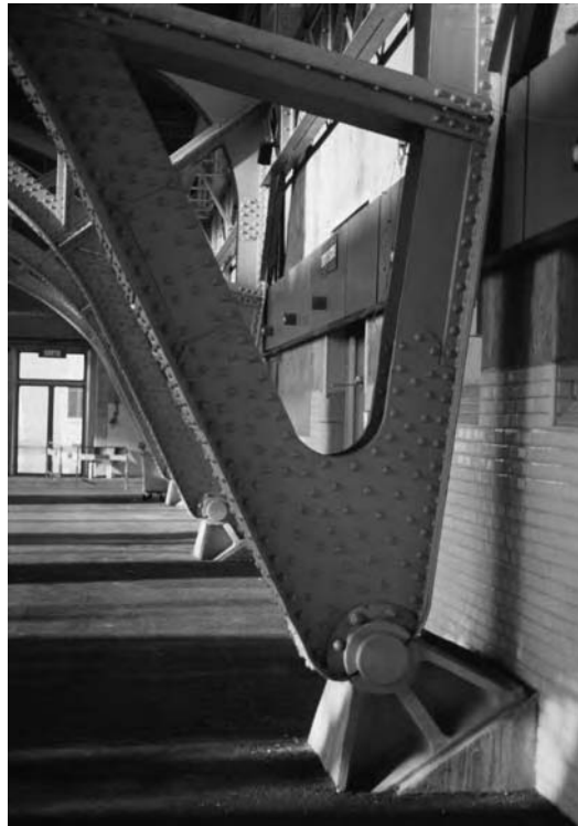
2.12 Global form: the three-hinged frame of the original slaughter-hall in Lyon (1914). Architect Tony Garnier.
