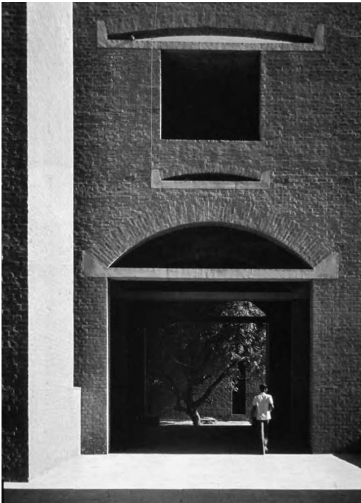
2.6 Dormitories. Architect Louis I. Kahn: Indian Institute of Management (1974), Ahmedabad, India.
