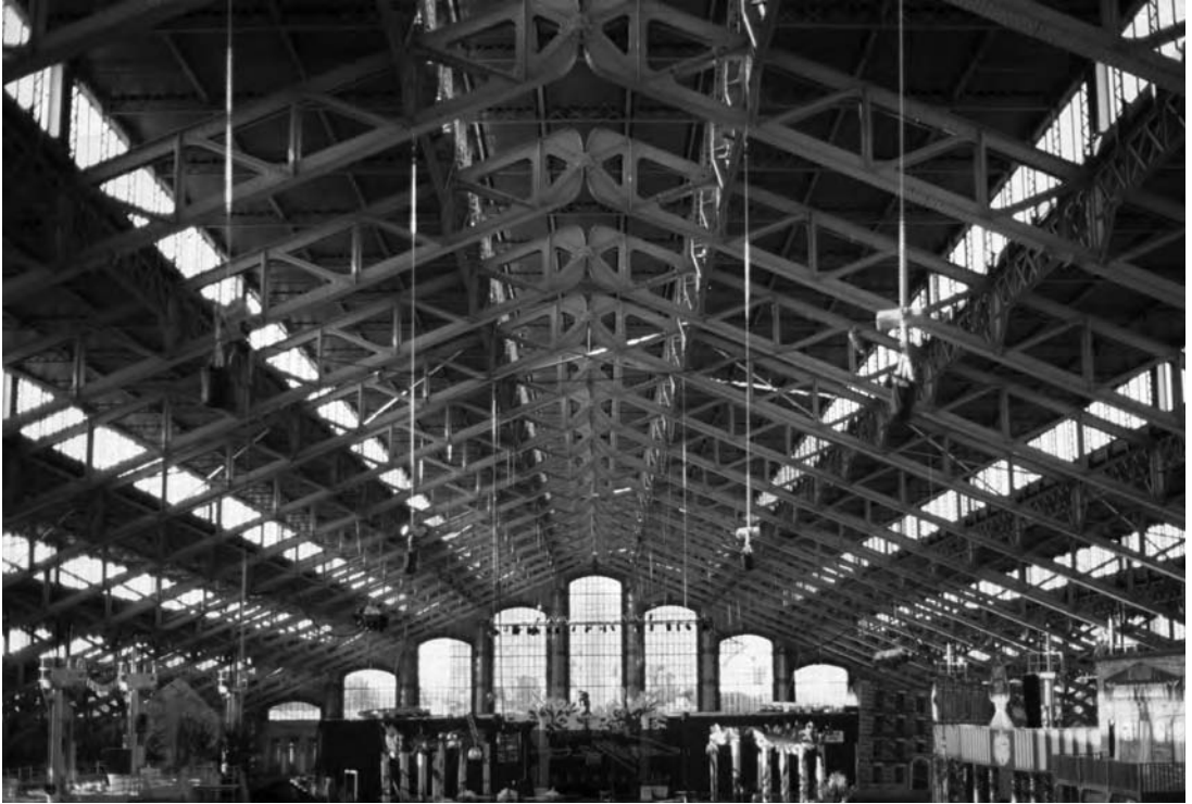
2.12 Global form: the three-hinged frame of the original slaughter-hall in Lyon (1914). Architect Tony Garnier.
