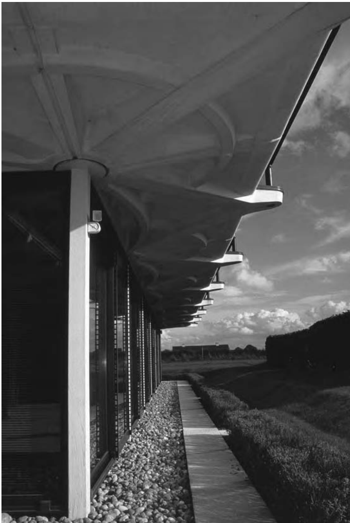
2.56 A more recent example of efficient distribution of concrete in a slab, inspired by Nervi. Architects Michael Hopkins and Partners: Schlumberger Cambridge Research Phase 2 (1992), Cambridge, UK.
