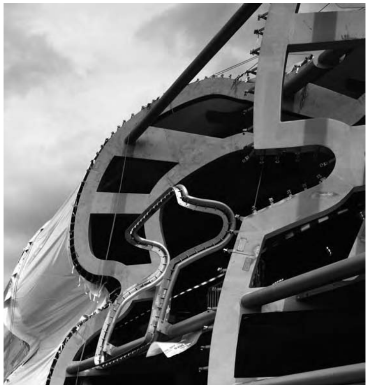
3.42 IAA pavilion 'Dynaform'. Detail of the structure.
