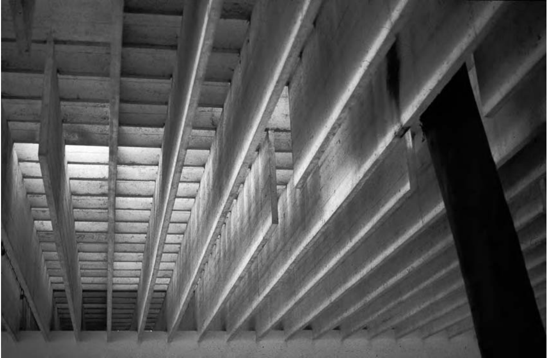
3.35 The Nordic Pavilion. Two-layered structure filters the light and allows trees to grow through the roof.
