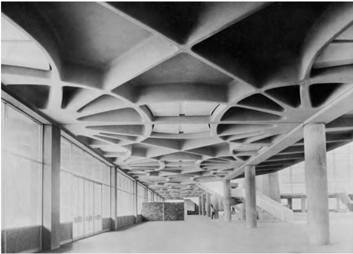
2.55 Isostatic slab structure. The ribs in the floor slab are arranged to follow the trajectories of the principal bending moments. Engineer Pier Luigi Nervi: the Palace of Labour (1961), Milan.
