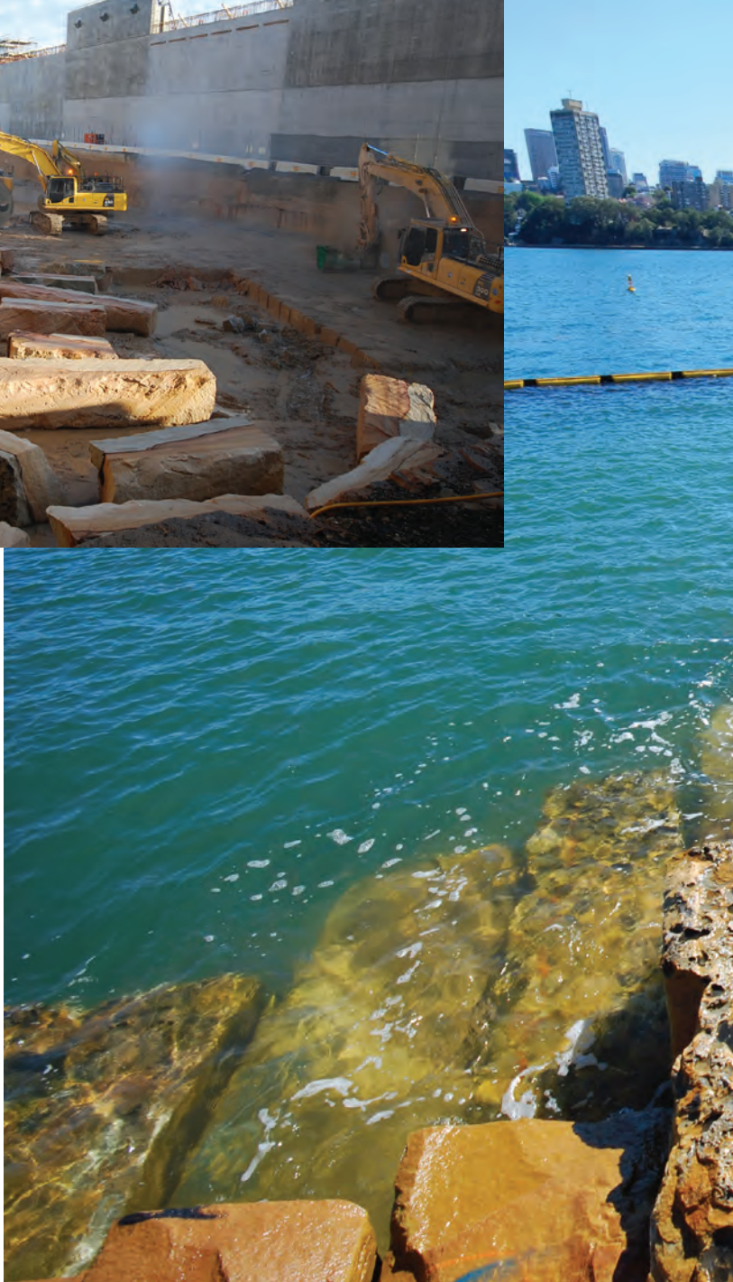
Figure 1-12 Barangaroo Headland Park Foreshore, cutting stone blocks from the onsite extraction hole.
