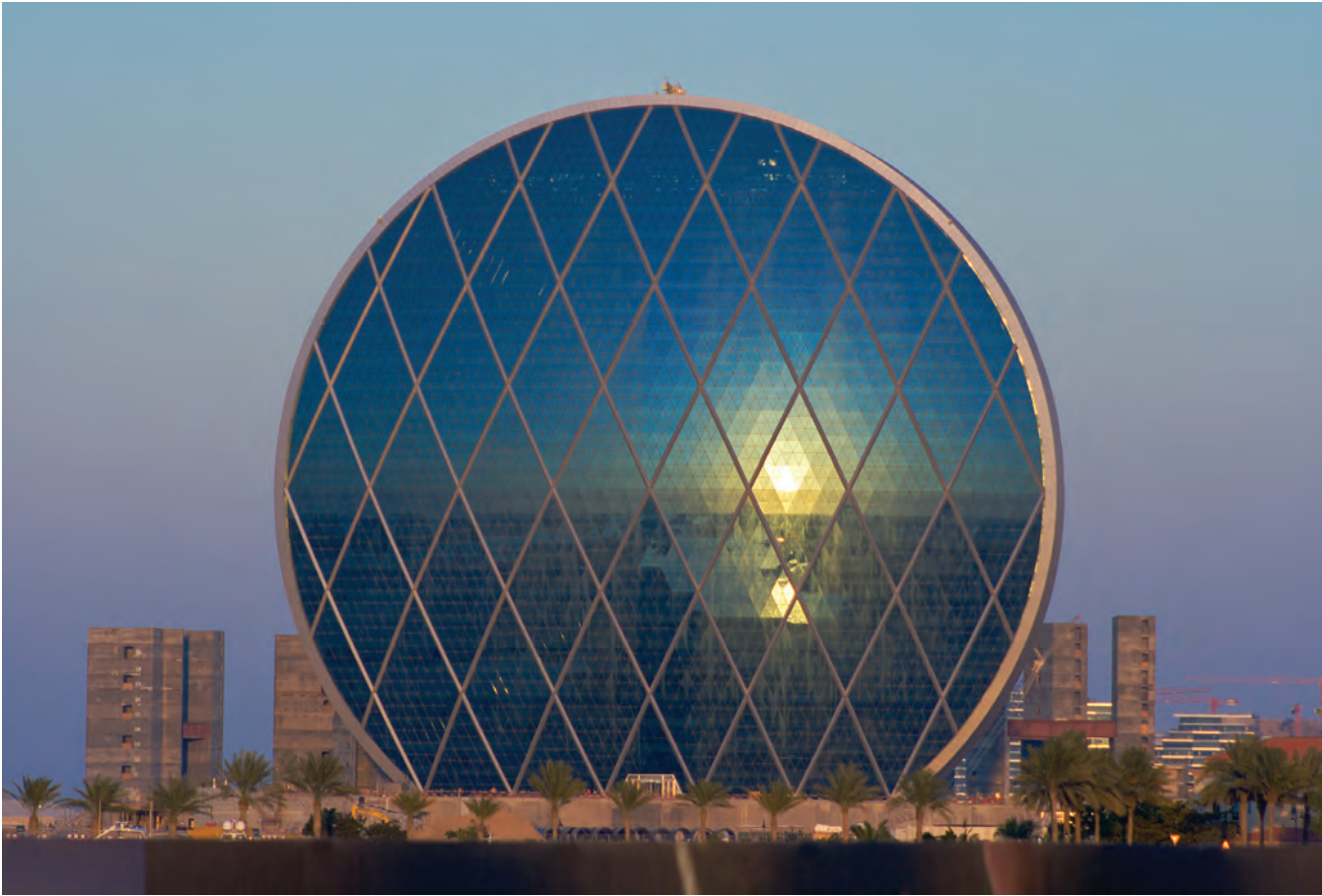
Figure 1-5 Arup, Aldar HQ Designer's impression and detailed construction model including steel and concrete detailing.
