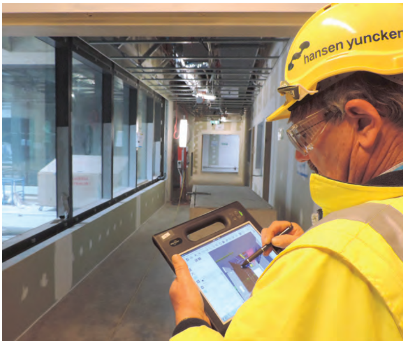
Figure 1-4 The new Royal Adelaide Hospital Field BIM used by the Hansen Yuncken Leighton Contractors Joint Venture.
