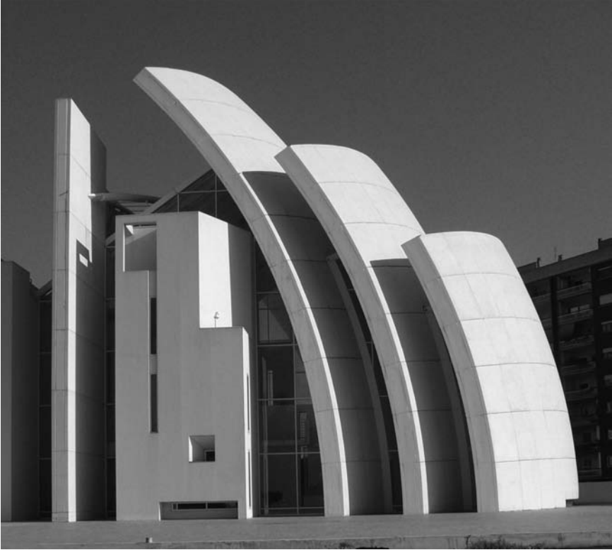
Figure 2.4 The facade of Dives in Misericordia in Rome, built in 2003, consists of 256 precast, self-cleaning concrete sections assembled into 25-metre high curved white sails (source: photo courtesy of Claudio La Rosa, Rome (Flickr – axez02)).
