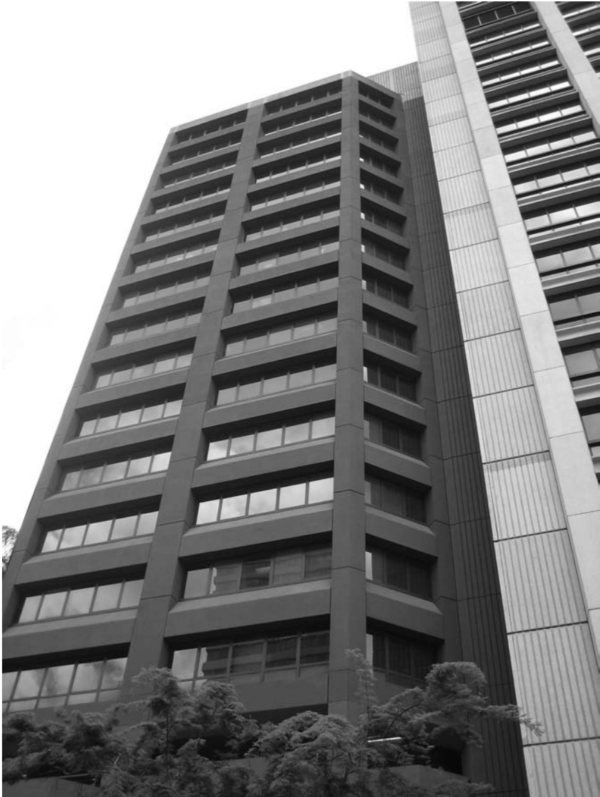
Figure 14.7 Facade of one of the existing buildings in the test location.
