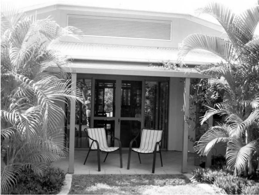
Figure 13.3 Research House's passive cooling techniques, with good cross-ventilation and well-ventilated roof space.
