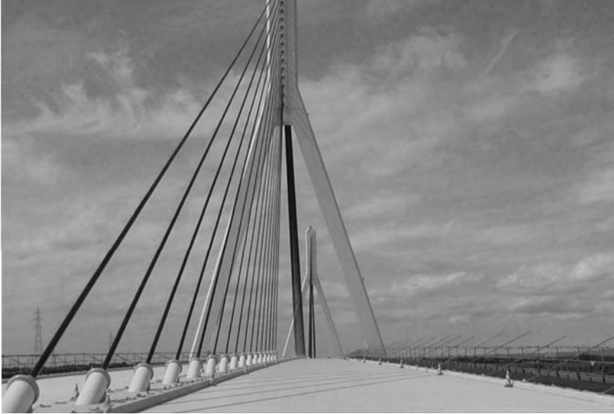
Figure 2.1b Cable-stayed Mihara Bridge in Hokkaido, opened in 2005 with an ECC on steel deck. The ECC stiffens the jointless deck and decreases stress, resulting in a 40 per cent weight reduction and a 50 per cent cost reduction (source: photo courtesy of Kajima Corporation and Kuraray Co. Ltd).
