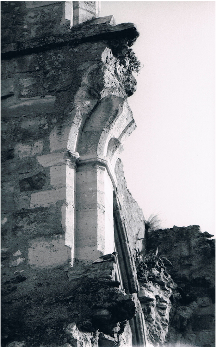
Figure 8 Le Lys, south side of nave, springing of triforium arches, ca. 1248 (Photo: A. Gajewski).
