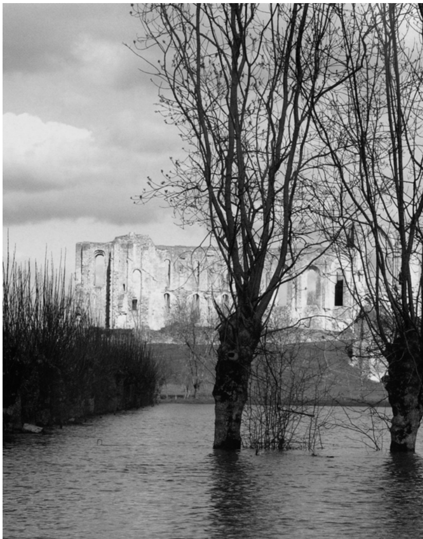
Figure 1 Maillezais Abbey, western end and remains of south facade, ca. 1080. View from the canal to the south (Photo: M. Abel).
