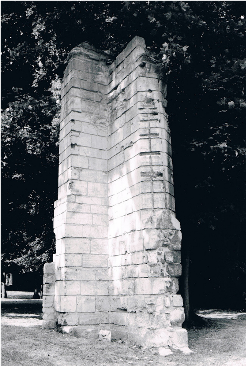
Figure 9 Maubuisson, south transept chapel, south eastern corner, ca. 1244 (Photo: A. Gajewski).
