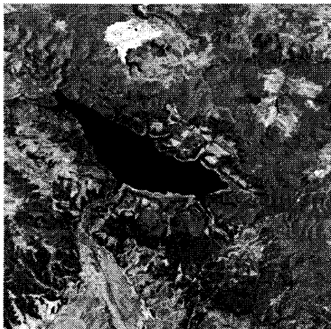
Figure 5. Space image of Iskar Dam
