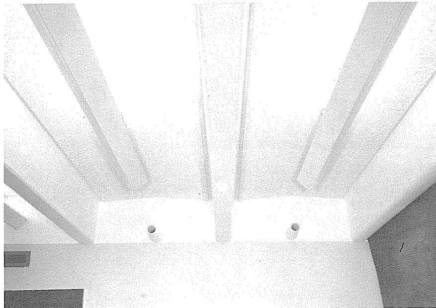
3 Mock-up of indirect lighting scheme.
