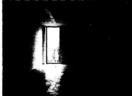
Fig. 43: Positioning the window in the corner leads to different lighting effects. Diener + Diener: Pasquart Centre (museum), Biel (CH), 1999
