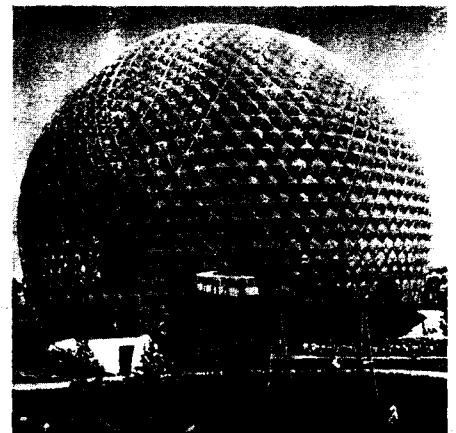
Fig. 71: The truncated sphere has a base diameter of 110 m. Buckminster Fuller: USA Pavilion, EXPO 67, Montreal (CAN), 1967
