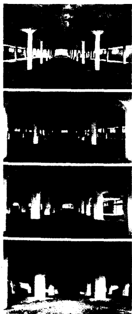
Fig. 1: Flared-head columns in reinforced concrete (diameter varies with storey, or rather load) Robert Maillart: gran warehouse, Altdorf (CH), 1912
