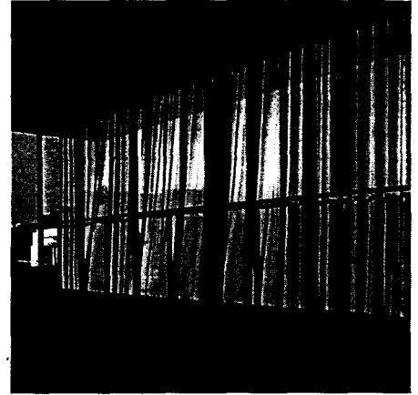
Fig. 87: Curtains for preventing glare and for partial exclusion of the surroundings Ludwig Mies van der Rohe: New National Gallery, Berlin (D), 1968
