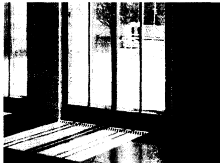
Fig. 17: Underfloor heating plus hot-air ducts supplied from the cellar (in front of French windows) Ludwig Wittgenstein: house in Kundmangasse, Vienna (A), 1928
