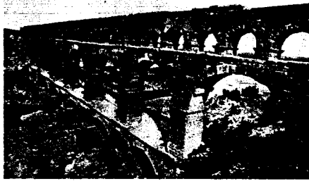
Fig. 36: Succession of stacked arches: sectional concept in order to omit superfluous material. The arch construction is sensible from an engineering and an economic viewpoint. Pont du Gard, Roman aqueduct at Nîmes (F), 1st century AD
