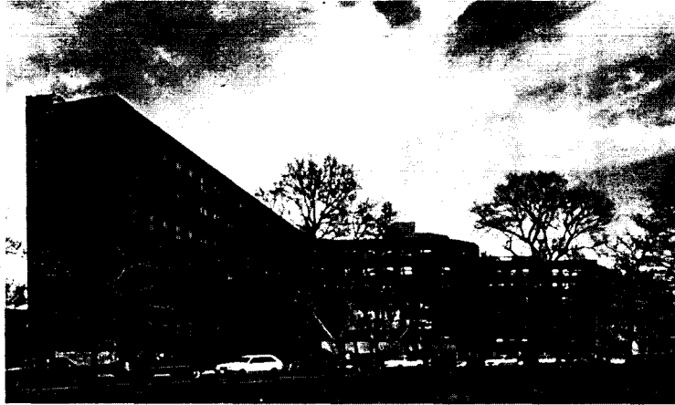
Fig. 25: Organic form making use of the identical, smallest "cell" Alvar Aalto: Baker House, Massachusetts Institute of Technology, Cambridge (USA), 1954
