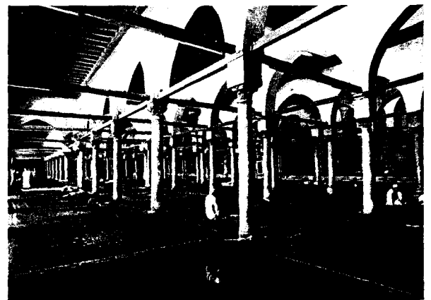
Fig. 110: ... while the prayer hall appears to be less directional owing to the transverse beams. El-Azhar Mosque, Cairo (Egypt), c. 970
