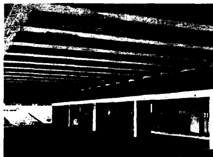
Fig. 62: Basement garage, c. 1960 Ribbed slab
