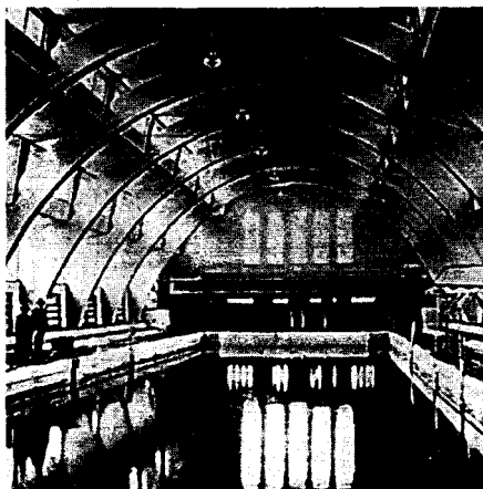
Abb. 56: Fixed-based arch Stuttgart Building Department (F. Fischle, F. Cloos); swimming pool, Heselach (D), 1929
