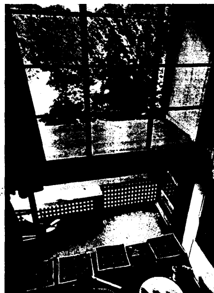
Fig. 76: Fixed sunshade as a tangible intermediate layer with brise-soleil (top) and loggia Le Corbusier: Unité d'habitation, Marseille (F), 1947
