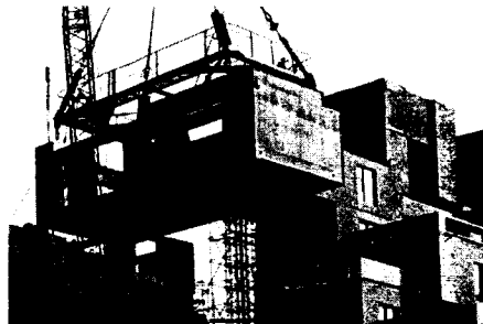
Fig. 135: The units are erected as "structural shells" without any roof. Moshe Safdie: HABITAT 67, Montreal (CAN), 1966-67
