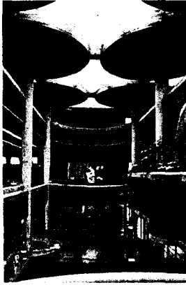
Fig. 2: The roof as a "baldachin" Frank Lloyd Wright: office building for Johnson Wax company, Racine (USA), 1940–50
