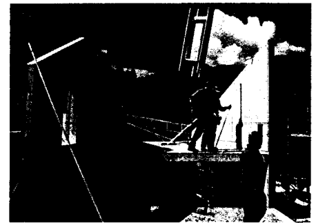
Fig. 298: Assembling the wall and floor elements The floor elements are suspended between the walls on Z-sections.
