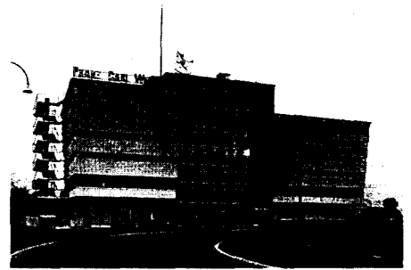
Fig. 124: Facade using Durisol system Rudolf Kuhn and Heinz Ronner: FCW warehouse, Zurich (CH), 1954–55
