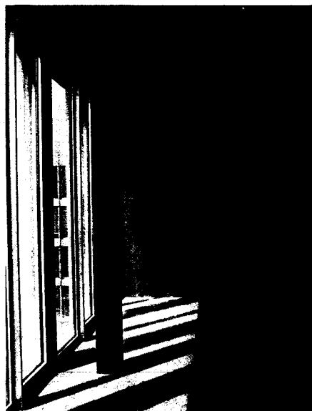
Fig. 216: Column and wall Access zone in secondary school, fair-face concrete wall with formwork type 2 and precast concrete column
