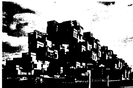
Fig. 133: Stacking of concrete room units ("heavyweight prefabrication") Moshe Safdie: HABITAT 67, Montreal (CAN), 1966-67
