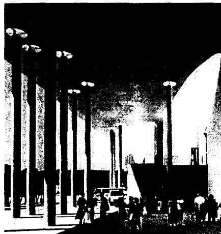
Abb. 54: Spun-concrete columns, connected to reinforced concrete roof via steel web plates. Axel Schultes: art gallery, Bonn (D), 1992
