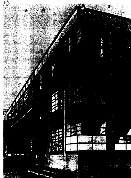
Fig. 8: The first curtain wall in Europe wraps around the corners to enclose the whole building. Walter Gropius: Fagus factory, Alfeld a. d. Leine (D), 1911–25; view from south-east, condition after 1914
