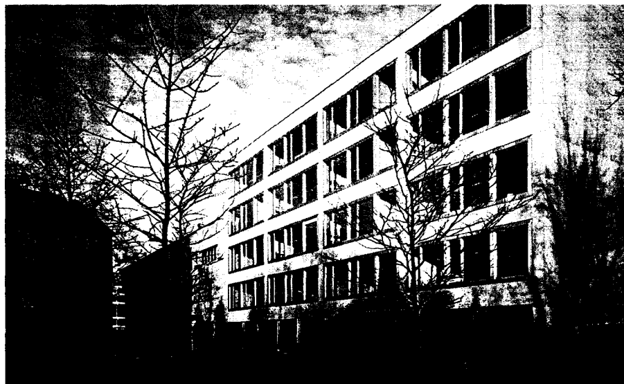
Fig. 153: Entrance elevation fronting the open area
