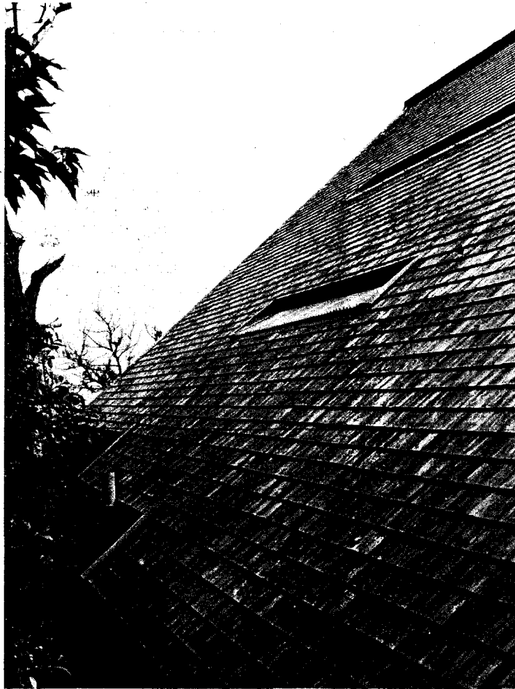
Fig. 63: Roof covering of wooden shingles Shin Takasuga: "Railway Sleeper House", Miyakejima (J), 1980
