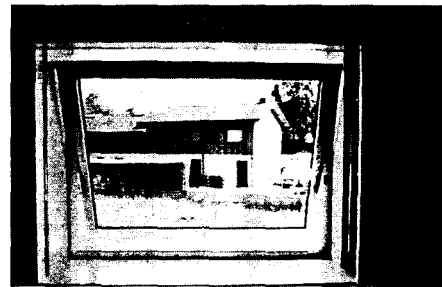
Fig. 122: Horizontal pivot window from inside
