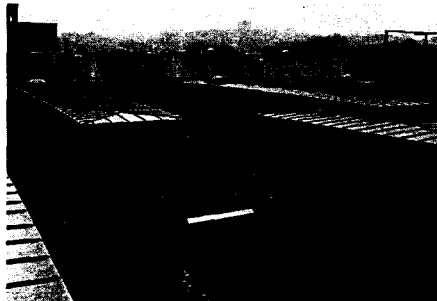
Fig. 62: The lantern lights (clad with patterned glass) span from wall to wall. Herzog & de Meuron: locomotive depot "Auf dem Wolf", Basel (CH), 1995
