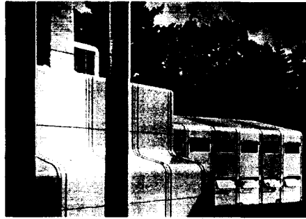
Fig. 131: Plastic walls and roof James Stirling: Olivetti training centre, Haslemere (GB), 1969
