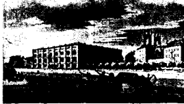
Fig. 75: Reduction of the structure Karl Friedrich Schinkel: Academy of Architecture (destroyed), Berlin (D), 1836
