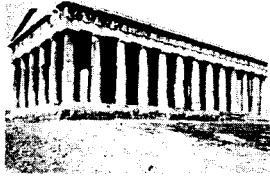
Fig. 55: The plinth as a platform to prepare the site Greek temple, c. 500 BC
