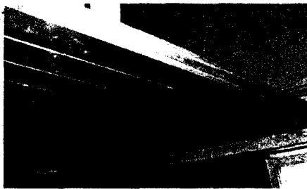
Fig. 8: Staggered positioning of solid timber elements
