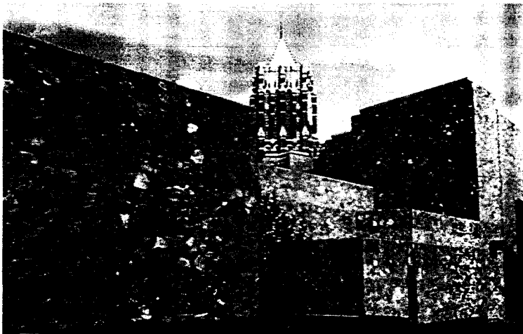
Fig. 23: Unconventional masonry Eero Saarinen: Ezra Stiles College and Morse College, Yale University (USA), 1960
