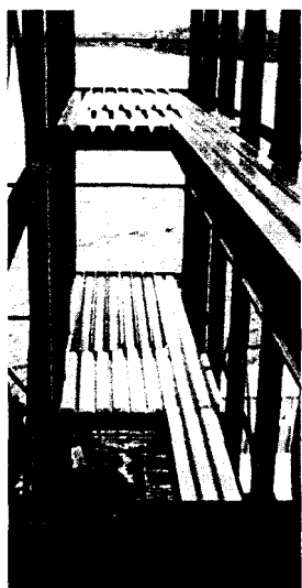
Fig. 37: Composite floor construction Profiled metal sheeting prior to concreting
