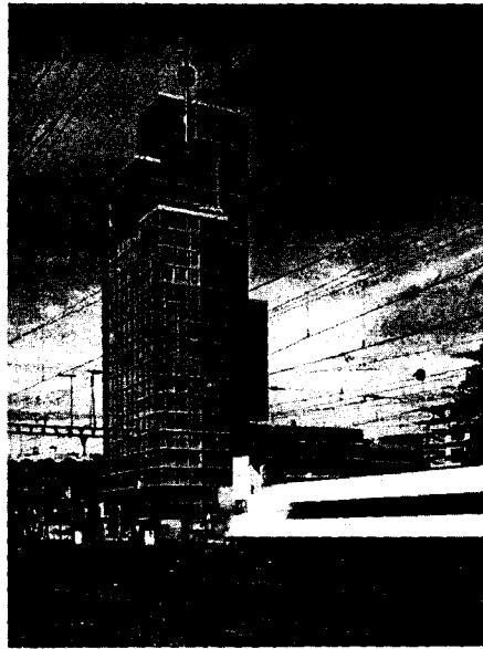
Fig. 58: On the facade the floor slab edges are the only visible part of the loadbearing structure. Burkard, Meyer Architekten: Swisscom headquarters, Winterthur (CH), 1999
