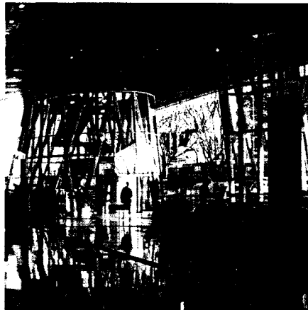
Fig. 72b: The corner columns house the stairs. Toyo Ito: Mediothek, Sendai (J), 2001
