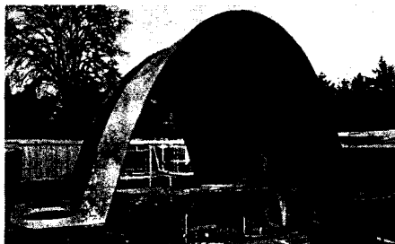
Abb. 69: Shell designed with perfect form (parabola), shell thickness approx. 6 cm. Robert Maillart: Cement Industry Pavilion for Swiss National Exhibition, 1939
