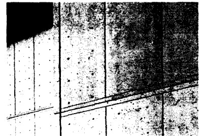
Fig. 26: Vertical panel formwork, panels coated with synthetic resin lacquer Louis I. Kahn: Salk Institute, La Jolla (Cal, USA), 1959–65
