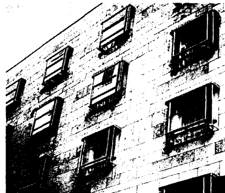
Fig. 34: Cantilevering glass oriels enable good views of the street below. Alejandro de La Sota: Calle Prior apartment block, Salamanca (E), 1963
