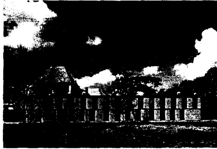
Fig. 127: Storey-high clay elements with loadbearing and insulating functions; (left) erection of loadbearing structure at ground floor level, (above) finished building Tectone: hotel training school, Nivilliers (F), 1999
