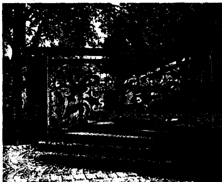
Fig. 52: Bent sheet steel ( d = 12 \text{ mm} ) as a structural element (above); plan, scale approx. 1:140 (left) Hild und K: bus shelter, Landshut (D), 1999
