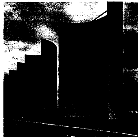
Fig. 34: Concrete half-cylinders 25 m high ( d = 25 cm); the tie bars at the top guarantee the stability of the form. Maarten Struijs: windbreak in Rotterdam Harbour (NL), 1985
