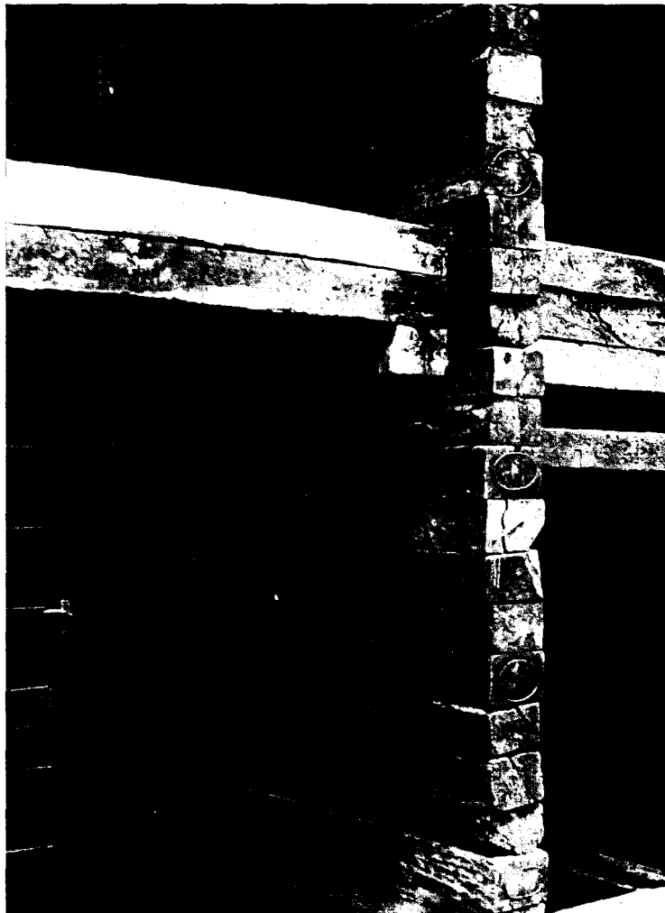
Fig. 66: Detail of jointing at projecting stack of sleepers on the entrance facade Shin Takasuga: "Railway Sleeper House", Miyakejima (J), 1980
