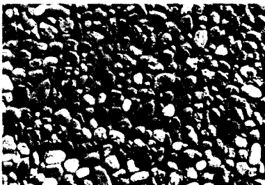
Fig. 27: Concrete with exposed aggregate finish Aggregate revealed by jetting
