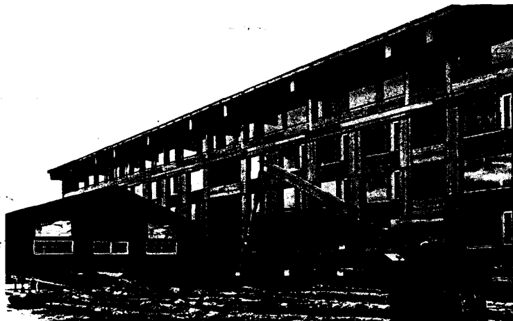
Figs 256 and 257: The Swiss School of Engineering for the Wood Industry is a series of wooden boxes.
