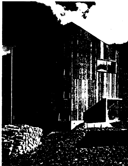
Fig. 303: West facade The linear arrangement of the windows identifies the position of the "static" rooms.
