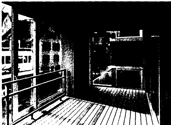
Fig. 62: Veranda Unheated intermediate zone acts as extension to living room and also as balcony.
