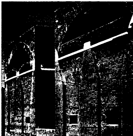
Fig. 38: The reinforced concrete tie accommodates the thrust and relieves the wall below. Louis I. Kahn: Indian Institute of Management, Ahmedabad (India), 1962-74
