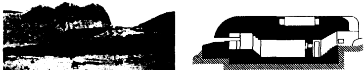
Fig. 51: Bunker in French Atlantic Wall "buried" in the sand (left), longitudinal section (right)
