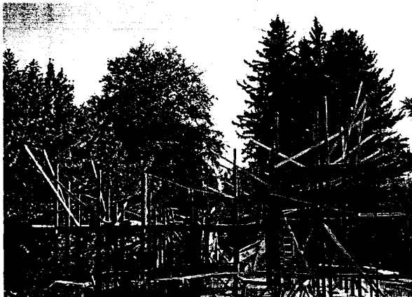
1 Horizontal wooden templates positioned and fixed with the help of a scaffold
