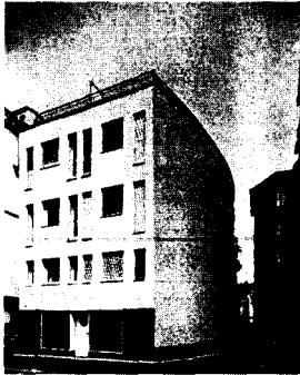
Fig. 66: Rendered thermal insulation with stone plinth Dolf Schnebli: apartment block, Baden (CH), 1990
