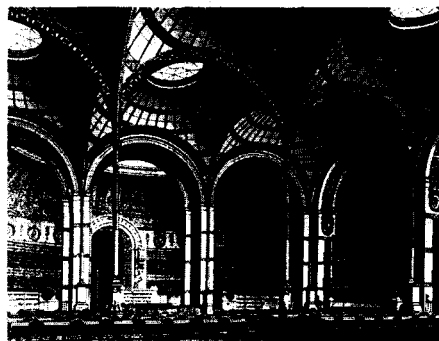
Fig. 4: Translation of a stone structure into cast iron Henri Labrouste: Bibliothèque Nationale, Paris (F), 1875
