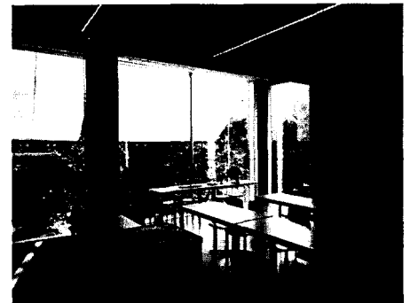
Fig. 241: Seminar room Views of the outside are still possible even when the awnings are extended.
