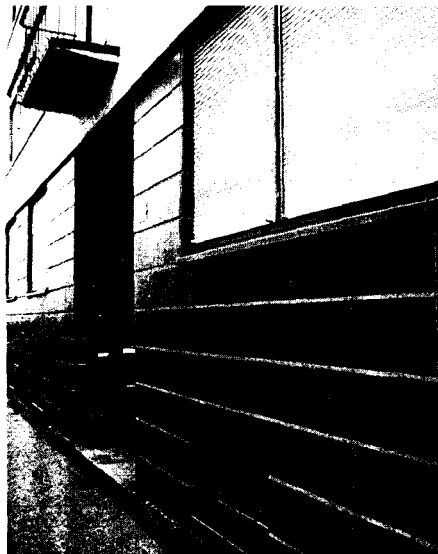
Fig. 67: Painted concrete and ceramic tiles as protection against weather and soiling, and also providing a figurative plinth function Otto Rudolf Salvisberg: apartment block, Zurich (CH), 1936
