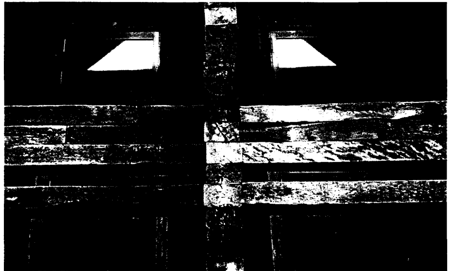
Fig. 76: Sleepers inserted into and cantilevering from the projecting stack provide stability Shin Takasuga: "Railway Sleeper House", Miyakejima (J), 1980
