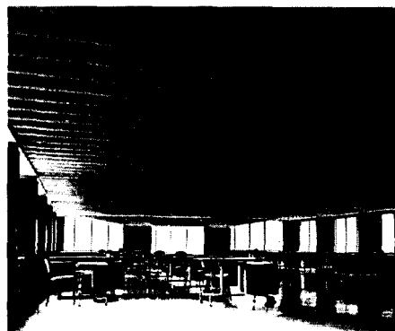
Fig. 9: Gaibani office building Milan (I), 1955/56 Reinforced concrete floor by Pier Luigi Nervi Design: E. Soncini, A. Pestalozzo
