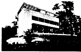
Fig. 9: The loadbearing steel structure disappears behind the render. Wassili and Hans Luckhardt: house on Rupenhorn, Berlin (D), 1928
