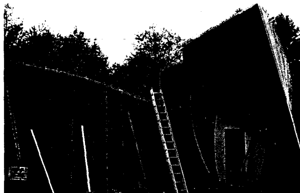
4 Cut-out for large entrance opening (note the difference between this and photo 3). Edges reinforced with additional bars.
