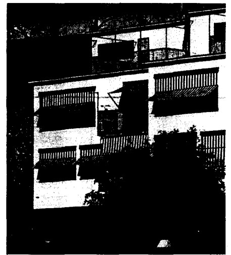
Fig. 83: Semi-awnings to the windows, straight-arm awnings and vertical blinds to the balconies Max Ernst Haeleli: Rotach development, Zurich (CH), 1928
