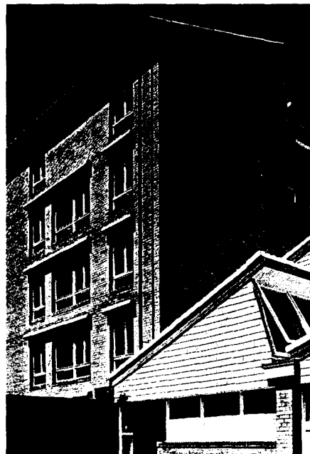
Fig. 86: Surface-mounted roller shutter boxes as a design element on the facade Ernst Gisel: housing and studios, Zurich (CH), 1953
