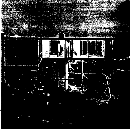
Fig. 111: The steel structure is a visible form criterion ("lattice structure"). Craig Ellwood: Smith House, Los Angeles (USA), 1957–58
