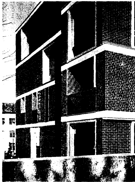
Fig. 4: Flexibility in planning: the position of the windows was determined by the buyers of the apartments. Burkard Meyer: apartment blocks, Martinsbergstrasse, Baden (CH), 1998/99
