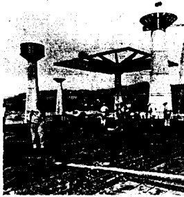
Fig. 76a: Canopies under construction Pier Luigi Nervi: Hall of Labour, Turin (I), 1961
