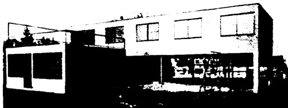
Fig. 114: All traces of the structure are concealed behind masonry panels and render. Artaria & Schmidt: Schaeffer House, Riehen (CH), 1927–28
