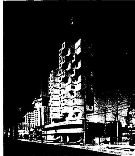
Fig. 106: External view; the taller staircase tower is clearly visible. Kisho Kurokawa: Nakagin Capsule Tower, Tokyo (Japan), 1972
