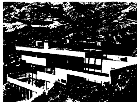
Fig. 8: The steel columns are hardly distinguishable from the window frames. Richard Neutra: Lovell Health House, Los Angeles (USA), 1927–29
