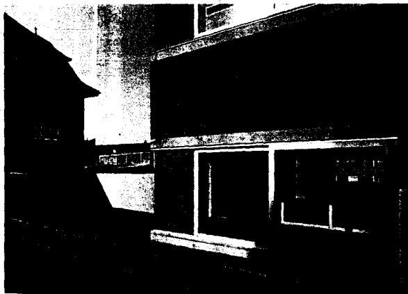
Fig. 61: Ground floor veranda The sliding doors opening onto the veranda lend depth to the facade.
