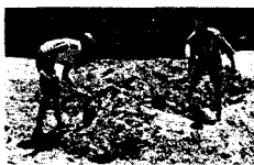
Fig. 2: Earth Mixing with cob and sand
