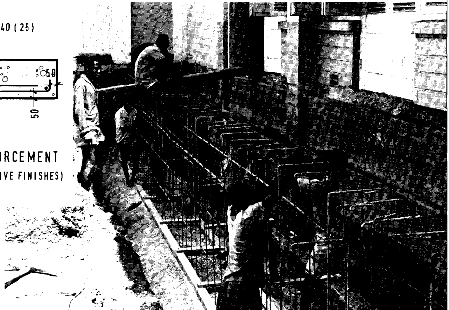
Fig. 186: Vertical stirrup irons in the new foundation wall at the Parliament House extensions.
