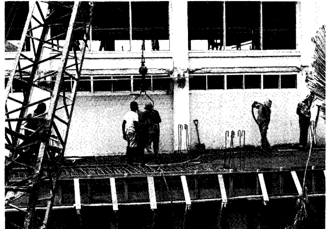
Fig. 180: Concreting dense concrete with a vibrator. First floor slab of the Members' Lobbies at the Parliament House extensions in Accra. Architect: HANNAH SCHRECKENBACH, 1970/71.
