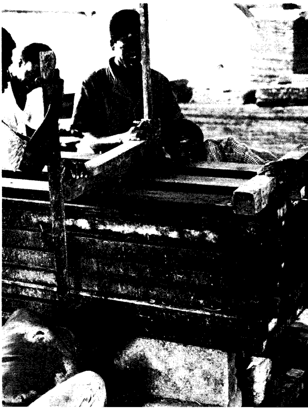
Fig. 205: Using a clamp to press down ready-mixed woodwool shavings in moulds.
