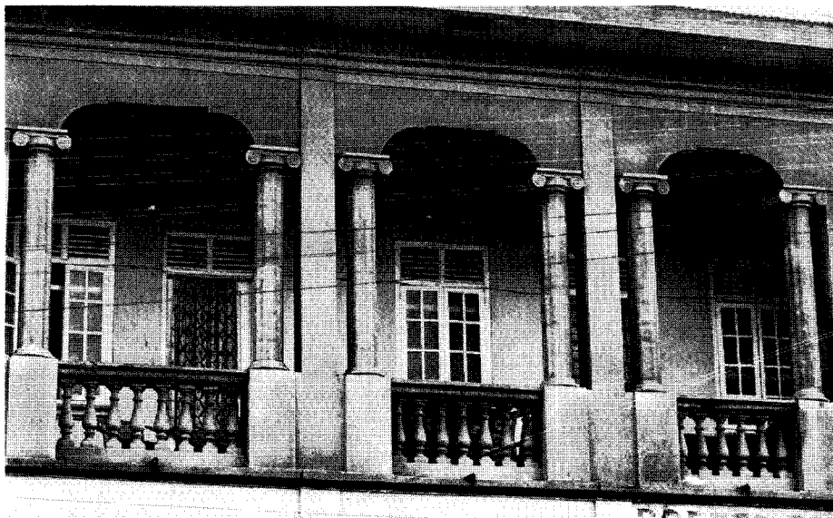
PART OF THE KING'S GUEST-HOUSE IN KUMASI AFTER R. A. FREEMAN FROM HIS BOOK "TRAVELS AND LIFE IN ASHANTI AND JAMAN" (1898). THE LOWER PORTION OF THE WALL WAS FINISHED IN POLISHED RED CLAY. THE FRIEZES OF THE UPPER WALL PANEL, THE FLAT PILASTERS ON BOTH SIDES OF IT AND THE UN-DECORATED GABLE PANEL WERE FINISHED WITH LIME WASH.
