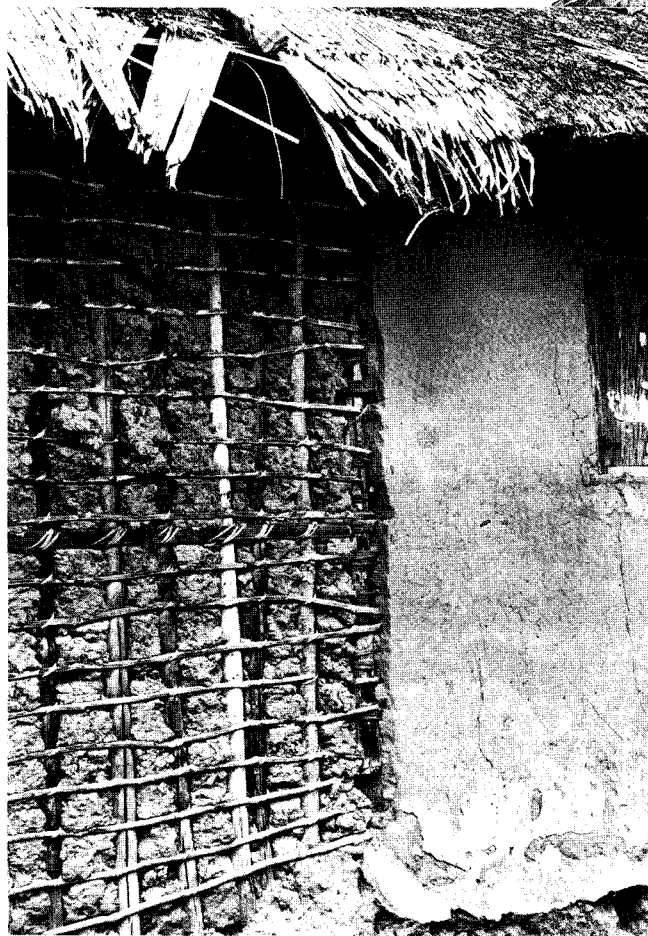
FIG. 92 : WATTLE AND DAUB WALLS IN AN ASHANTI FOREST VILLAGE ( ABOVE AND ABOVE RIGHT ), 1981.
