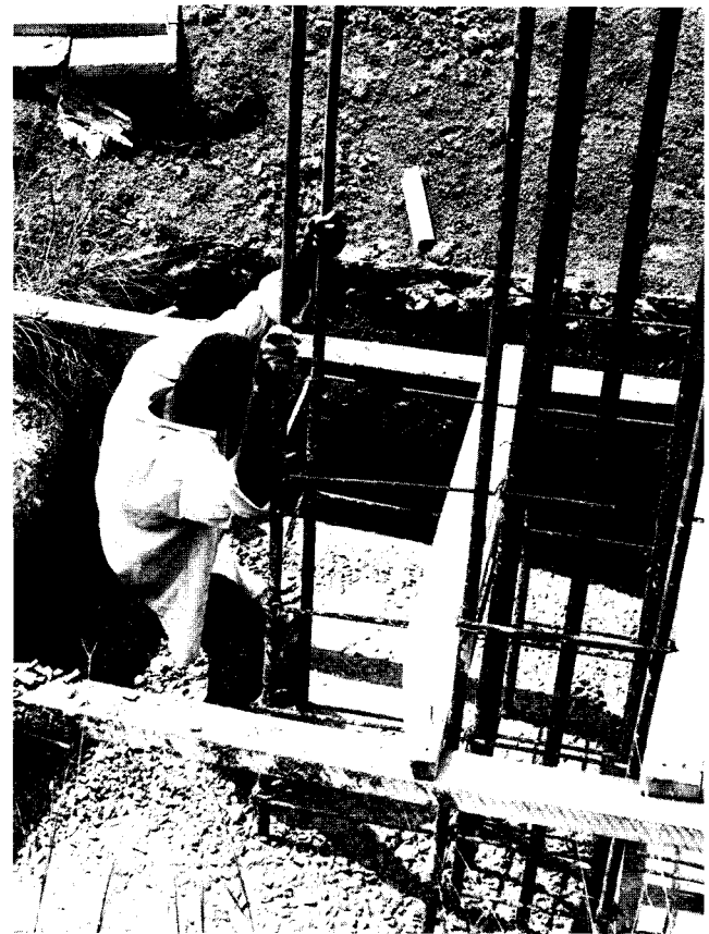
Fig. 256: The completed pad foundation with starter bars for vertical column reinforcement, 1981.
