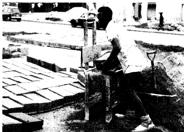
Fig. 289: A 350 × 230 × 150 mm block has been pressed. The block maker will turn the handle down to lift the block up.
