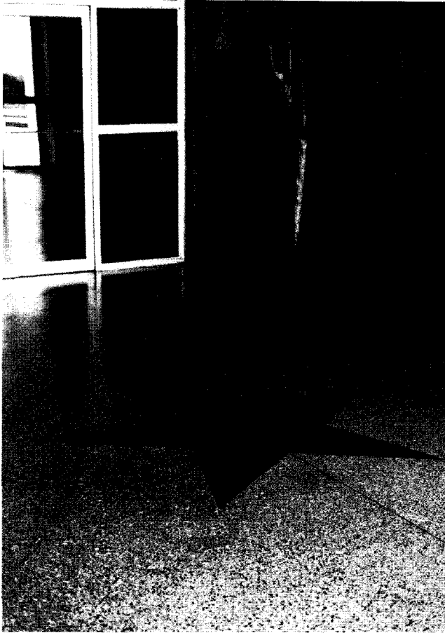
Fig. 272: The in situ terrazzo floor in the entrance hall of Parliament House, Accra, 1971. Architect: HANNAH SCHRECKENBACH.
