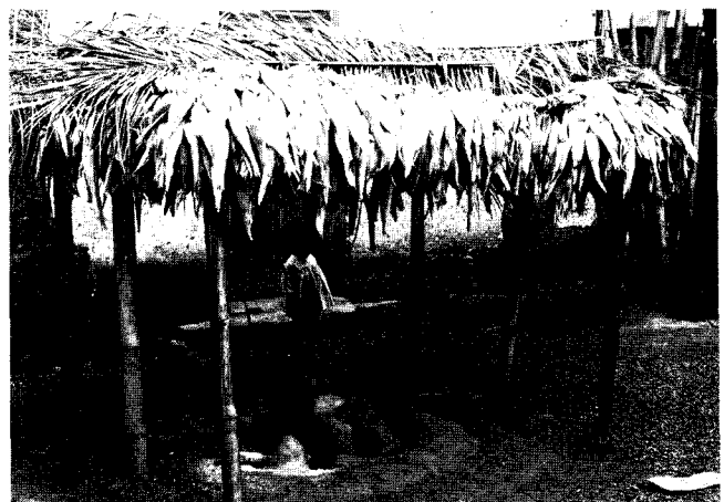
Fig. 55: Bamboo shelter in Kuntanase, Ashanti Region, over an outdoor cooking area, serving also as corn storage, 1979.
