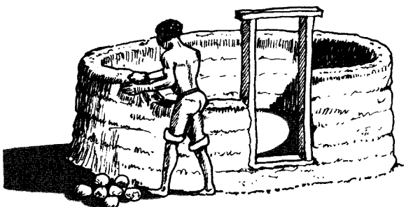
CONSTRUCTION OF WALL WITH DOOR FRAME
