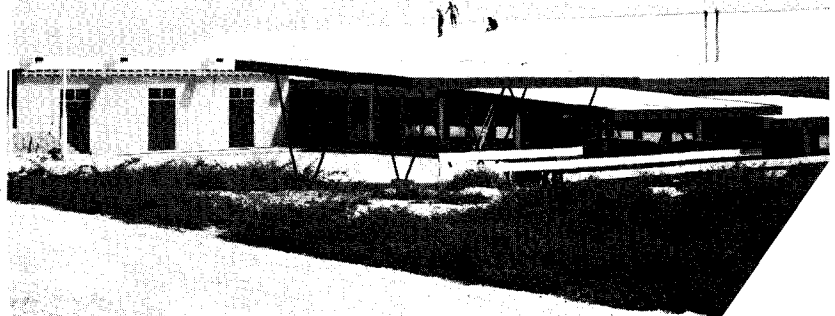
FIG. 347 a : CORRUGATED ASBESTOS - CEMENT ROOF
