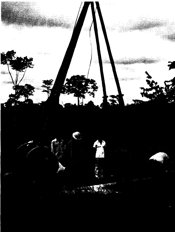
Fig. 244: Soil tests with the B.R.R.I. drilling rig at the Faculty of Engineering, School of Mining Engineering site, U.S.T., 1982.
