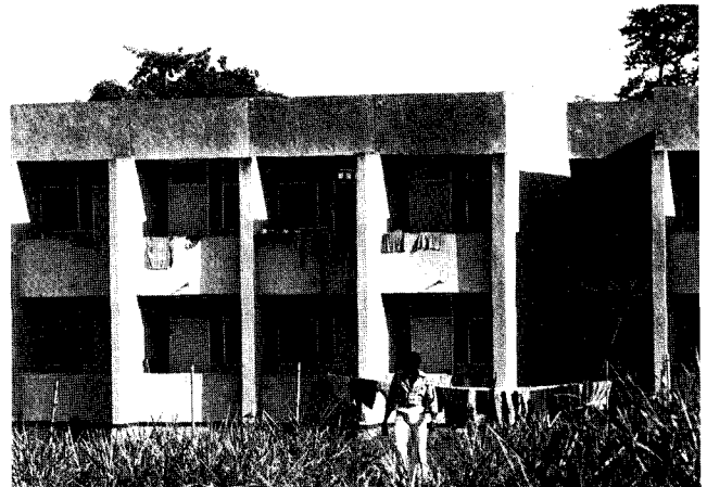
Fig. 283: Students' Hostel, U.S.T., Kumasi with TEK-block walls, 1982. Department of Housing and Planning Research, U.S.T.
