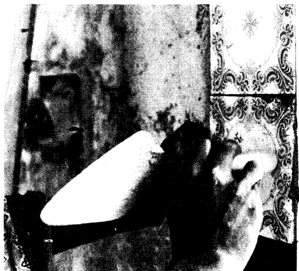
Fig. 302: Fixing of glazed wall tiles, Kumawu, 1982.
