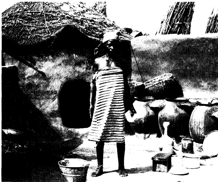
Fig. 17: Ventilation opening under the thatched roof of a kitchen in a Kusasi compound at Zebila, 1968.
