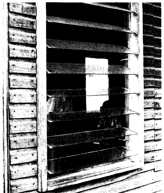
WINDOW 9 : ELEVATION FROM THE OUTSIDE IN CLOSED POSITION NACO LOUVRE WINDOW WITH 9 BLADES, 150 mm WIDE, CLEAR GLASS, WITH MOSQUITO GAUZE AND BURGLAR PROOFING AS PART OF THE FRAME, WITH NACO LOUVRE CARRIERS AND ALUMINIUM WEATHER STRIP.
