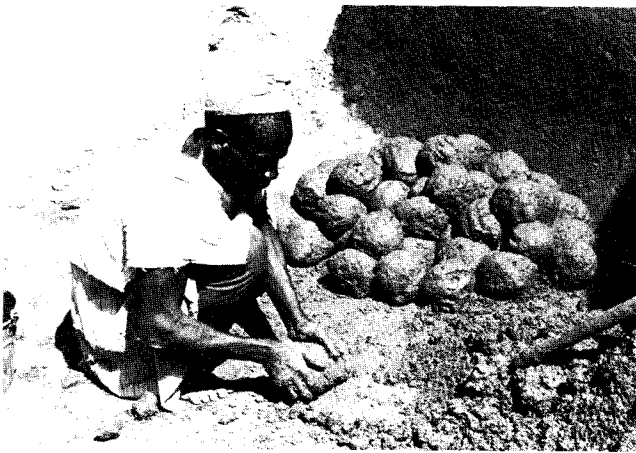
Fig. 12: A Talensi farmer moulding mud balls for house construction. In the background is part of a completed wall, 1976.
