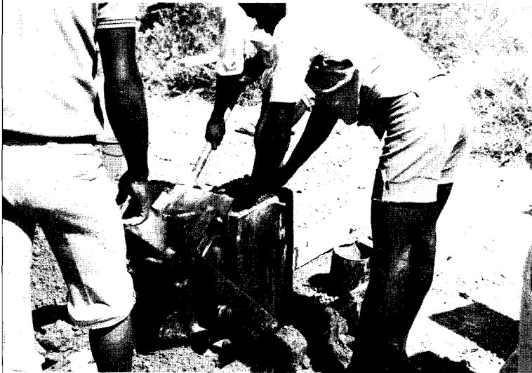
Fig. 132: Blockmaking with the TEK-Block Press, 1979: Filling the mould;
