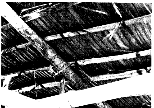
Fig. 157: Detail of a roof covered with Raphia palm leaf tiles, shown from underneath.
