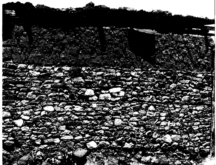
Fig. 114: A stone and mud wall house in Akropong, 1981 (Photograph by G. OWUSU).
