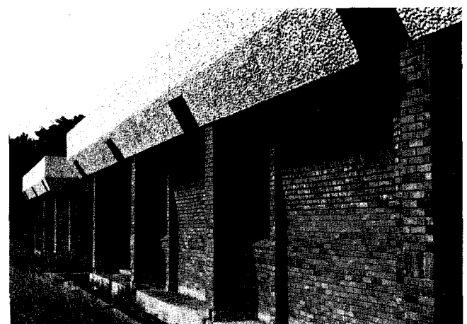
Fig. 282: External fairfaced brick wall, C.S.I.R. Library building (under construction), Accra, 1982. Architects: V. MAHADEVAN (Head, Consultancy & Development Division, B.R.R.I., Kumasi).
