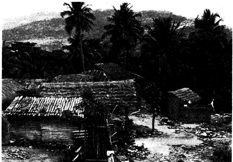
Fig. 70: Roofscape of Aviefe. Note the bamboo roof in the foreground.
