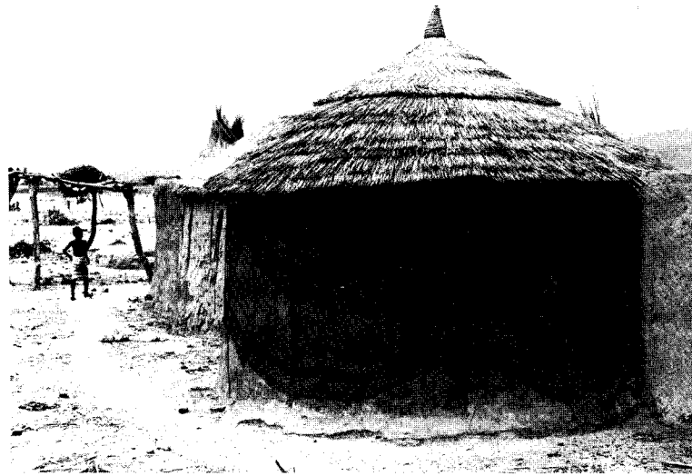
Fig. 22: A fresh roof cover on a Kusasi house at Zebila, 1976.
