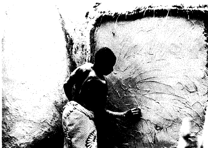
Fig. 27: After the plaster has been applied another woman smoothens the surface with a flat stone.
