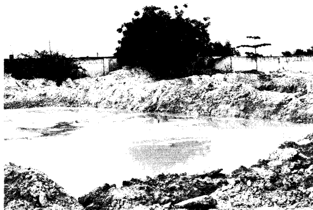
Fig. 207: Lime sludge waste at the AIR LIQUID factory in Tema, 1981.
