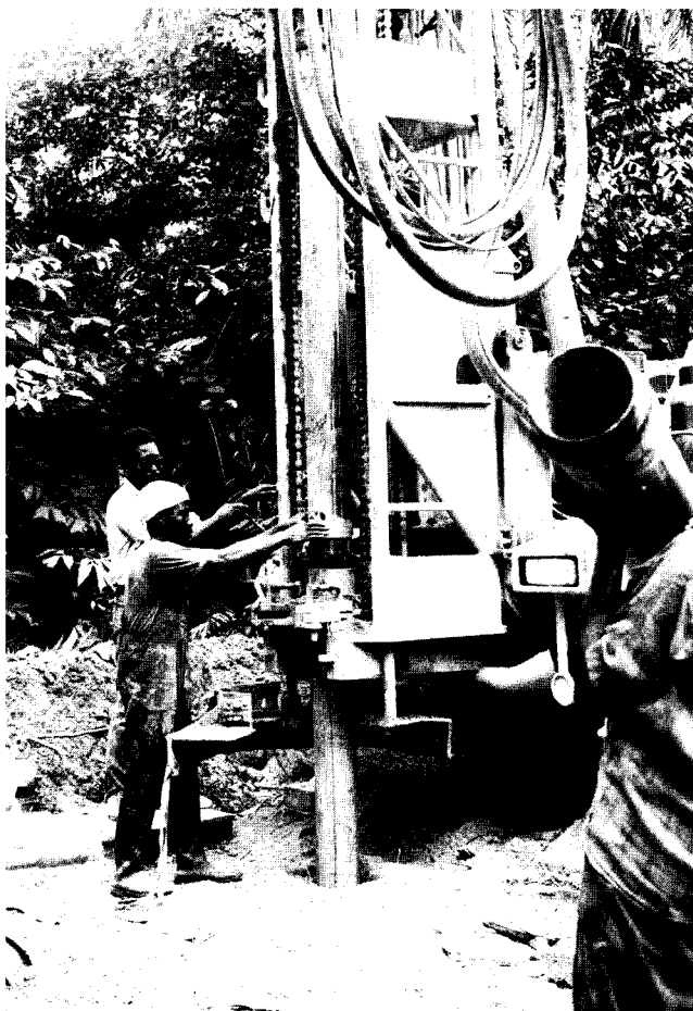
Fig. 377: Well drilling in the Volta Region, 1982. (Prakla Seismos Well Drilling Project).
