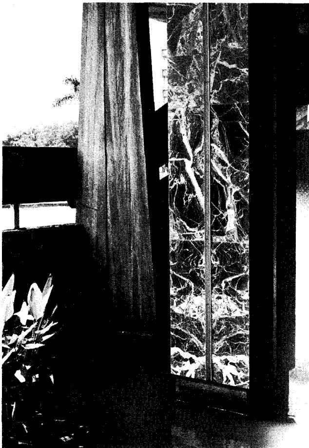
Fig. 301: Polished stone cladding (containing Jasper, Volta Region) on the Volta River Authority Building, Accra, 1982. Architect: KENNETH SCOTT.
