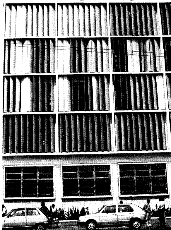
For Fig. 331: South elevation of Barclays Bank, High Street, Accra, 1982. Architects: HARRISON, BARNES & HUBBARD.
