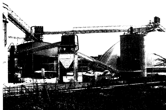
Fig. 179: Part of the Cement Works in Tema, 1981.
