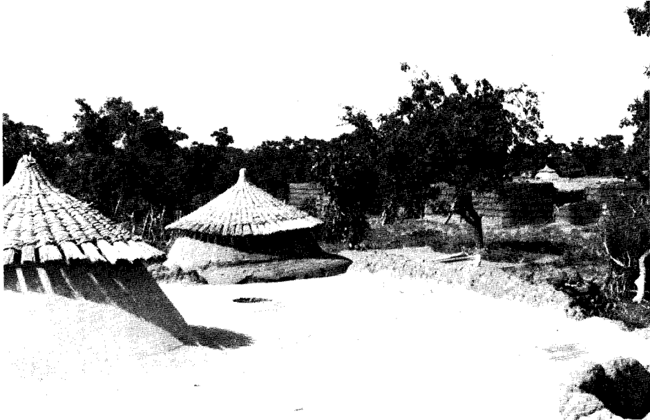
Fig. 45: Roof of the same compound. Note the grain silos protruding through the flat mud roof, and the low parapet around the roof.
