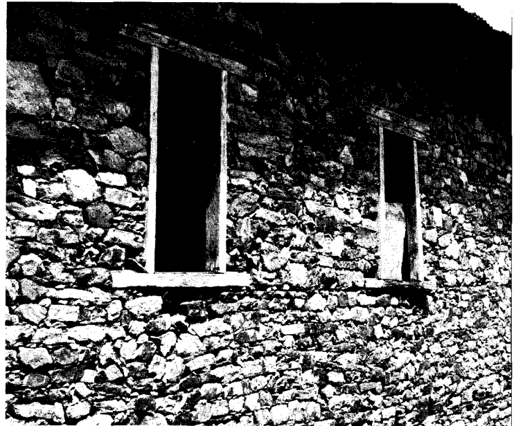
Fig. 113: A newly constructed stone house in Akropong, Akwapim, 1981 (Photograph by G. OWUSU).
