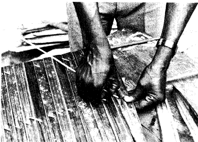
Fig. 154: ...fixing them around two split pieces of bamboo;
