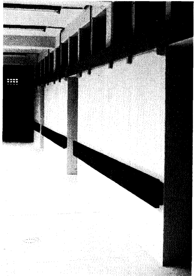
Fig. 412: Trunking fixed above door level with conduits on wall surfaces leading to light switches and high fittings. Lomé Hospital, Togo; Architect: G. LIPPSMEIER.
