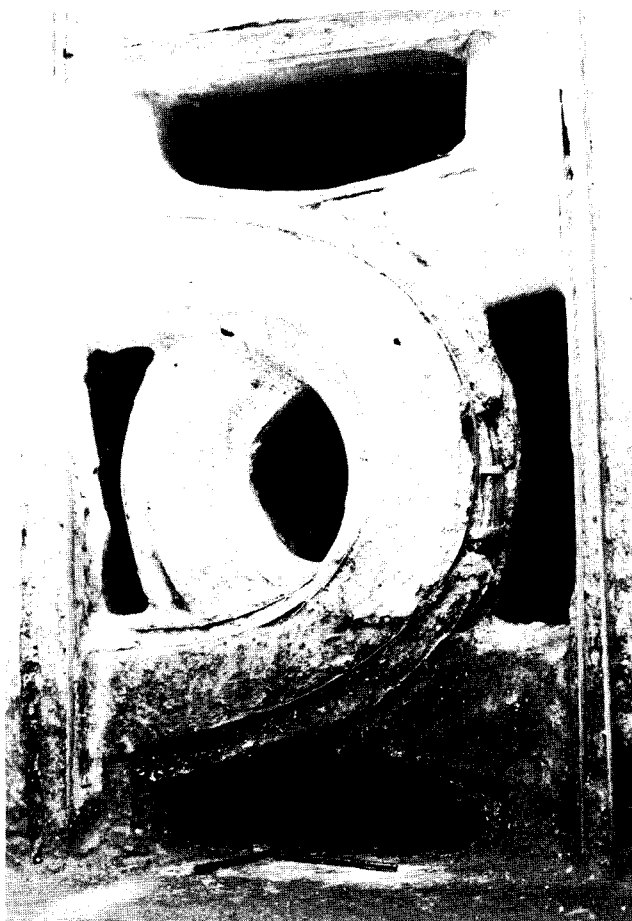
Fig. 85: Detail of screen wall showing part of the core.
