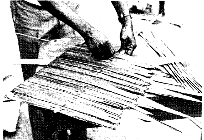
Fig. 155: ...tying the leaves together with small bamboo splits.
