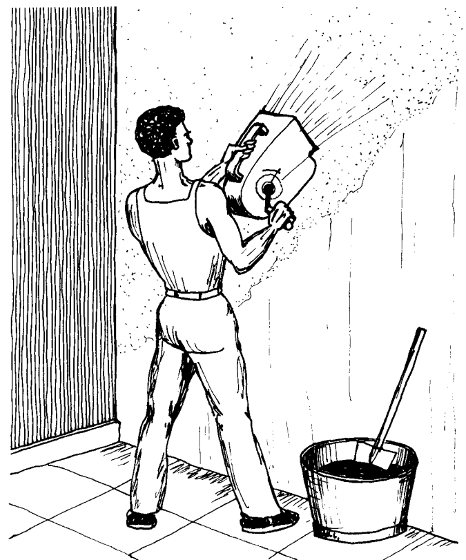
FIG. 293 : APPLICATION OF 'TYROLEAN' FINISH .
