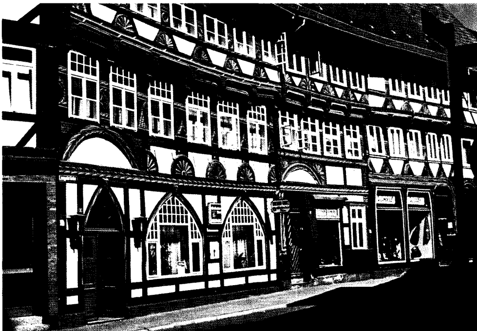
Fig. 233: 16th Century square panelled timber framework in Einbeck, Lower Saxony, West Germany, 1978.
