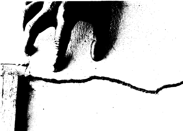
Fig. 217: Runways of subterranean ants on a house wall in Kumasi.
