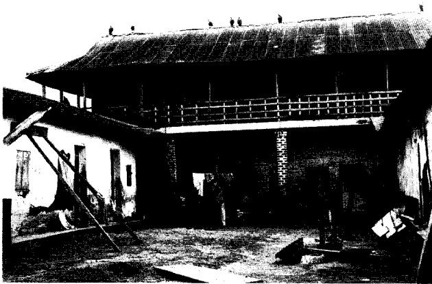
Fig. 120 and 121: A brick-core house with cantilevered first floor verandah in Konongo, Ashanti Region, 1981.
