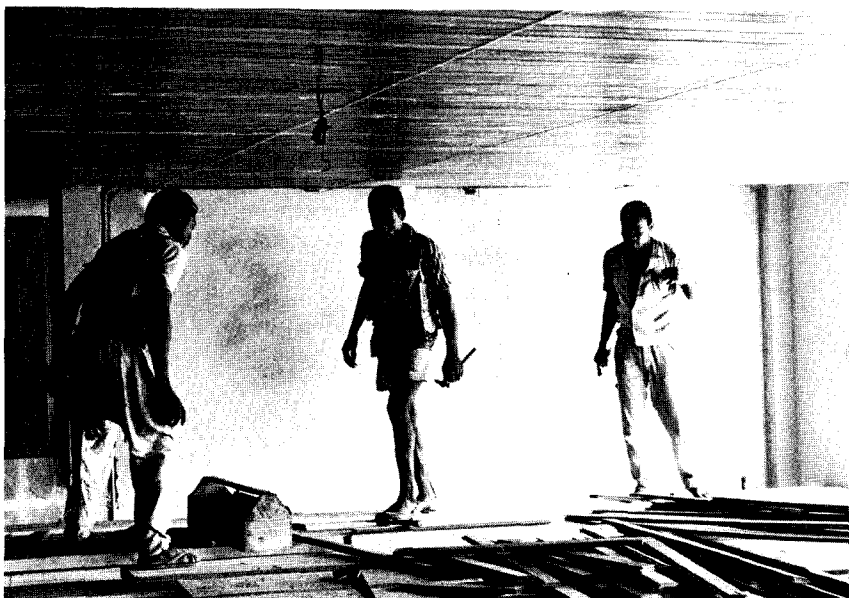
For Fig. 350: Fixing of a suspended hardwood strip ceiling in the entrance hall of Parliament House, Accra, 1970.
