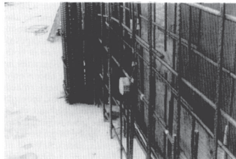
(b) Photograph of fiber installed in the rebar grid.
