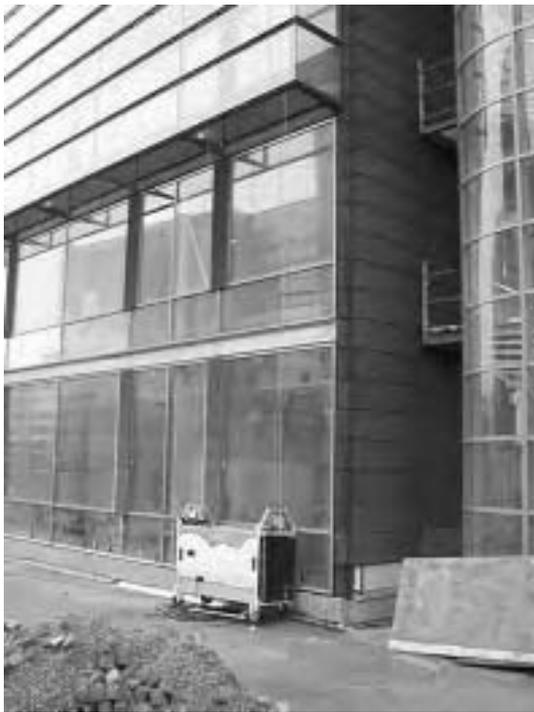
Figure 10: The service cage for the maintenance of the intermediate space.
