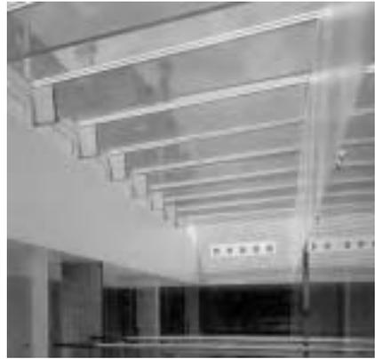
Figure 1: An example of structural glass : tempered beams supporting a glass roof in the Louvre museum
