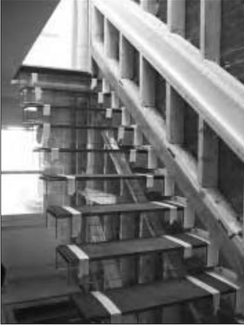
Figure 2: Global structural system of glass stair (during construction)
