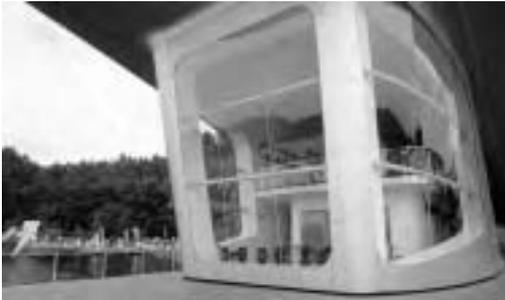
Figure 6: Cold deformed laminated glass panels
