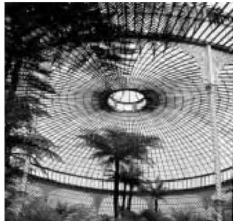
Figure 1: Kibbles Palace in Glasgow (1873). Note the slight out-of-plane curvature of the vertical iron arches on the right photo. This indicates the bracing action of the glass panels.
