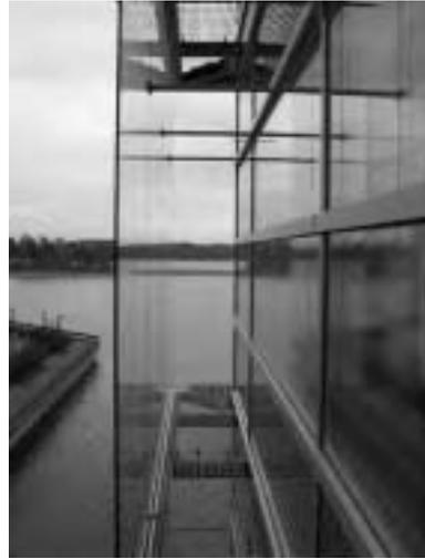
Figure 1: Cantilever beams as a supporting structure
