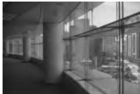
Figure 5: Horizontal glass beams span 12m
