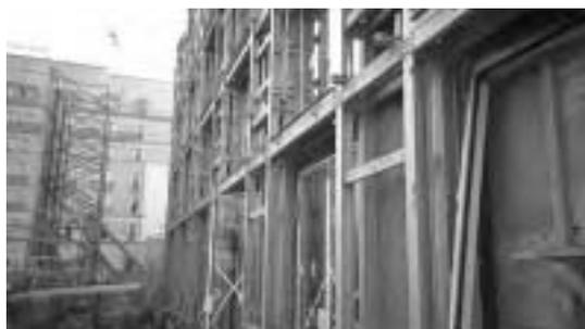
Figure 5: Steel-girder construction of the façade
