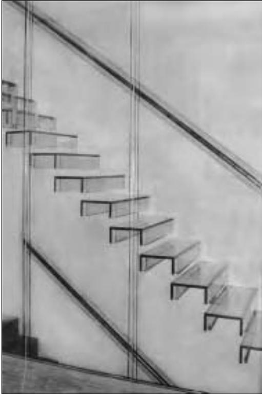
Figure 12: Finished glass tread and balustrade (not touching the treads)
