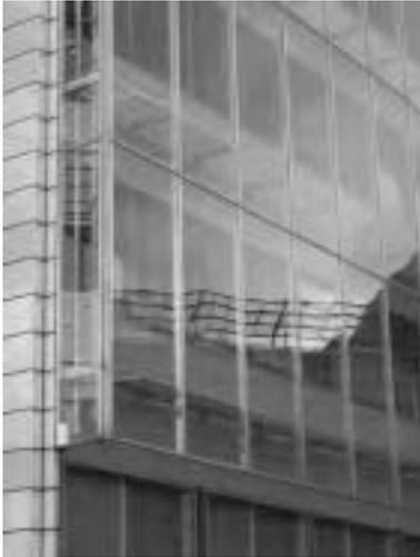
Figure 3: Vertical frames as a supporting structure
