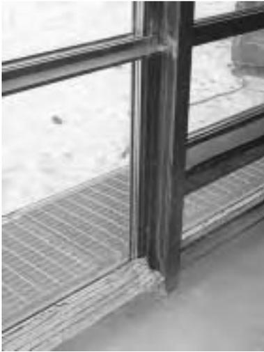
Figure 8: Double-skin structure connected to an I-section column
