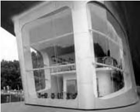
Figure 20: Cold bent glass laminated panels in the Floriade building in the Haarlemmermeer
