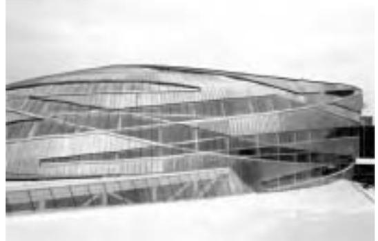
Figure 9: The so-called ‘spaghetti-strips’ of cold formed glass panels
