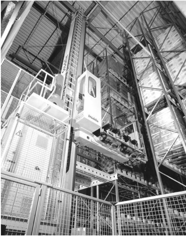
Figure 4.23. Rack feeder for pallet handling [Photo: STÖCKLIN SIEMAG]
