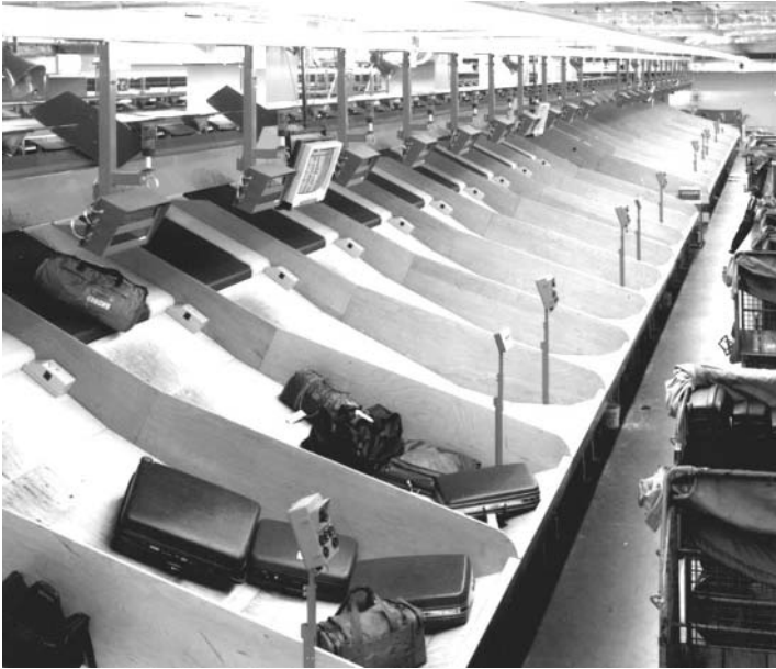
Figure 4.27. Terminals: chutes [Photo: BEUMER]
