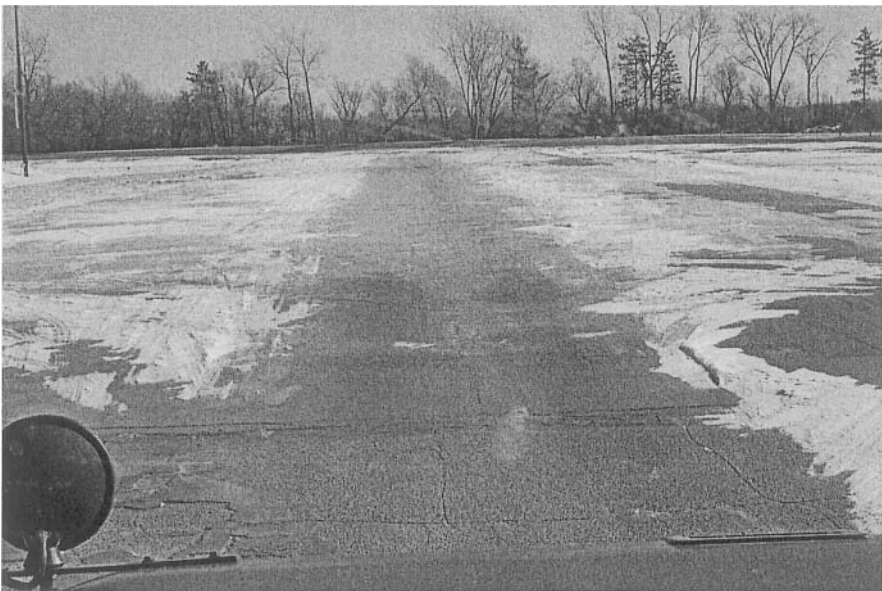
Figure 14-11. The track used to conduct the experiments for this section
