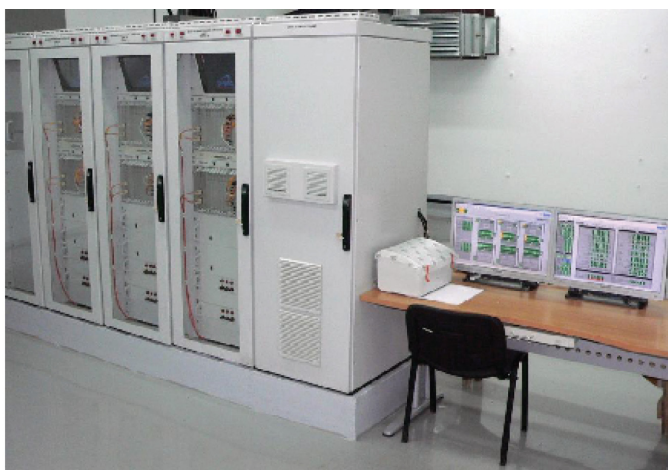
Figure 7. Reactor power control and limitation system
