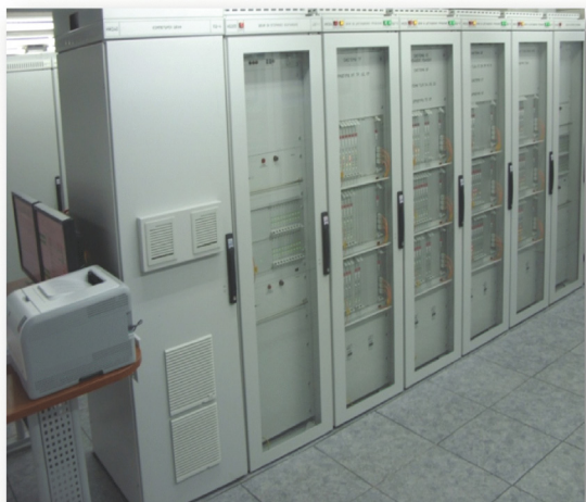
Figure 5. Part of software-hardware complex of engineered safety features actuation system on the base of RADIY PLATFORM
