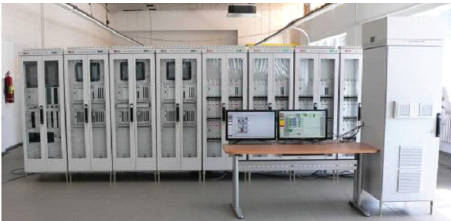
Figure 8. Rod control system
