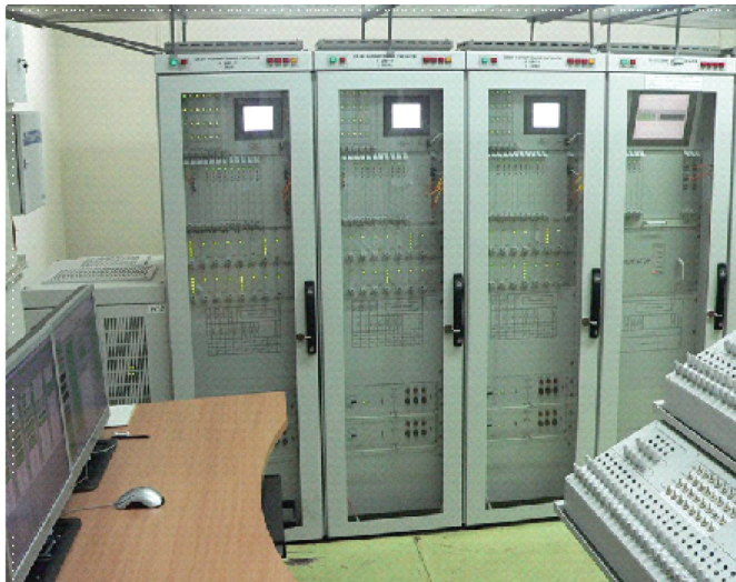
Figure 7. Reactor power control and limitation system
