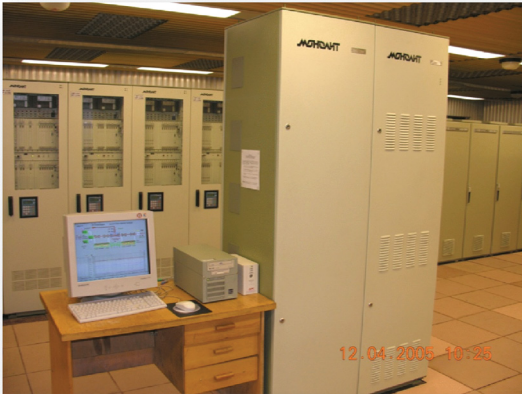
Figure 6. Software-hardware complex of turbine control system
