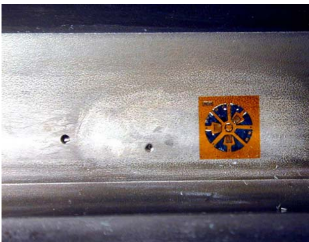
Fig. 14 Gauge and drilled holes at the OD
