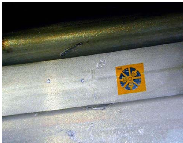
Fig. 15 Gauge and drilled holes at the ID
